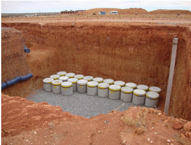
Figure 9.1 Disposal of low and intermediate level radioactive wastes at Vaalputs, South Africa. Reproduced with permission from M. Ojovan
