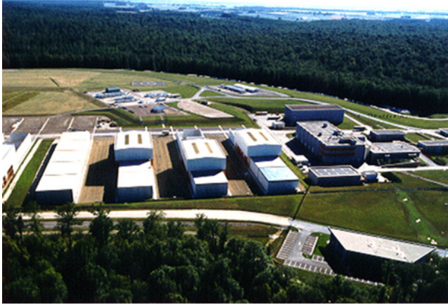
Figure 9.3 Steel movable shelter for Centre de l'Aube (Potier and Gallagher, 1998). Reproduced with permission from J.-M. Potier. © 1998
