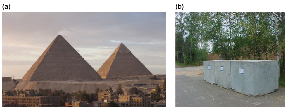
Figure 10.2 (a) Egyptian pyramids. Reproduced with permission from P. Yakovlev. According to Davidovits' theory, they have been cast on site and are composed of blocks made of geopolymers. (b) Concrete containers. The long-term durability of cementitious materials is crucial to ensure safe immobilization of nuclear waste. Reproduced with permission from M. Ojovan
