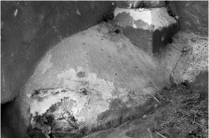
Figure 2.3.14. Detail of the left most, dual ovoid symmetric structures flanking the rectangular discharge opening within the internal water tank at the north end of the theatre.
