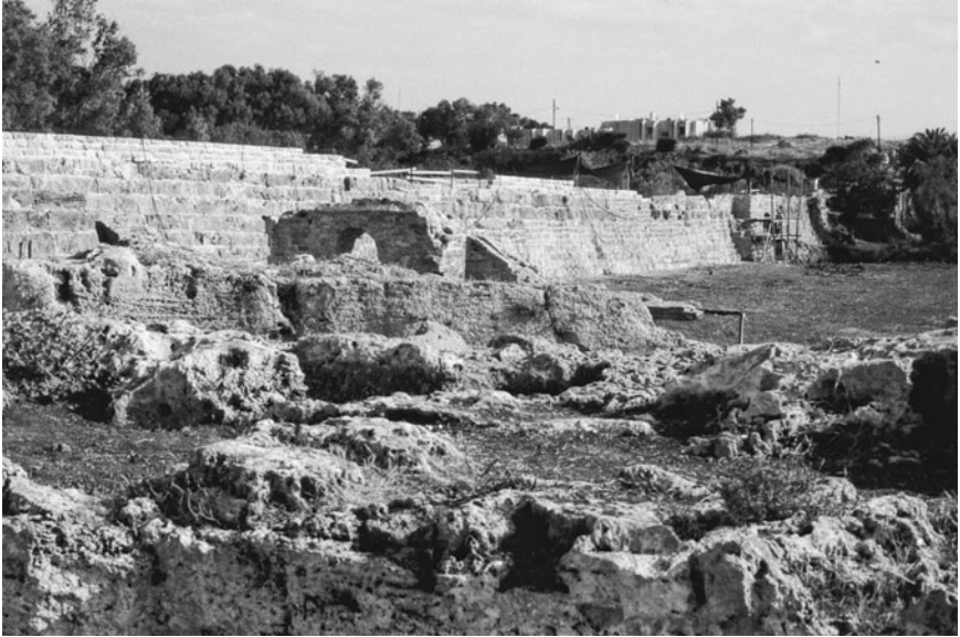
Figure 2.5.2. The dam front wall of the reservoir supplying water to Caesarea with ~8 m height.
