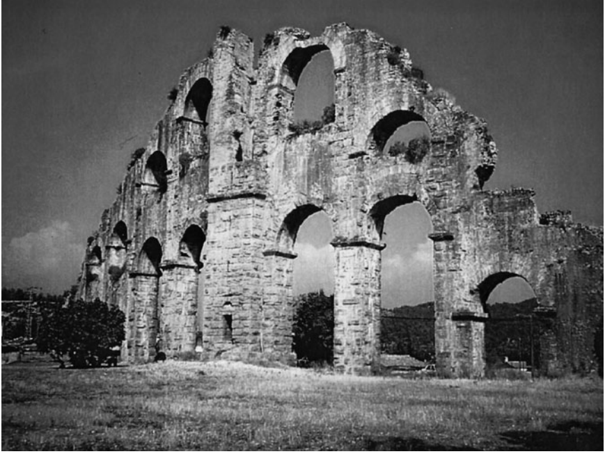
Figure 2.2.3. One of the two towers supporting open tanks of the Aspendos Siphon.
