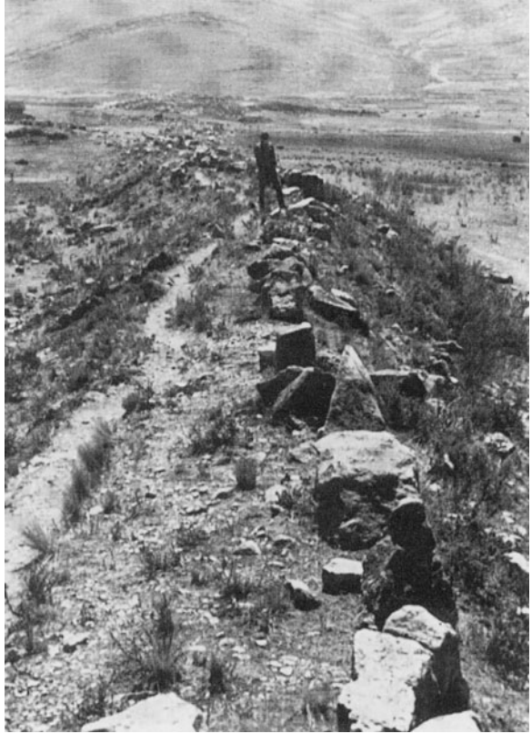
Figure 1.2.9. The Pajchiri aqueduct.
