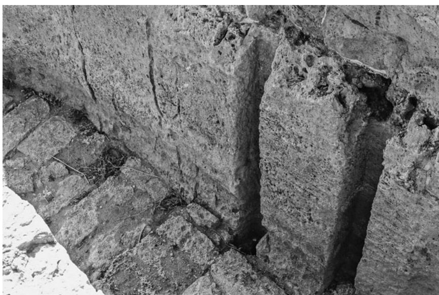
Figure 2.5.4. Detail of the symmetric vertical groove structure carved into the walls in the exit region of the dam. Wall height in this area is c. 5 m.
