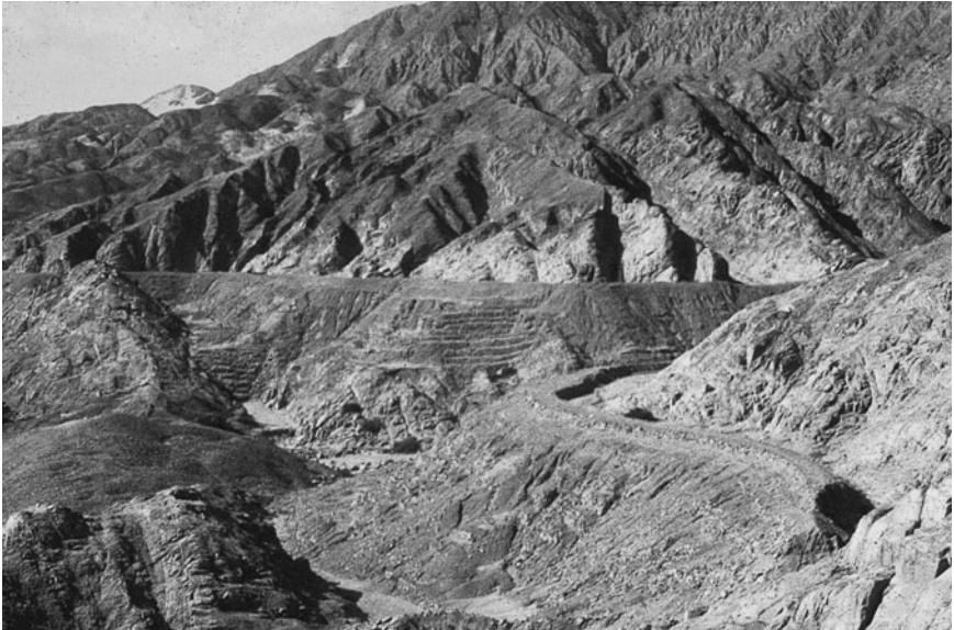
Figure 1.1.16. The Intervalley Canal at point M (Figure 1.1.6) north of Quebrada del Oso. The canal is built on 20 m high fill terraces on mountain slopes for much of its length.
