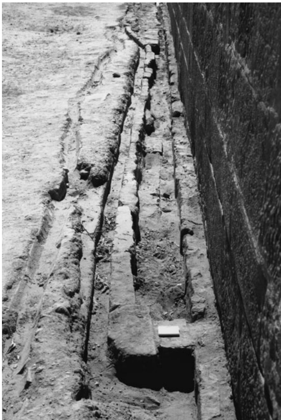
Figure 2.1.9. Part of the drainage channel collecting seepage water from the back wall of the Great Temple. Water led to an underground reservoir in the eastern part of the temple.
