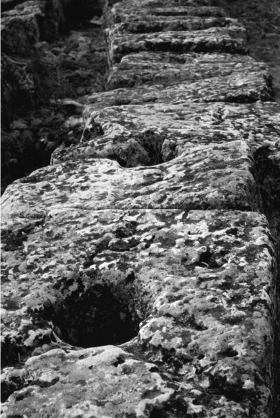
Figure 2.3.7. Top holes in the Laeodocian piping system. The top holes let air into the piping to alleviate partial vacuum regions that result from the contracted water (normal) depth in the steep downhill piping supporting supercritical flow.
