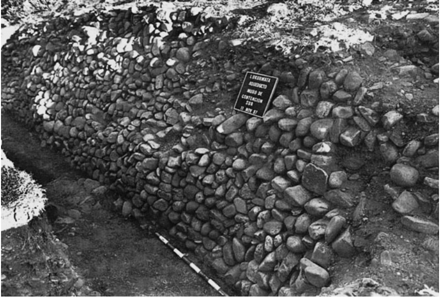
Figure 1.2.3. Stone lined side wall of the Lukurmata aqueduct. The aqueduct directs rainfall runoff from adjacent hill slopes into the centre section of the aqueduct between stone outer walls.
