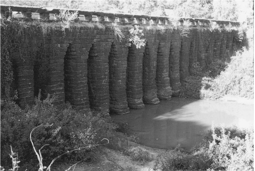
Figure 3.1.7. Khmer bridge of 15 m height built with corbelled arch construction and still in use in modern times.
