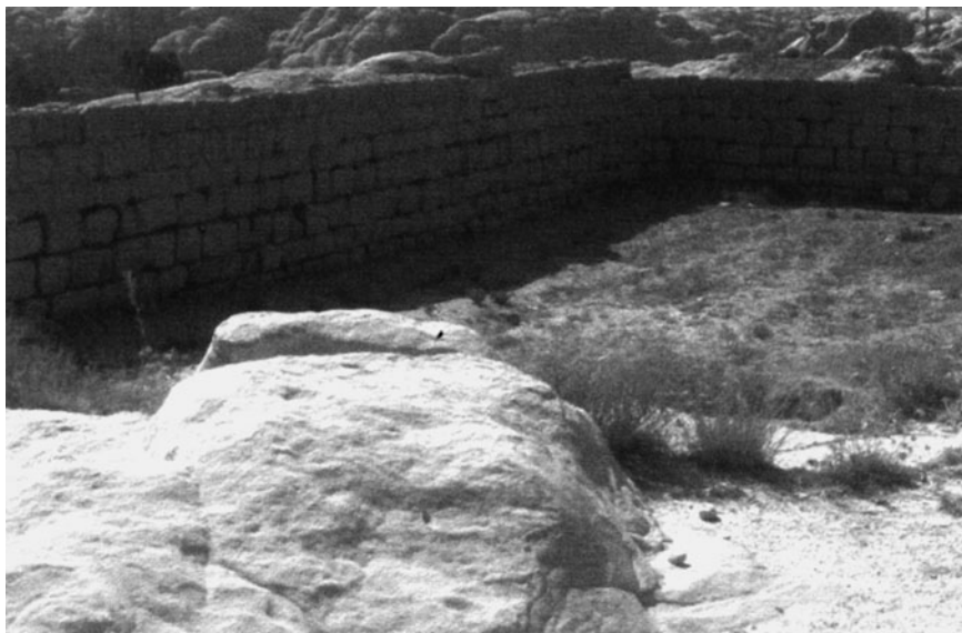
Figure 2.1.4. The Zurraba (al Birka) reservoir made from clay bricks; the current height of the enclosing wall is 2 to 3 m.
