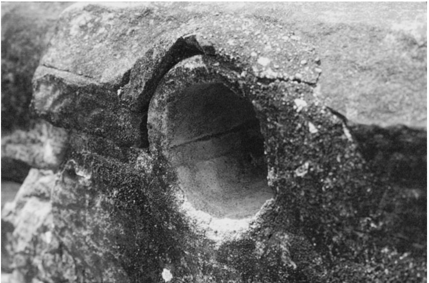
Figure 3.1.5. Piping detail between the central basin and an adjacent basin. The laterite piping is carefully inserted into the surrounding block structure with sealant to eliminate leakage.
