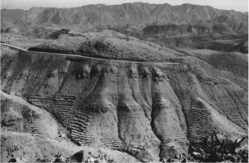
Figure 1.4.2. Canal with drop off outlets on alternate sides of a mountain ridge to supply terraces on each mountain face typical of Wari terrace canal construction techniques in mountainous terrain.
