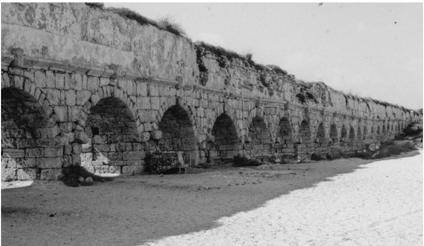
Figure 2.5.1. The Roman aqueduct at Caesarea in northern Israel.
