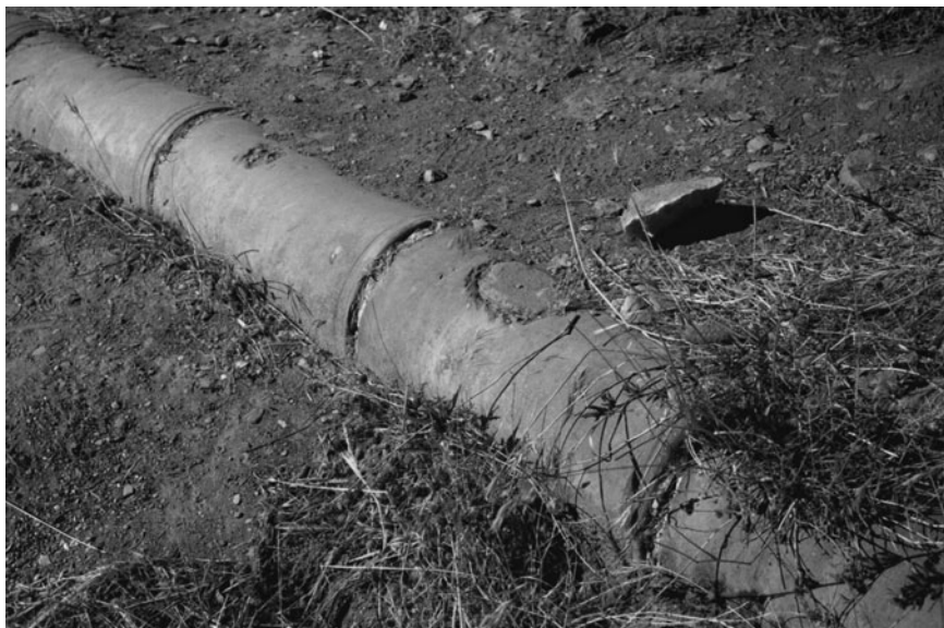
Figure 2.3.5. Roman construction piping elements leading from the Castellum. Top holes, some plugged and some open, are indicative of partial flow conditions within the piping.
