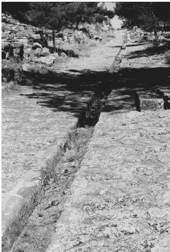
Figure 2.4.2. The West Gate (Figure 2.4.1) drainage channel running downhill in the east west direction interior to Priene.
