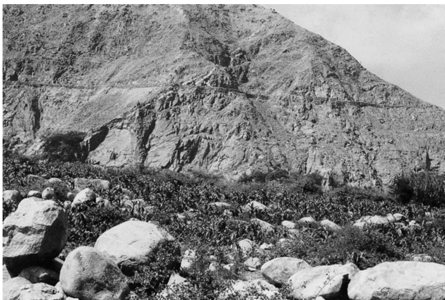
Figure 1.1.11. Highest elevation canal (Huatape S3, Figure 1.1.4) on the southern face of Cerro Orejas in the Moche Valley designed to provide water to upvalley farming areas.
