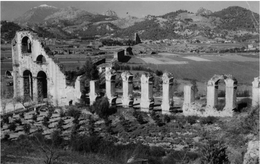
Figure 2.2.2. Field view of the Aspendos Siphon with the South Tower in the foreground.
