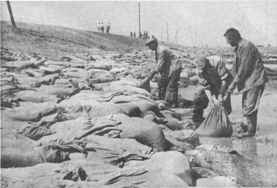
Fig. 3.24. Slope and toe loaded by bags filled in with sand.
