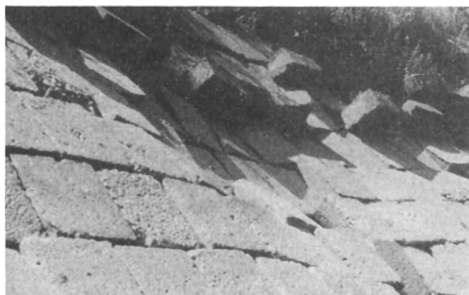
Fig. 3.17. Floor deformation.
