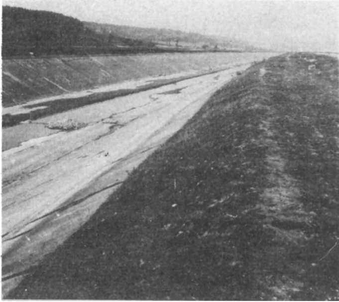
Fig. 2.61. Canal in empty conditions.
