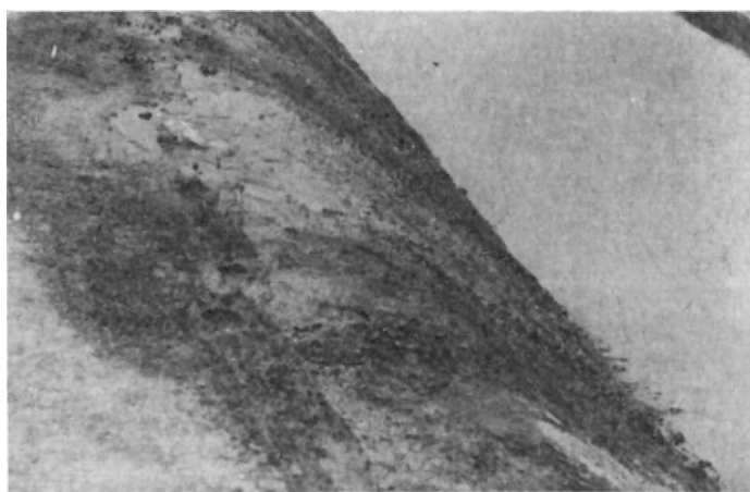
Fig. 2.60. Water boils caused by groundwater pressure.
