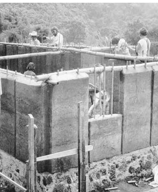
7-17: A low-cost bamboo-reinforced earth house project in Guatemala.
