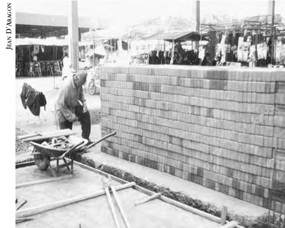
5-13: In order to encourage a market for compressed earth blocks, Jean D'Aragon, built a prototype building of the new material in downtown Santo Antonio, with the help of a local mason.
