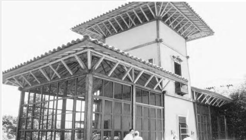
7-10: A two-story bamboo structure by Marcelo Villegas.
