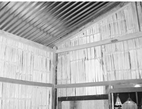
7-9: An interior view of one of the houses by Hogar de Cristo, showing the lightweight frame, bamboo exterior panels, and metal roof.
