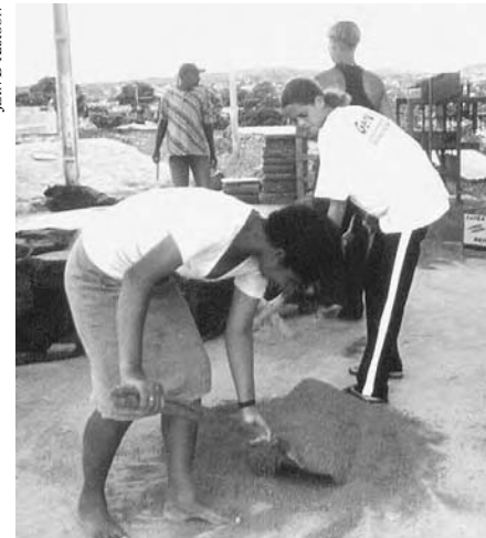
5-11: Students mix clay, sand, and water in proper proportions to make compressed earth blocks.
