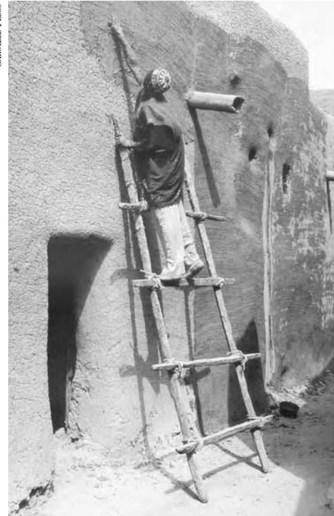
2-1: In Djenne, Mali a plasterer works without a trowel. Adobe walls are replastered, as needed, after one or several rainy seasons.
