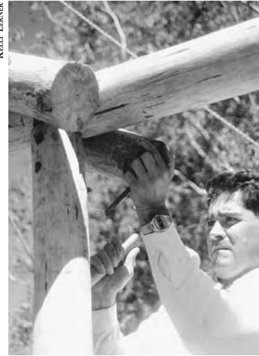
7-20: Small-diameter wood poles create the structure for a straw bale house in Argentina.
