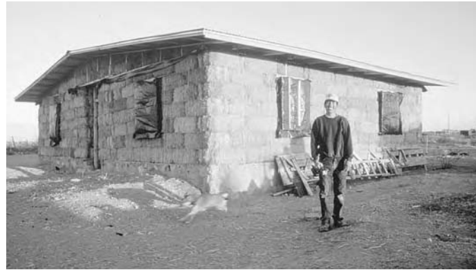
1-11: Jose Luis Rocha stands proudly in front of his house built (with the help of Builders Without Borders members) of locally available materials such as straw, recycled concrete, and wooden pallets.
