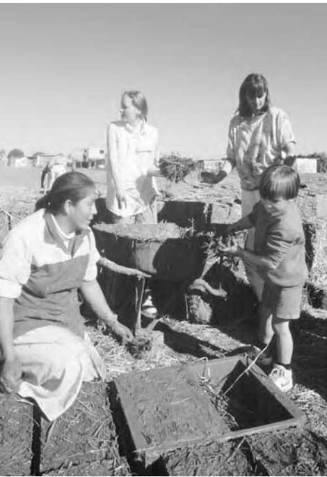
3-1: Mexican women and children engaged in producing straw-clay blocks, a sustainable building material using local resources.
