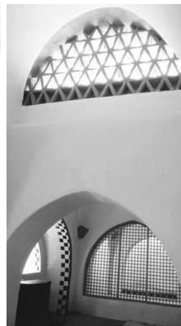
2-11: An interior view of Hassan Fathy's only US project, the Dar al Islam mosque near Abiquiu, New Mexico showing vaulted ceiling and claustra ventilation system.
