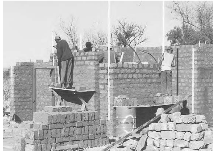
1-8: The local clay earth is used at Tlholego to create modern looking, comfortable, and inexpensive dwellings.
