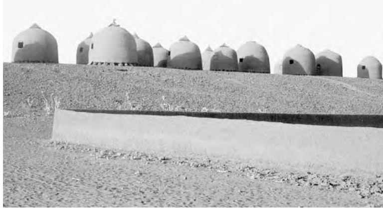
2-3: Granaries in Affala, Niger are built in coils, an application of a pottery-making technique on a larger scale.
