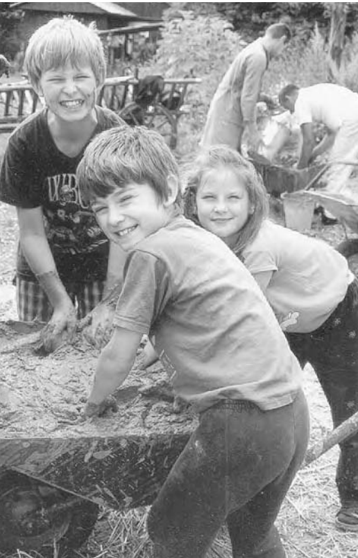
7-15: Children mixing earth plaster for use on a straw bale house.
