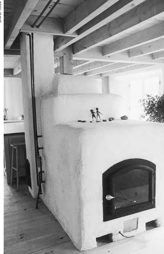
3-2: This high-mass masonry stove at the Earth Sweet Home Institute is an example of a highly efficient heating technology designed to minimize the use of wood and reduce pollution.
