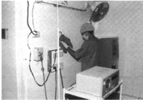
Fig. 6.2: Cleaning of the operation theatre walls with Bacillocid
