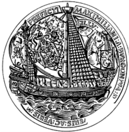
FIG. 4. Three-masted ship of carvel construction with living quarters in the fore- and aft-castles and with gun ports. Seal of Maximilian, prefect of Burgundia, 1493.
