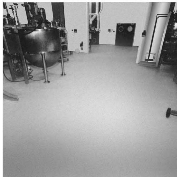
Figure 1 Polyurethane-modified concrete laid by Swansback. Photographic Unit of the Boots Company plc.
