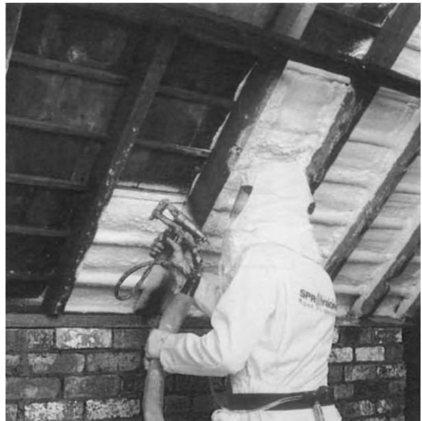
Figure 3 Stabilizing polyurethane Spraybond foam being applied. Courtesy of Liquid Polymers plc.
