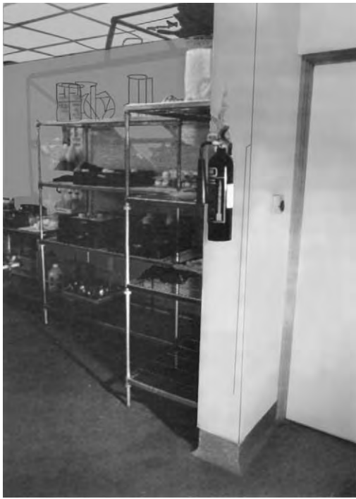
Figure 2 A polyurethane-based wall finish by Sempol Surfaces Ltd in association with an epoxy seamless floor in a food factory.
