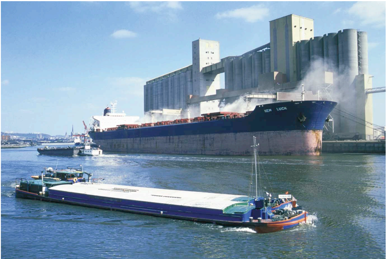
Plate 24 Cereals Harbor elevator in Rouen, France, with a total storage capacity of 300 000 tonnes. This is able to load grains into vessels at a rate of 5000 tonnes h -1 . Photo courtesy of J. Pfeiffer.
