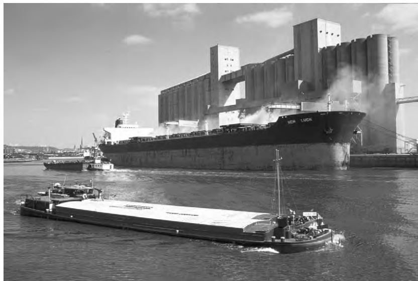
Figure 2 (see color plate 24) Harbor elevator in Rouen, France, with a total storage capacity of 300 000 tonnes. This is able to load grains into vessels at a rate of 5000 tonnes \text{h}^{-1} . Photo courtesy of J. Pfeiffer.
