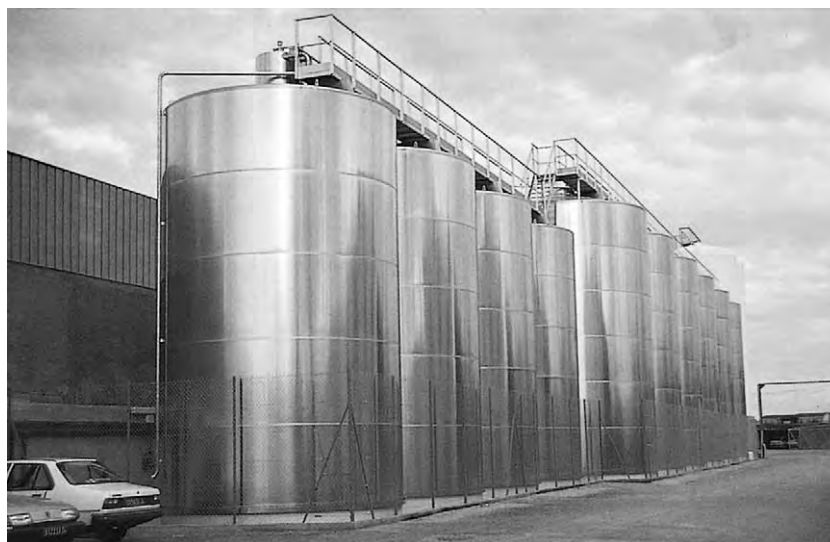
Figure 2 A battery of wine storage tanks made from chromium nickel molybdenum stainless steel. Addition of molybdenum allows the tanks to be used for white as well as red wine. (Courtesy of UGINE S.A., France.)
