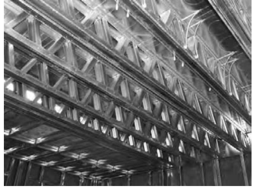
Figure 4.21 Steel frame, Stoneguard house
