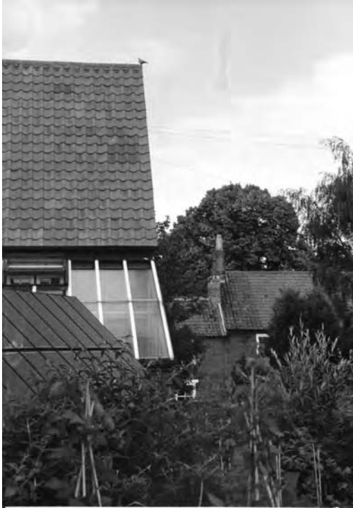
Figure 4.3 The 'Autonomous House' Southwell, rear view with 2.2kW photovoltaic cell array
