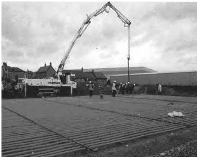
Figure 11.7 Pipe network beneath the school playground
