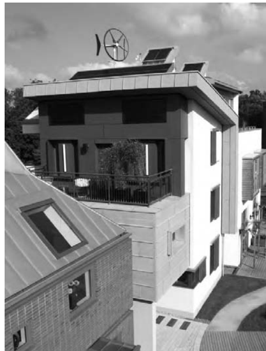
Figure 4.16 Zero Carbon house by Barratt Homes and Architects Gaunt Francis
