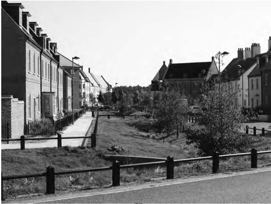
Figure 5.3 Storm ditch between rows of houses, Upton, Northampton, UK
