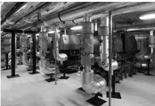
Figure 11.3 Ground source heat pumps plant room, Churchill Hospital, Oxford
