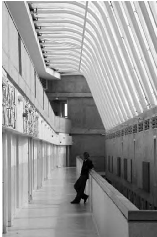
Figure 11.4 St Francis of Assisi school: interior with translucent ethylene tetrafluoroethylene roof
