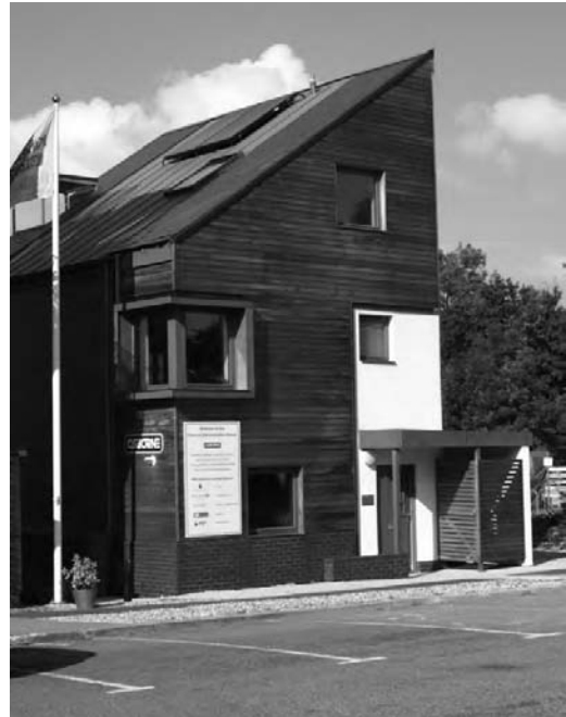
Figure 4.12 Osborne House at BRE with lightweight construction and low thermal mass
