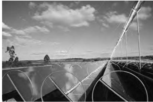
Figure 14.10 Fresnel solar thermal electricity, southern Spain
