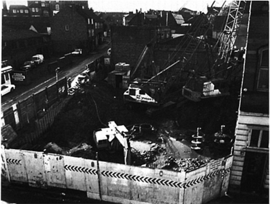
Figure 13.6 Development under construction at Micklegate, York. (Source: York Archaeological Trust.)
