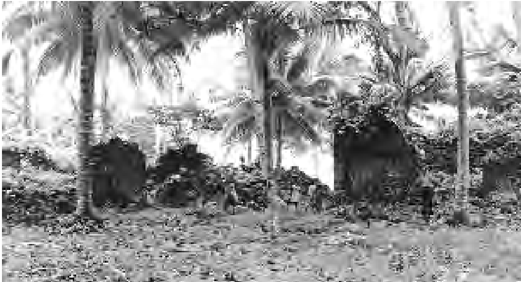
Figure 4.2 Site 1 — Kota Lama Wokam: Dutch Fort, view of rampart looking southwest
