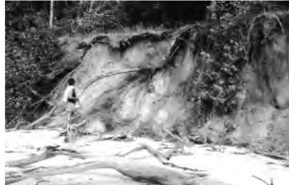
Figure 4.20 Site 17 — Jambu Air Lama: close-up of eroding section of site
