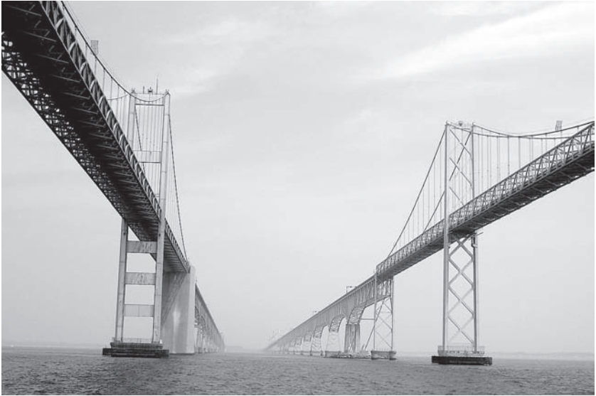
Figure 3. Twin spans of the Bay Bridge over the Chesapeake Bay in Maryland.
