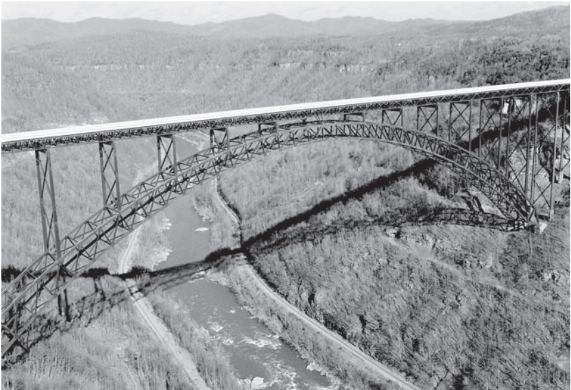
Figure 2. New River Gorge Bridge in Fayetteville, West Virginia.
