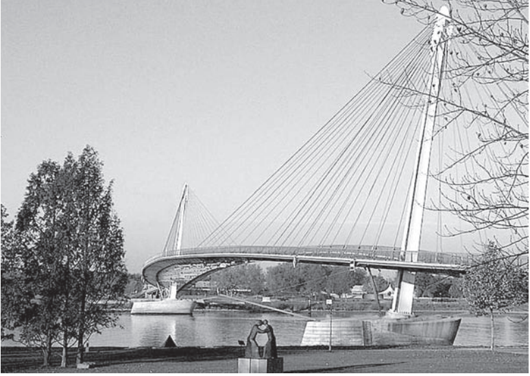
Figure 1. The Passerelle du Jardin des Deux Rives is a bicycle and pedestrian bridge between Kehl in Germany and Strasbourg in France.
