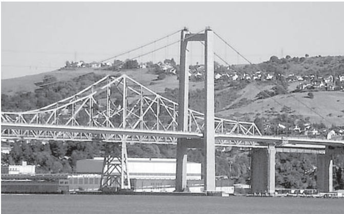
Figure 5. The newest Carquinez Strait Bridge, a suspension bridge, was completed in 2003, adjacent to the second Carquinez Strait Bridge, which was finished in 1958.
