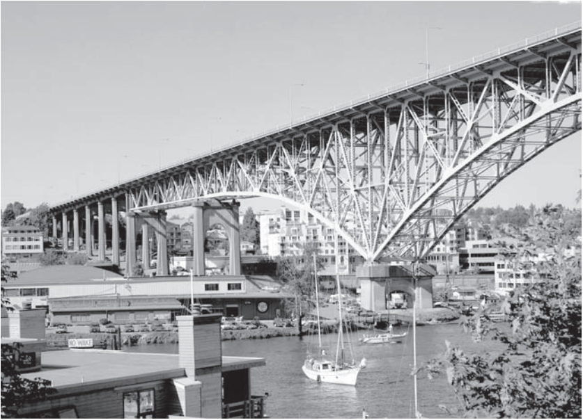
Figure 3. Aurora Bridge, Seattle.
