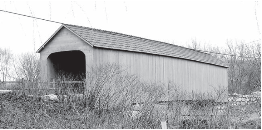
Figure 1. Upper Sheffield Bridge crossing the Housatonic River in Sheffield, Massachusetts.
