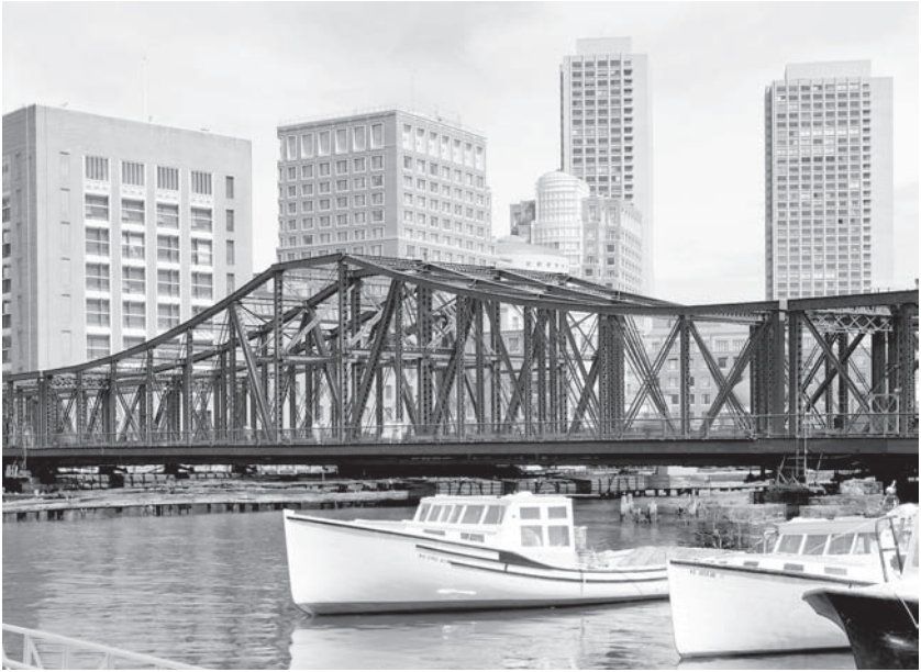
Figure 1. Northern Avenue Bridge in Boston.
