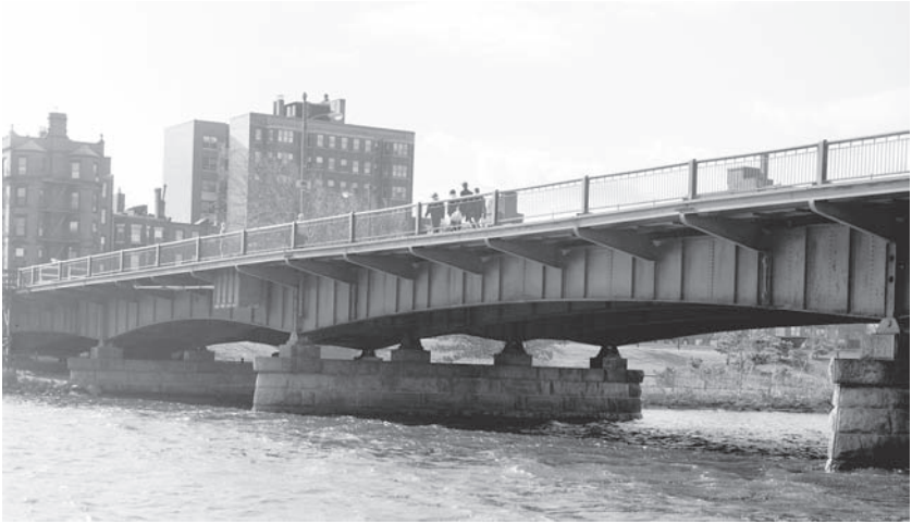
Figure 1. Harvard Bridge crossing the Charles River in Boston.
