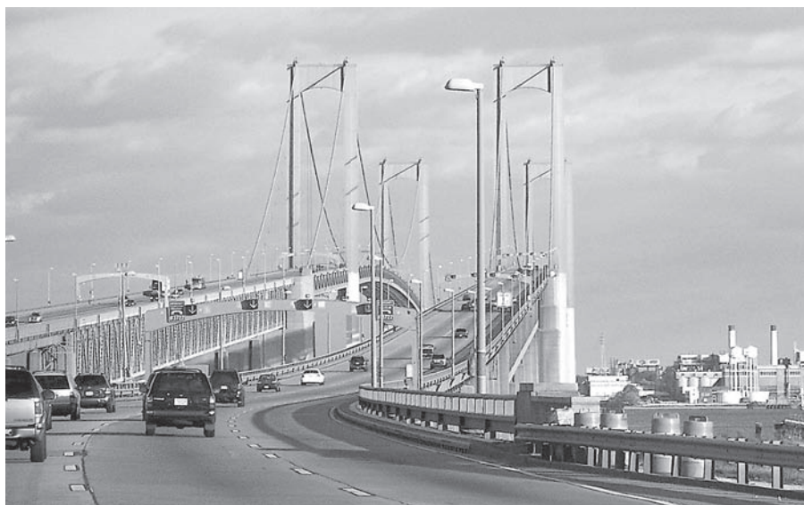
Figure 4. Twin spans of the Delaware Memorial Bridge were built 17 years apart.
