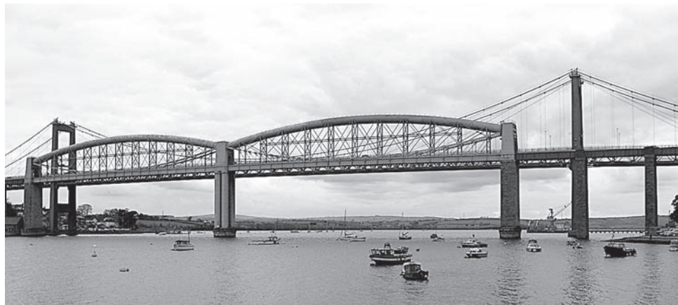
Figure 3. In the United Kingdom, the Tamar Road Bridge, a suspension bridge, was paired unfortunately with the Royal Albert Bridge, a lenticular truss railroad bridge designed by I. K. Brunel.
