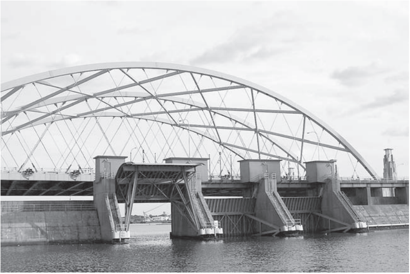
Figure 1. Providence River Bridge, a new tied-arch bridge in Providence, Rhode Island. Note the hurricane barriers.
