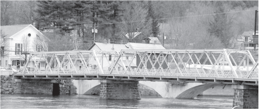
Figure 3. Shelburne Falls Truss Bridge.
