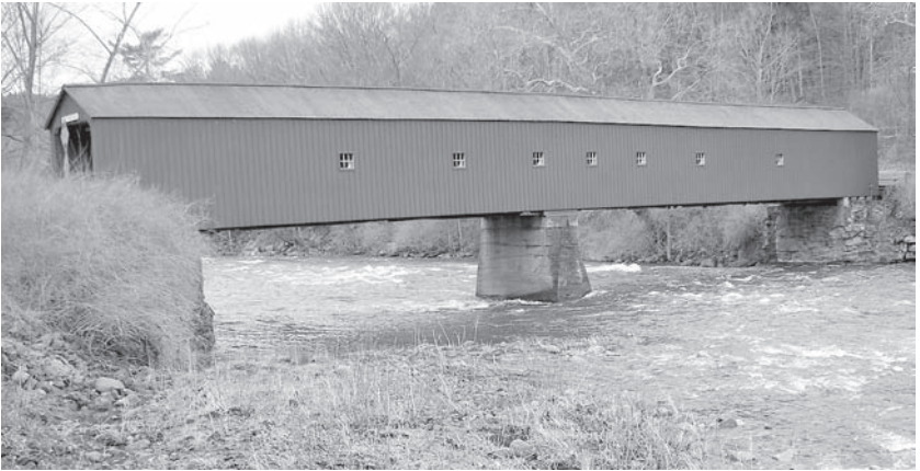
Figure 2. Covered bridge in West Cornwall, Connecticut.
