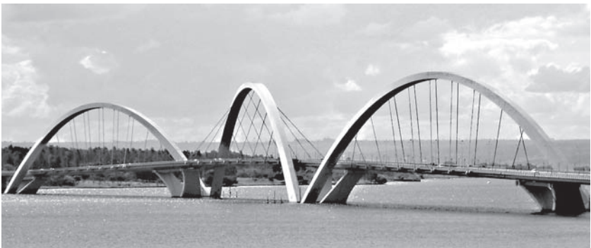
Figure 3. JK Bridge over Lake Paranoá, Brasília, Brazil
