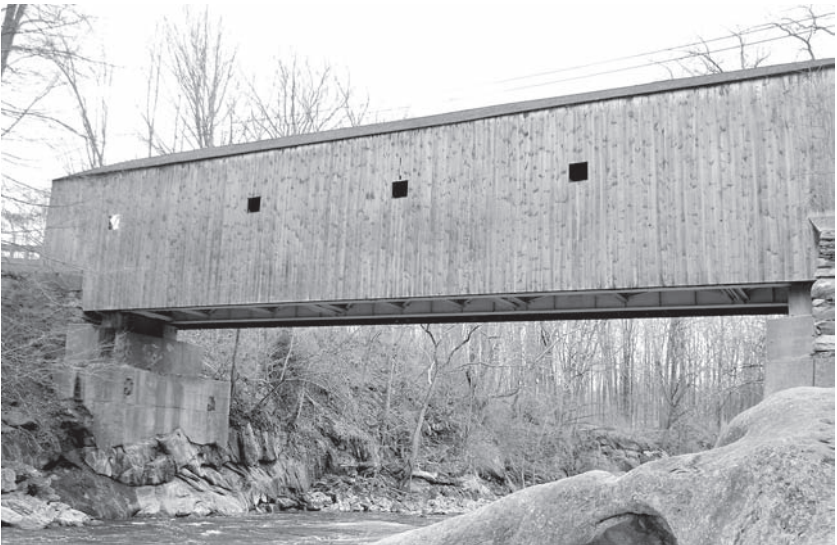
Figure 3. Bull's Bridge in Kent, Connecticut.
