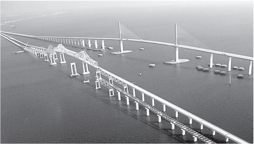
Figure 2. The Sunshine Skyway Bridge crosses Tampa Bay in Florida. The original bridge (left) is being dismantled; the new cable-stayed bridge (right) carries traffic.
