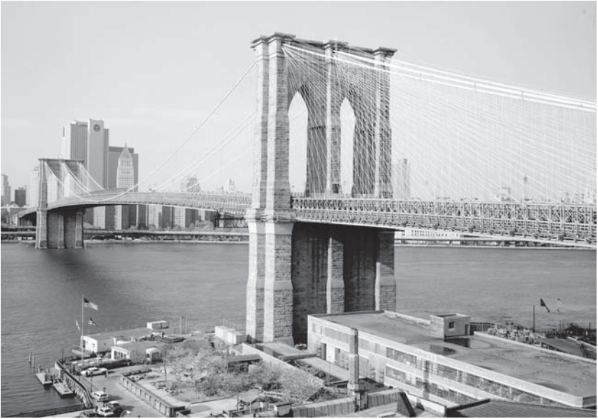
Figure 1. Brooklyn Bridge, with the Brooklyn ferry slip in the foreground.
