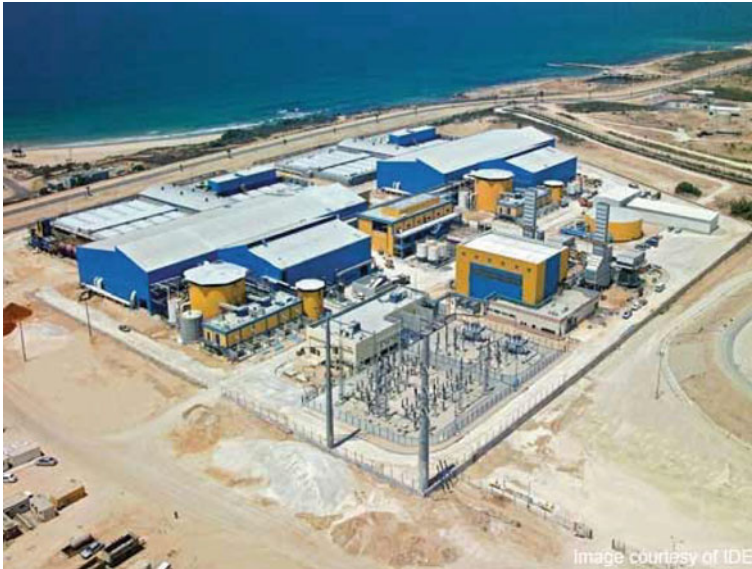
Fig. 2 Ashkelon seawater reverse osmosis desalination plant, Israel. As of circa 2006 it was manufacturing 50,000,000 m 3 yearly. Ultimately, it will manufacture 100,000,000 m 3 annually
