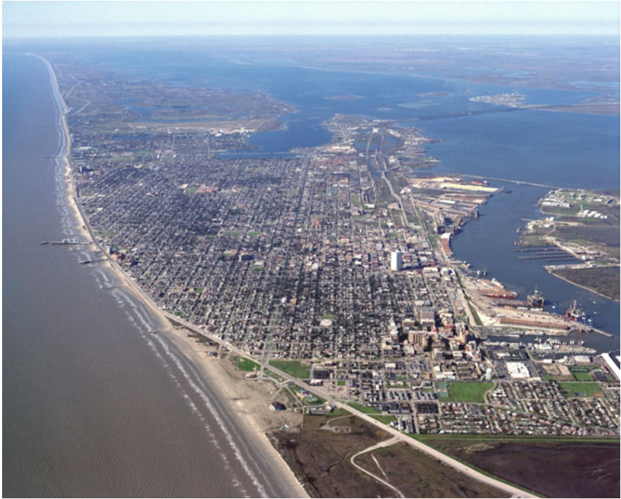
Fig. 10 City of Galveston Aerial showing the modern Galveston Seawall. Reproduced by permission of Robert Mihovil, copyright 2010
