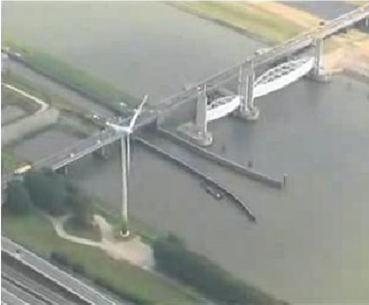
Fig. 7 The Hartelkering is a large lift gate that allows passages 98 m (322 ft) and 49.3 m (161 ft) wide with 14 m (46 ft) clearance
