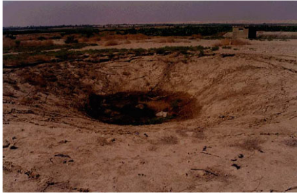
Fig. 12 Sinkhole along the eastern coast of the Dead Sea (taken by Sawariah, Natural Resource Authority, Jordan)
