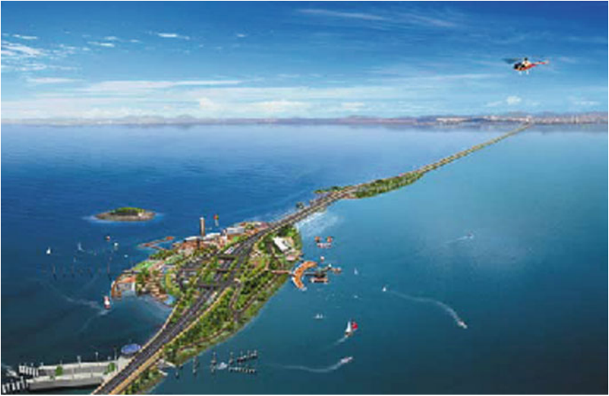
Fig. 14 View of Lake Shiwa tidal power plant (Korea) that was projected to be completed by the end of 2009, but still is being worked on according to information available in early 2010
