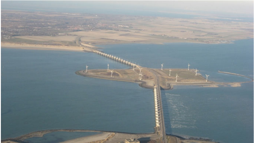
Fig. 8 Two of the three sections of the Oosterscheldekering, a surge barrier which allows tidal flows and water exchange between the Eastern Scheldt estuary and the North Sea. The total length of floodgates is 4 km (2.5 miles) composed of 62 individual steel doors each 42 m (138 ft) wide
