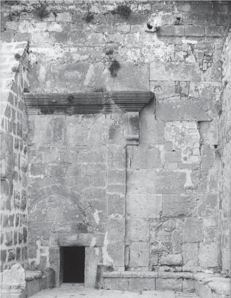
▲ Bethlehem. Main Door of the Nativity. The battered facade bears mute witness to the turbulent history of the edifice. The projecting flat lintel is that of the C6 entrance. The blocked arch door is medieval, and the present entrance is Mamluk or Ottoman.
