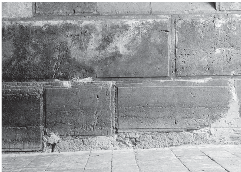
▲ Western Wall. The magnificent masonry of Herod's temple is illustrated by typical blocks (flat boss, wider upper margin) from its sister building, the Tomb of the Patriarchs in Hebron.
