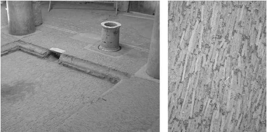
FIGURE 9.3. Impluvium surfaced with recycled amphora sherds set on edge at Casa dei Ceii at Pompeii. Left: general view. Right: detail. Photos: JTP.
