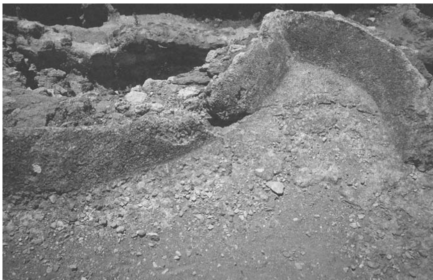
FIGURE 9.4. Decomposing cocciopesto lining in basin at Campetti site at Veii. Photo: JTP.
