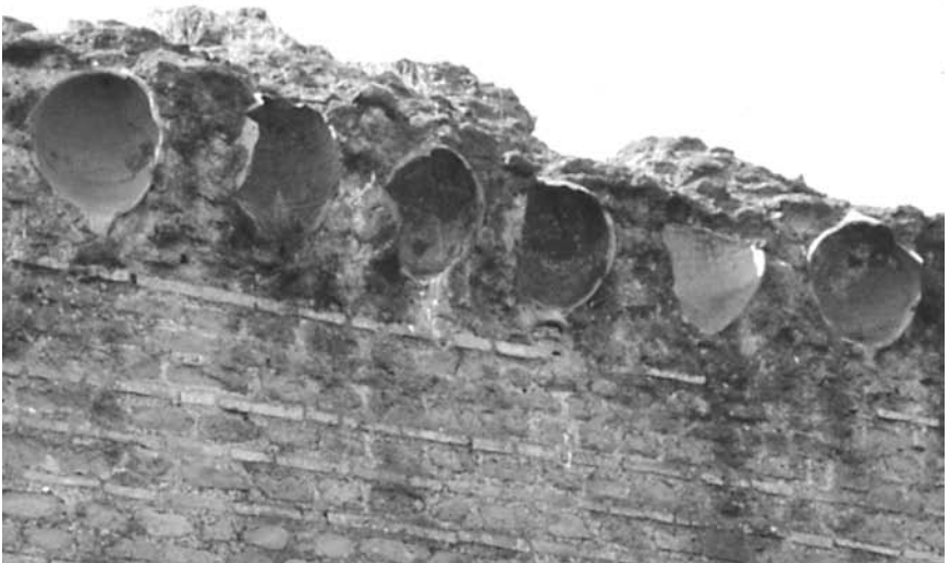
FIGURE 6.18. Dressel 23 amphorae reused as lightning elements in cavea of Circus of Maxentius, near Rome. Left: general view. Right: detail. Photos: JTP.
