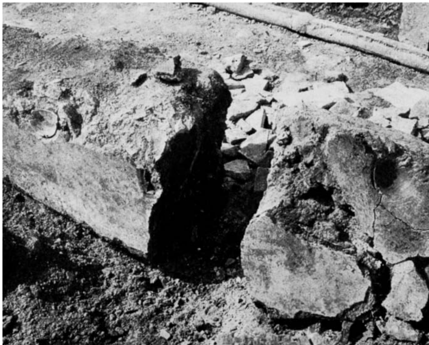
FIGURE 7.8. Fallen masonry from façade of apartment building at Ostia with decorative pottery insets. Ballardini 1964: 32 fig. 44.
