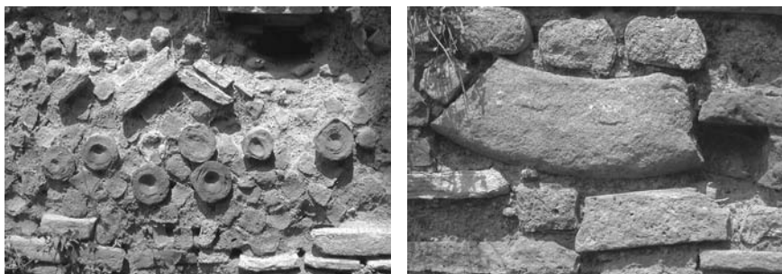
FIGURE 9.2. Detail of pottery recycled as facing in wall shown in Figure 9.1. Left: group of amphora bottoms/spikes. Right: dolium fragment. Photos: JTP.
