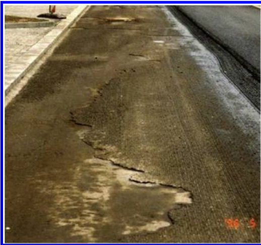
Figure 2. Surface after milling.
