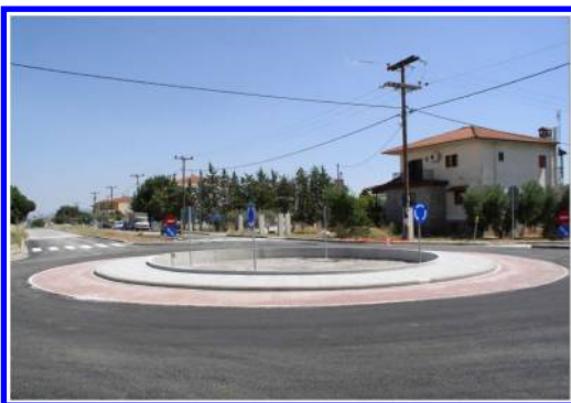
Figure 9. Intersection during the construction of the roundabout (Directorate of Technical Services, Municipality of Thermi, Thessaloniki, Greece).
