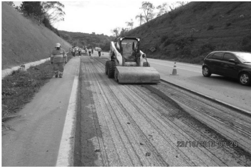
Figure 3. Pavement milling.
