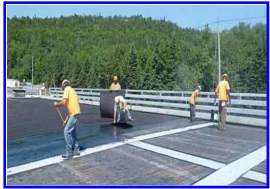
Figure 3. Laying waterproofing membranes over a concrete bridge.
