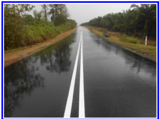
Figure 1. All-weather thermoplastic road markings.
