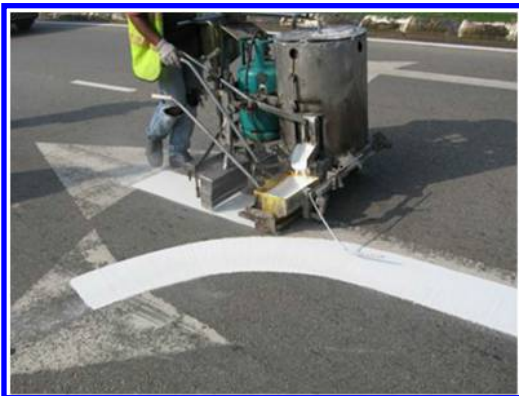
Figure 10. Applicator machine with single-drop facility.
