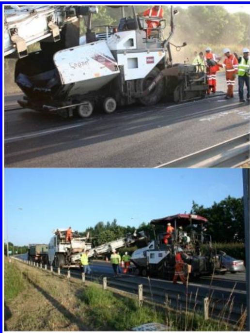
Figure 5. Paving process of the trial section.
