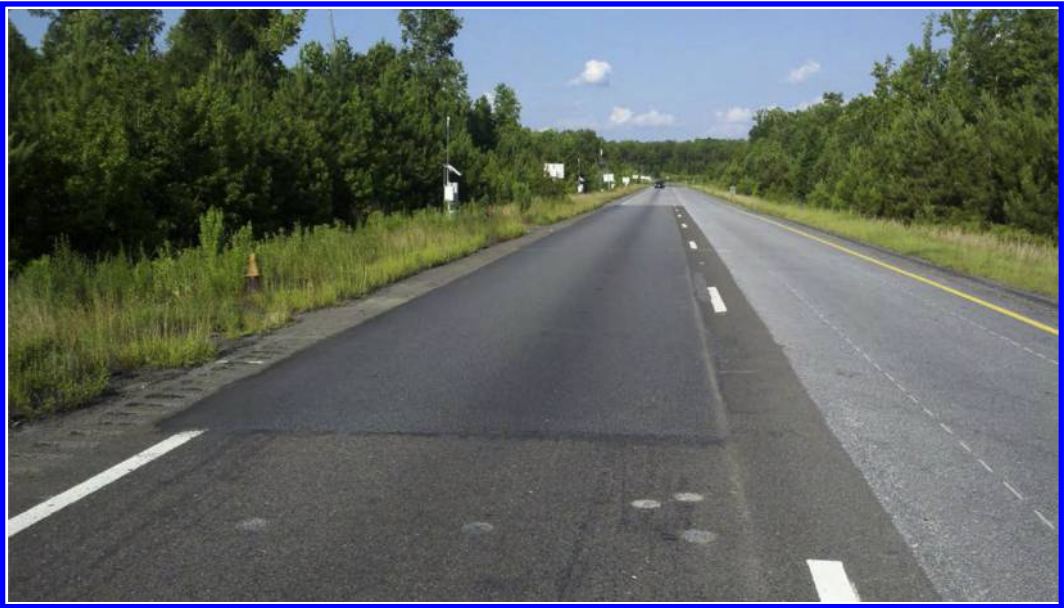
Figure 10. HiMA rehabilitated section N8 after 4.2 million ESALs.
