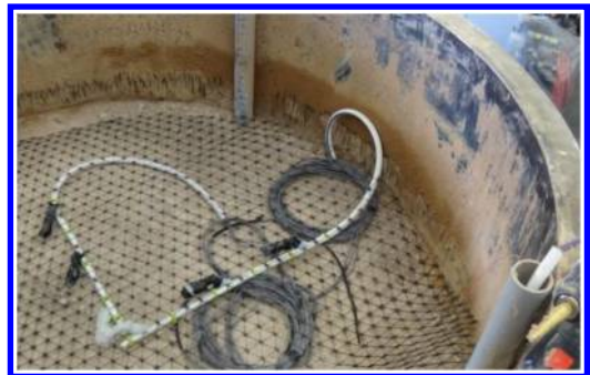
Figure 6. Installation of geogrid and strain gauges.
