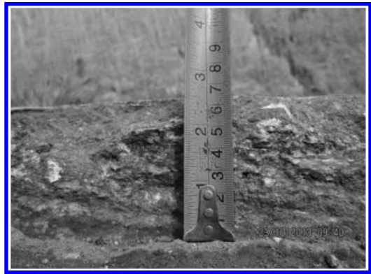
Figure 4. 6 cm of thickness milling.
