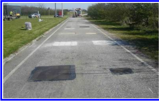
Figure 3. Trial of pothole repair options in Tuelso.
