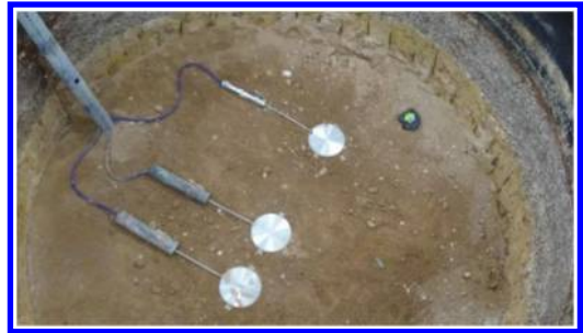
Figure 5. Installation of pressure cells.
