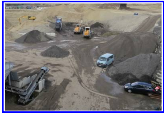
Figure 2. Open air storage of RA at mixing plant.
