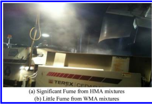
Figure 5. Photos during construction of (a) HMA and (b) WMA.
