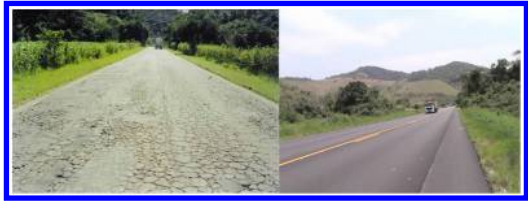
Figure 5. RJ 122 pavement before and after overlay placement with ARFC surface.
