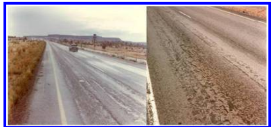
Figure 1. Raveled open graded friction course without asphalt rubber binder.
