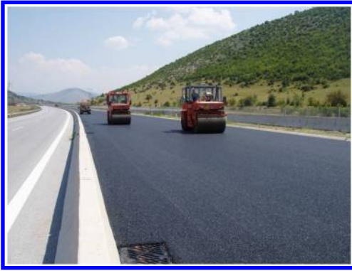
Figure 6. Compaction of AC-VTL (year 2006).
