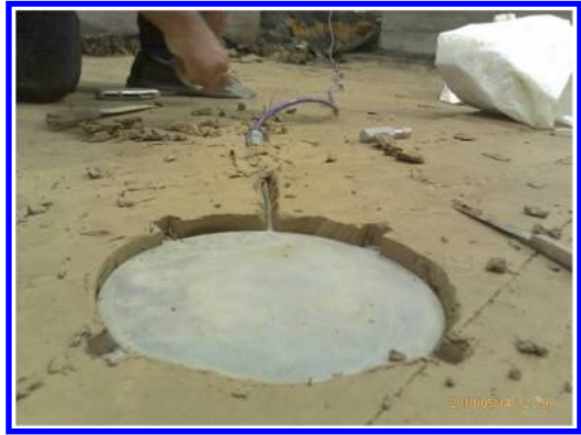
Figure 3. Installation of a pressure cell at PC-1.
