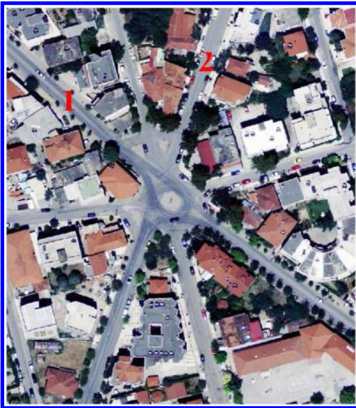
Figure 16. Intersection before the construction of the roundabout ( http://gis.ktimanet.gr/wms/ktbasemap/default.aspx ).
