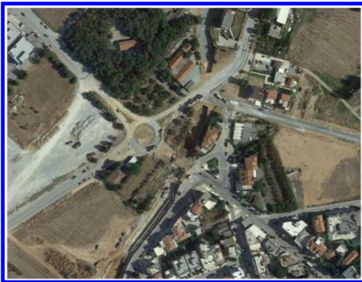
Figure 12. Intersection during the construction of the roundabout ( https://maps.google.gr/ ).
