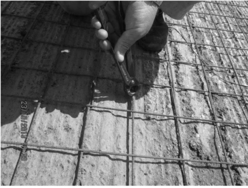
Figure 5. Detail of steel mesh.
