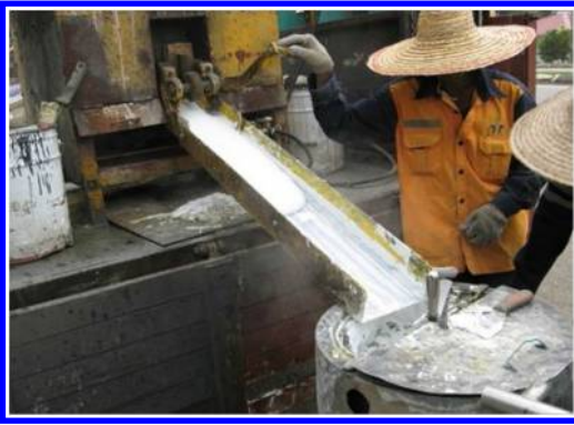
Figure 13. The mixing temperature should be as recommended by the material's supplier.
