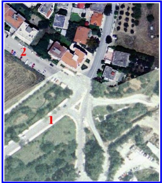
Figure 13. Intersection before the construction of the roundabout ( http://gis.ktimanet.gr/wms/ktbasemap/default.aspx ).
