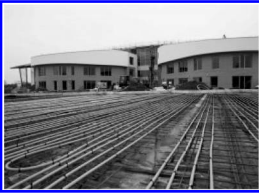
Figure 5. Road Solar Collector pipe system.
