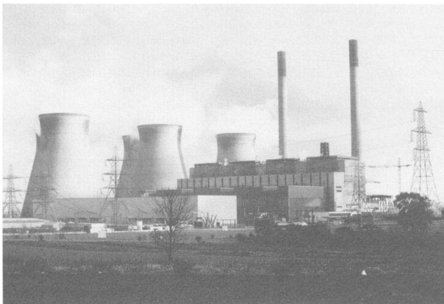
PLATE 3.1 A typical British coal-fired power station. Note that all of the pollutants that are of concern are discharged from the two tall stacks to the right. It is a common public misconception that the large cooling stacks to the left, with huge billowing clouds of steam, are emitting pollutants.
