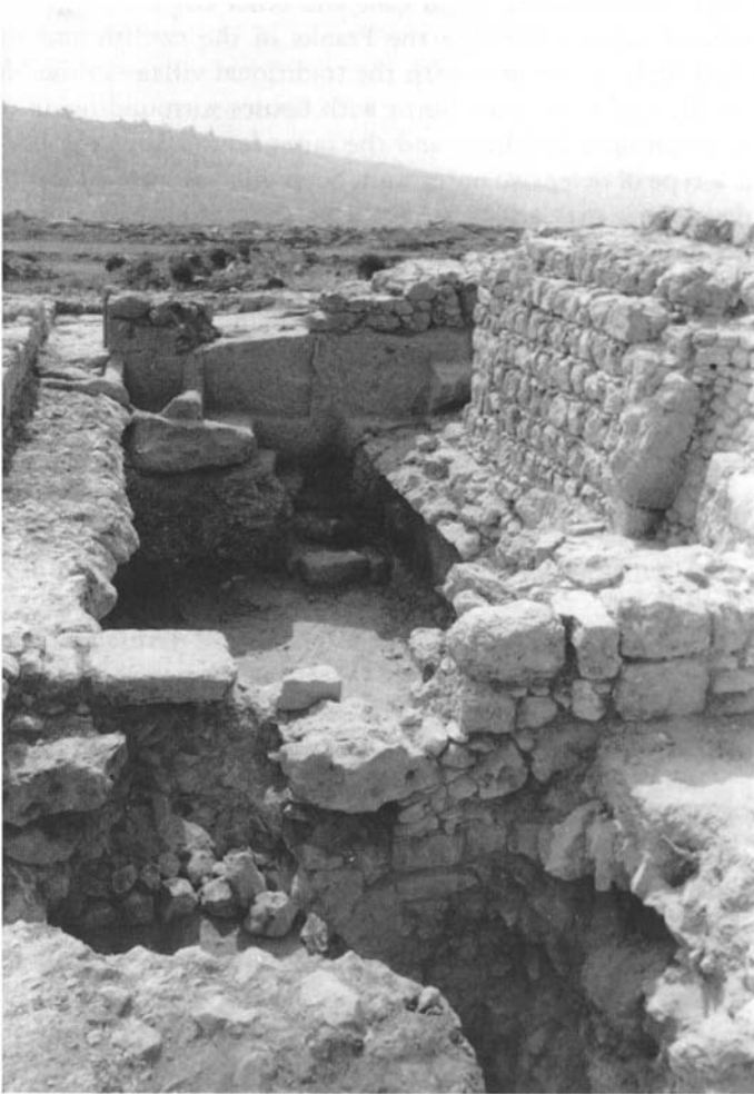
Plate 3.1 Khirbat al-Kurum, a house with an undercroft (photograph by the author)
