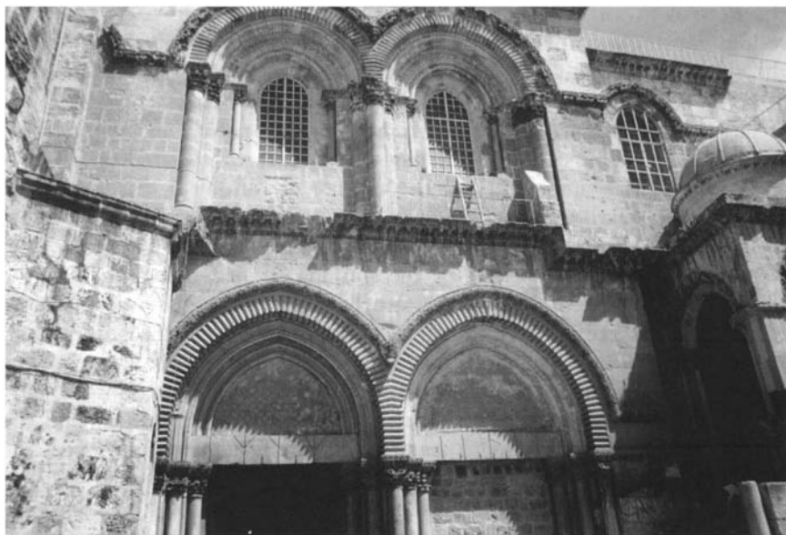
Plate 5.1 South facade of the Church of the Holy Sepulchre (photograph by the author)
