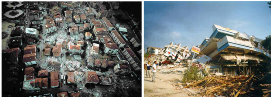
Fig. 1.32 Left Uneven distribution of damage in buildings located in the same area, subjected to the same ground motion. Right Totally collapsed buildings, which killed their occupants
