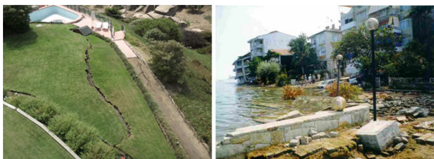
Fig. 1.37 Lateral spreading in the Olas development landscaping during the 2010 Maule, Chile earthquake ( left panel EERI Earthquake Photo Gallery) and buildings dragged into the sea due to lateral spreading in Gölcük during the 1999 Marmara earthquake ( right panel )
