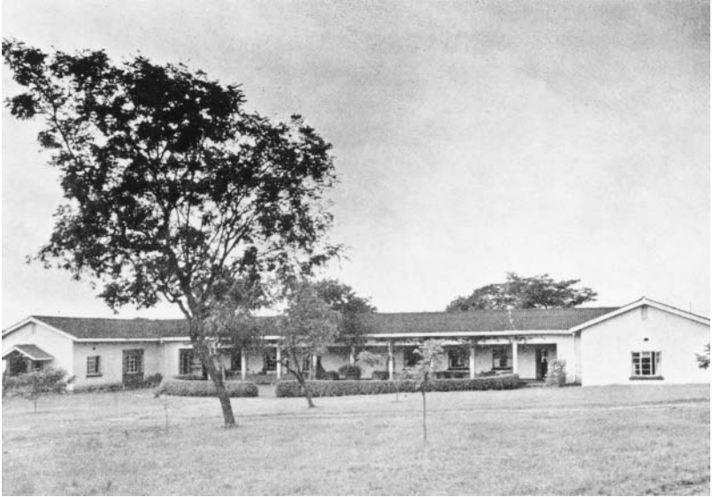
The Institute buildings in Lusaka shortly after construction. (Photo from RLI poster in author's possession.)
