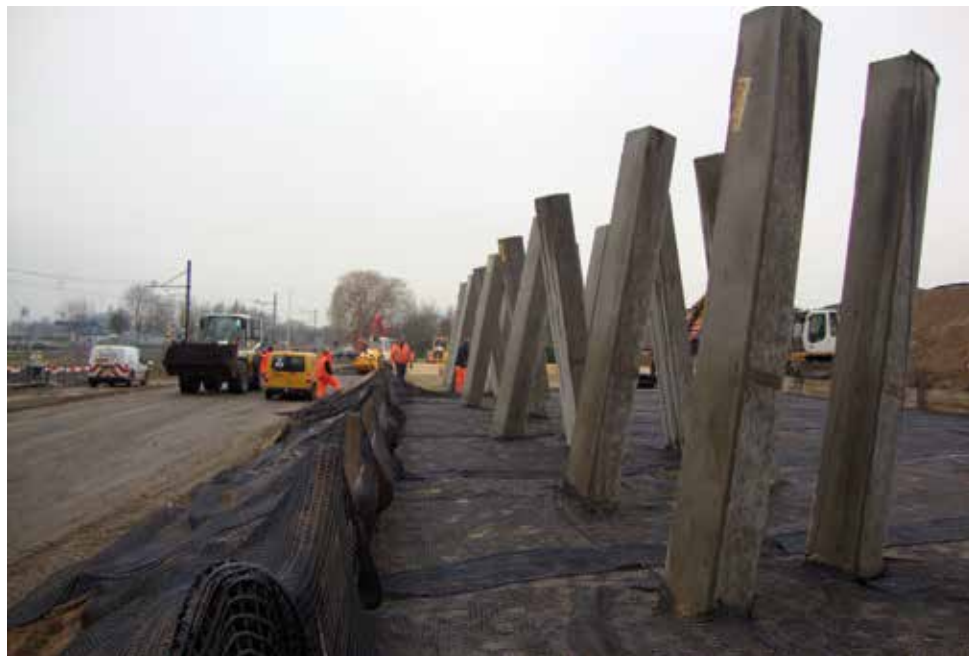
Fig. 8.5 Example of pile openings in reinforced embankment.
