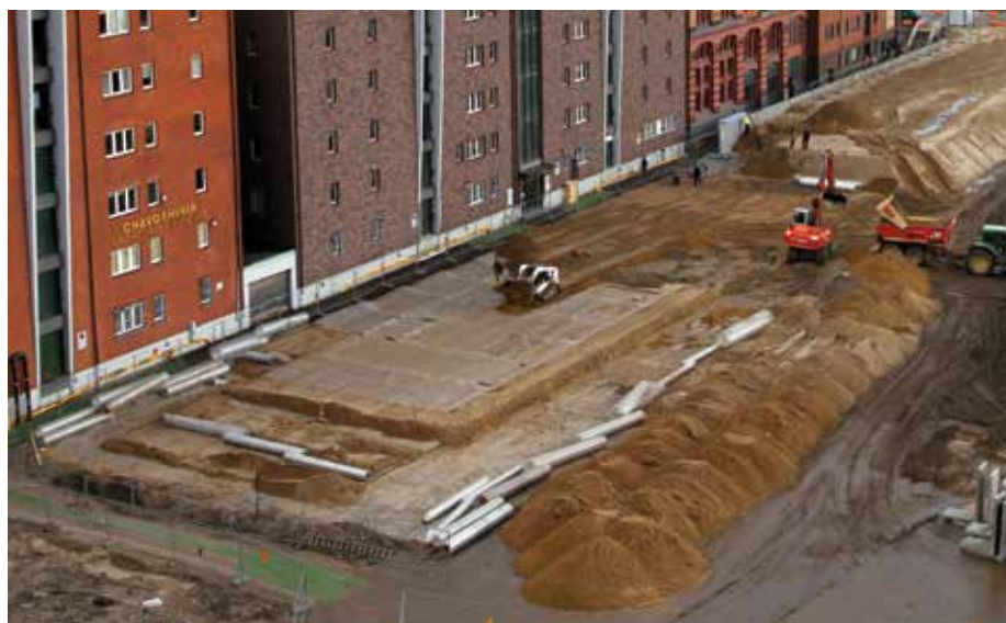
Fig. 8.7 Layer-by-layer filling of a piled embankment at Hafencity, Hamburg, Germany.
