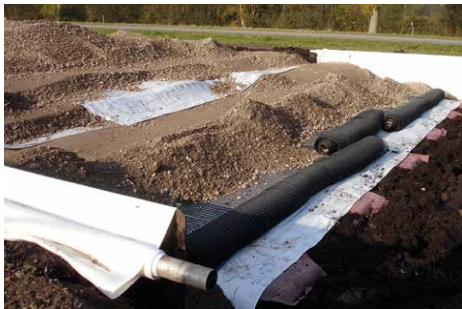
Fig. 8.6 Piled embankment of the N210 at the Krimpenerwaard, The Netherlands; formwork to temporarily enclose the aggregate before the geosynthetic is wrapped back.
