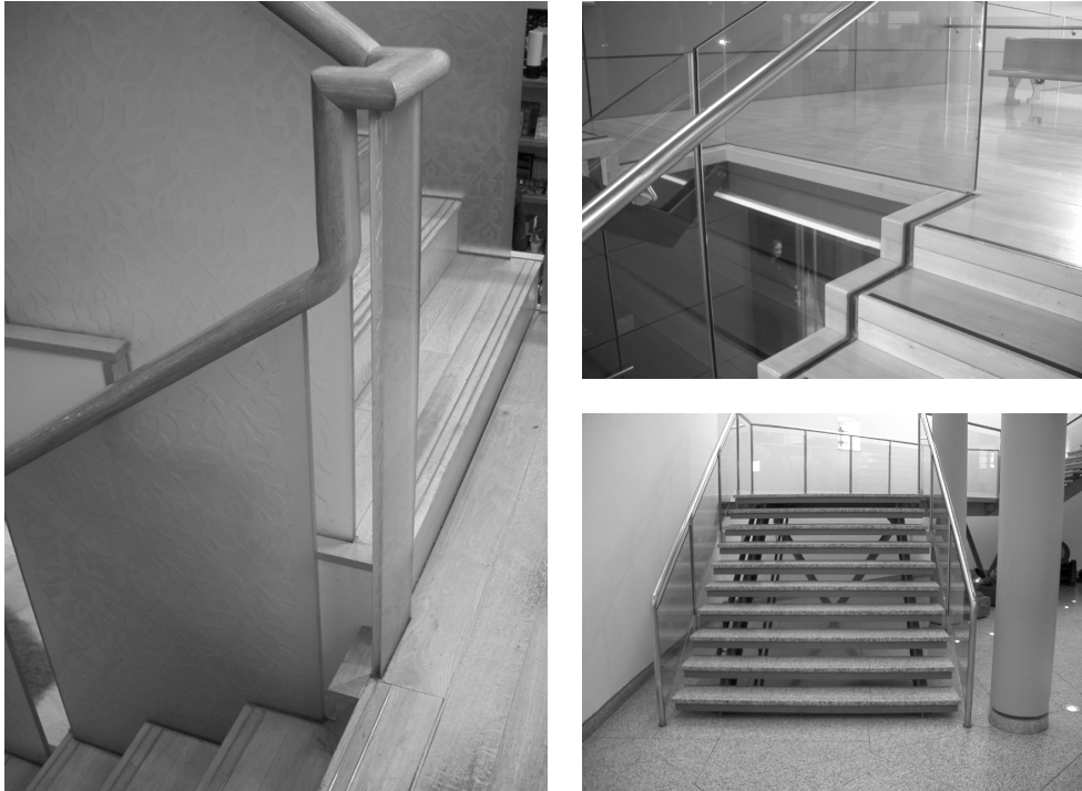
Photograph 9.5 Examples of structural glazing used in stairs.
