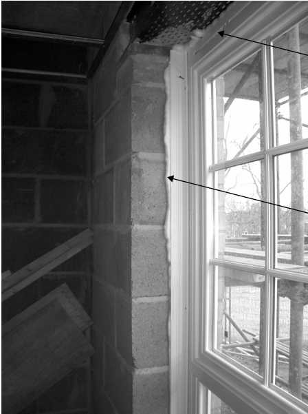
Photograph 7.1 Sealing the gap between window frame and wall.
