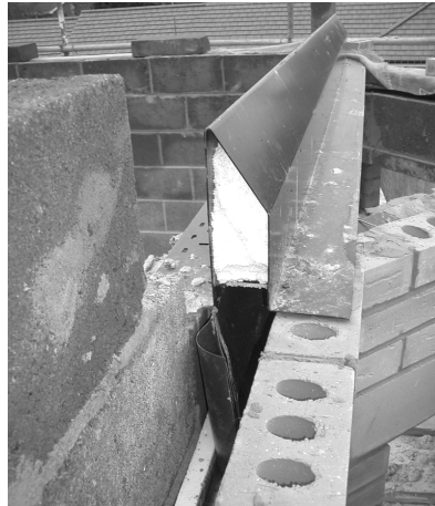
B Lintel placed on cavity wall ready to receive brickwork
