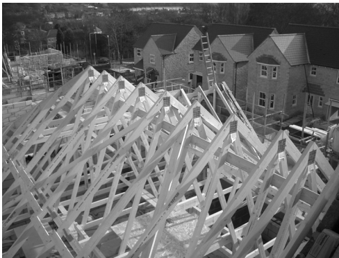
C Diagonal bracing across roof trusses
