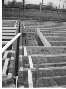
E Joist and joist hangers positioned around floor opening
