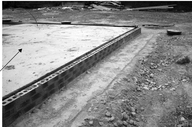
Photograph 3.2 Trenches and ground beams. Source: www.leedsmet.ac.uk/teaching/vsite
