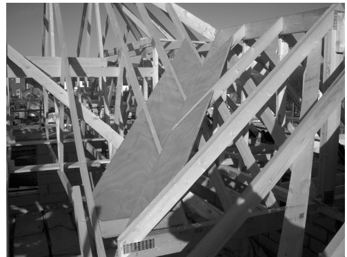
D Forming valley at intersection of roofs
