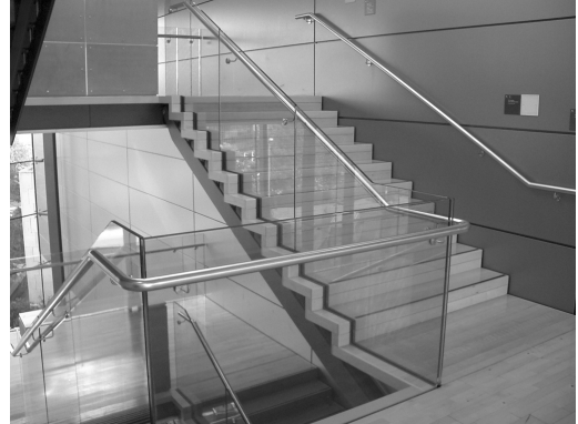
B Glass balustrades provide a feature, expose movement of people and reduce the risk of children climbing
