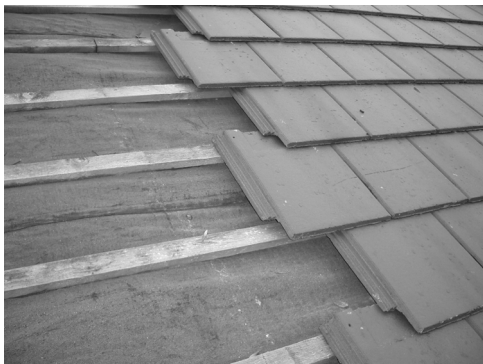
C Interlocking single tiles fixed to battens.
