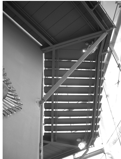
D The heavy cantilevered supporting steel structure has a visual impact. Open stair allows external light to penetrate gaps
