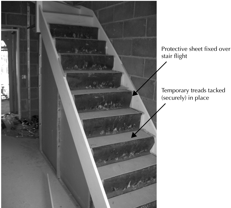
Photograph 9.4 Temporary protection of timber stairways.
