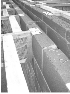
D Joists fixed into steel joist hanger. Horizontal strutting holds the joists firmly in place
