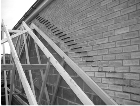
A Truss rafters ready to receive sarkin felt and roof battens.
