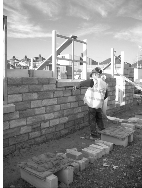
B Alternatively, cavity closer can be assembled providing a permanent opening former. The opening formers are held in place with temporary props.
