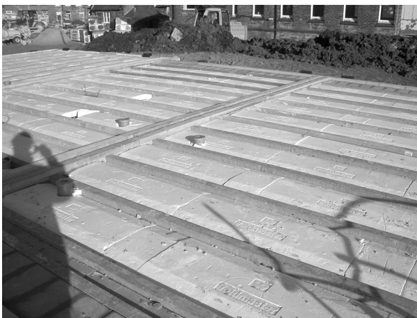
Photograph 4.2 Precast concrete 'T' beams and insulation infill panels.
