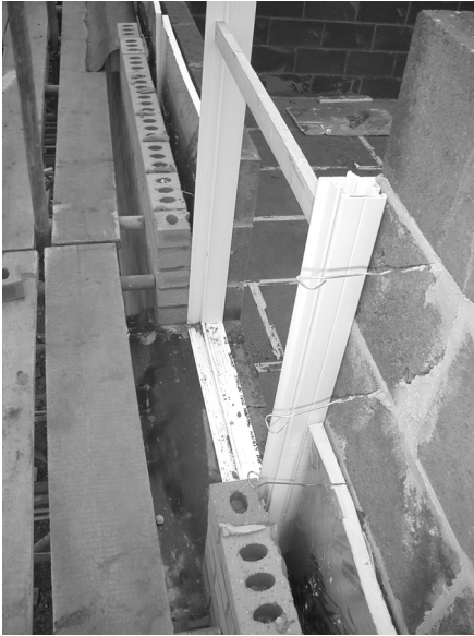
A Cavity closer and window opening former
