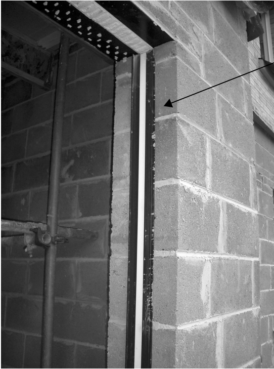
Photograph 5.4 Sealing the cavity in a wall opening: cavity closer
