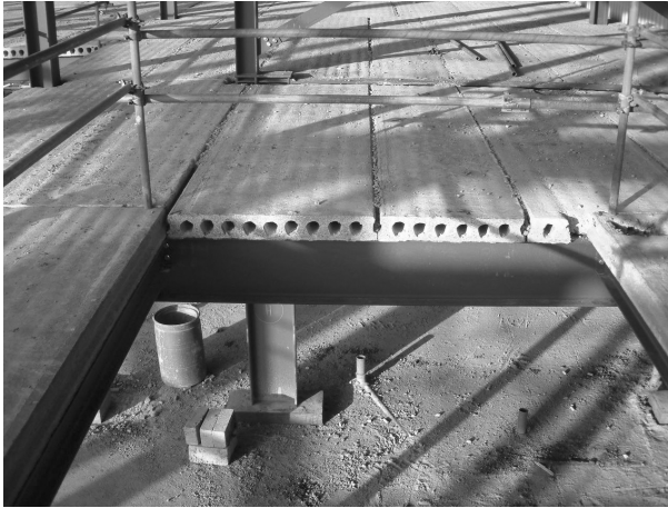
A Concrete floor beams
