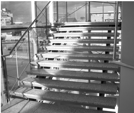
C Open stairways with glass handrails, behind glass cladding combine internal and external features to enhance views from inside and outside the building
