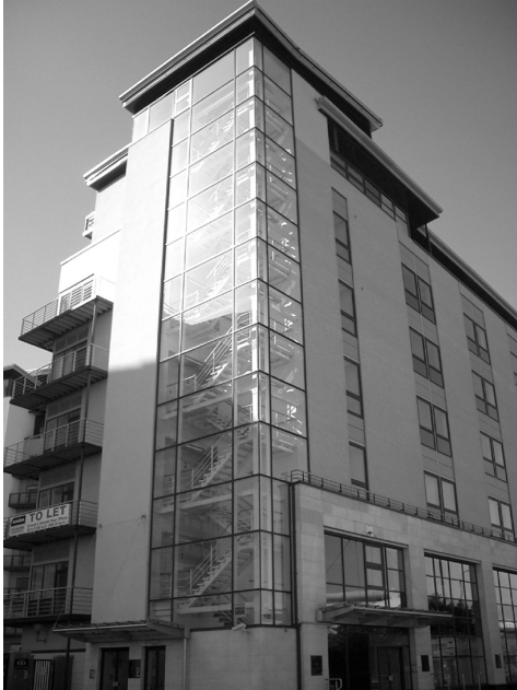
A Stairway: glass cladding exposes stairway to the public
