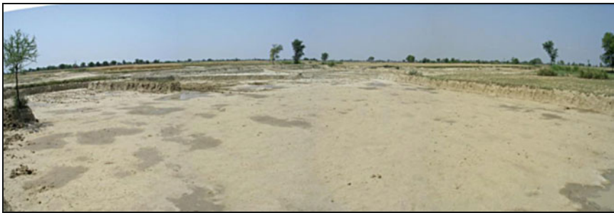
Site of soil excavation
