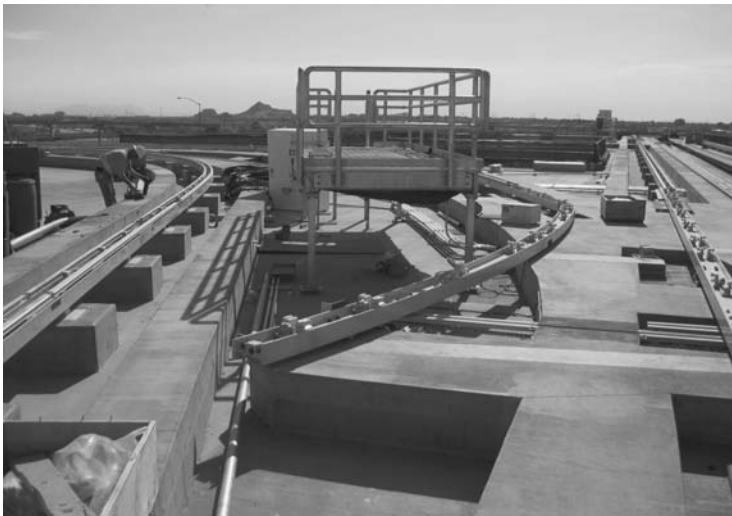
Figure 6. Switch Component Install
