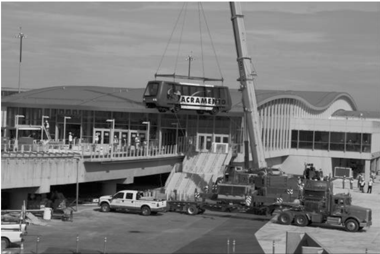
Figure 9: March 17, 2011 – Vehicle being lifted onto the Guideway - Bombardier
