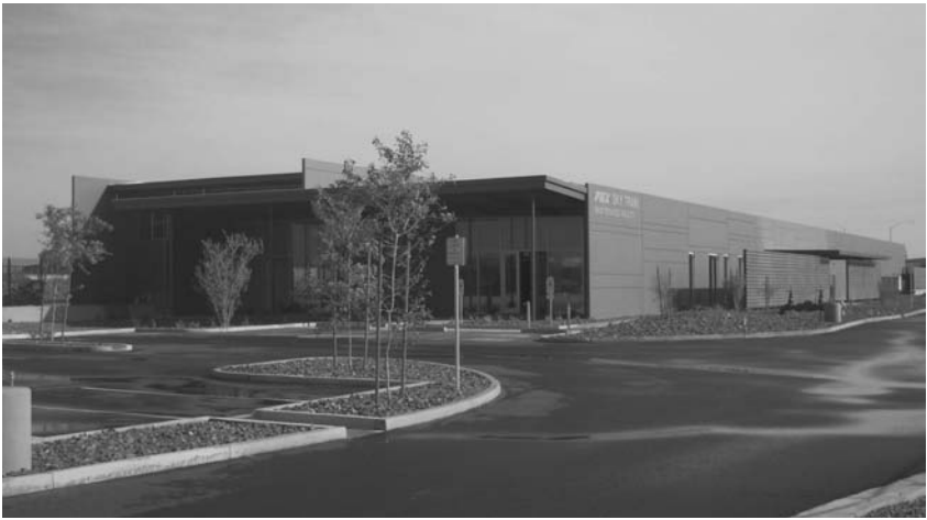
Figure 3. Maintenance and Storage Facility (Sky Harbor International Airport)
