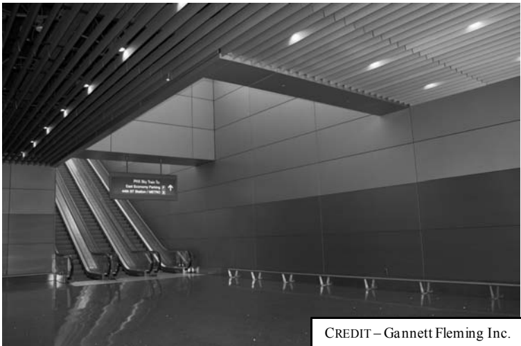
Figure 16 – Metal Wall Panels & Baffle Ceiling at Terminal 4 Station
