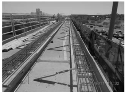
Figure 16: Plinth Reinforcing
