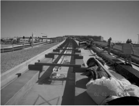
Figure 18: Guide Beams and Jigs
