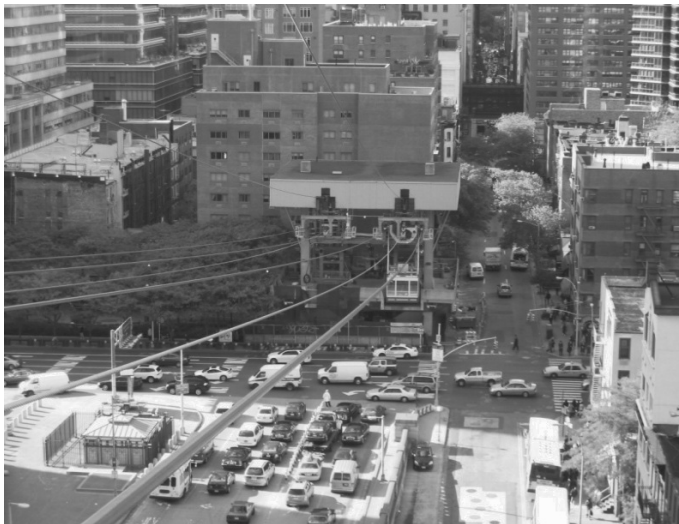
Picture 10 – Manhattan Station Looking West (ESG)
