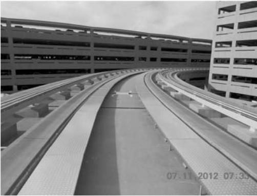
Figure 26: Cable Tray Superelevated Guideway
