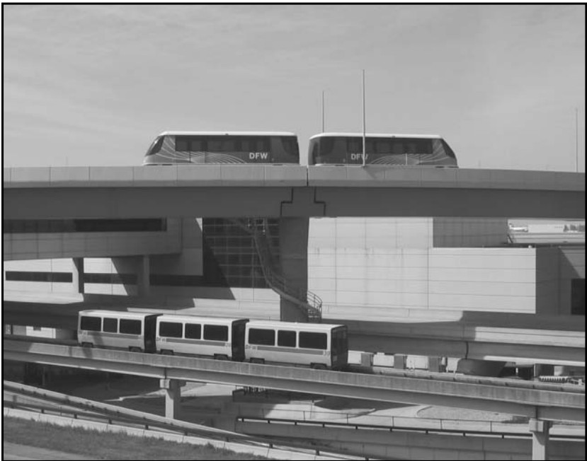
Figure 7: A Skylink train passes over a soon-to-be decommissioned Airtrans train at DFW Airport in 2005 (Ronald Sheahan, Lea+Elliot)
