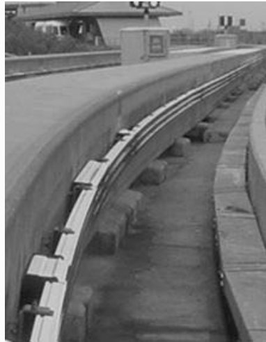
Image 20: Curved Guideway section with an expansion (long overlap cover) between two splice assemblies, Conductix Inc.
