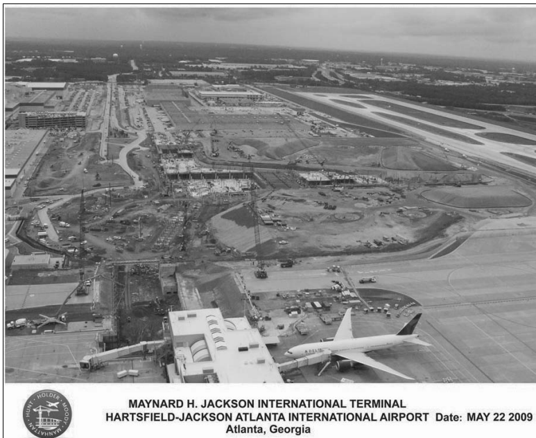
Figure 2. Looking East, International Terminal Tie-In Point in 2009 (3)
