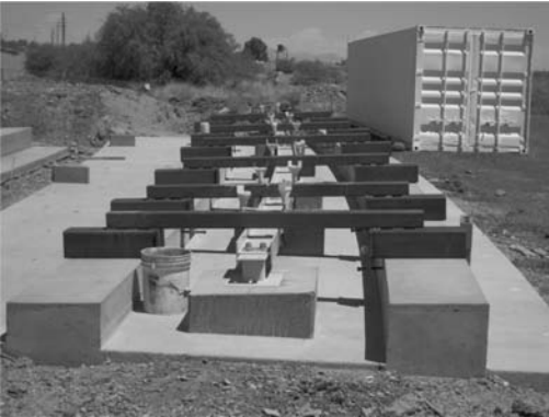
Figure 8: Final Guidebeam Jig Assembly
