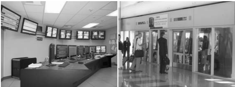
Figure 4: Central Control Operations (left) and Platform Screen Doors (right) - Bombardier
