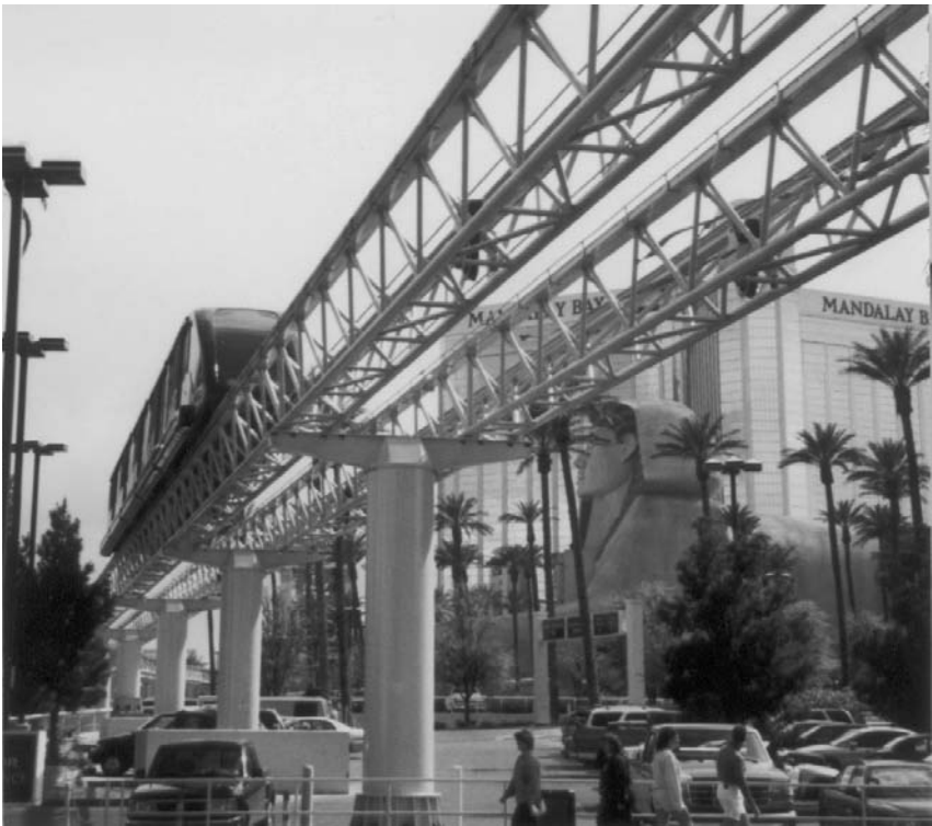
Figure 1. Mandalay Bay Guideway.
