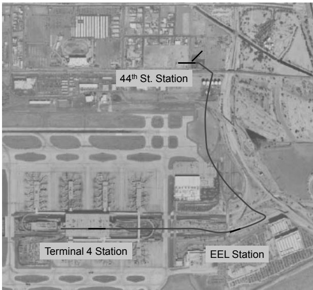
Figure 2. The Stage 1 System (Sky Harbor International Airport)
