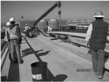
Figure 20: Guidebeam Placement
