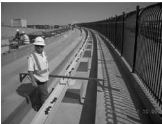
Figure 11: Beam Alignment Tool in Use
