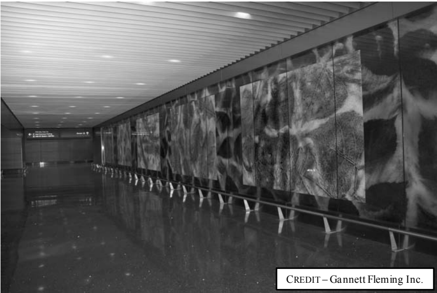
Figure 18 - Art Glass Wall @ Terminal 4 Station Connector Bridge
