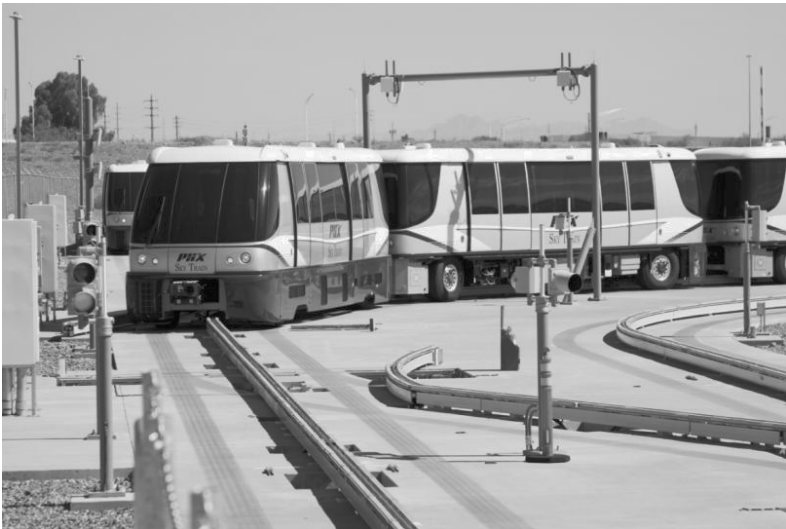
Figure 3: Photo[3] Access points in Maintenance Area.
