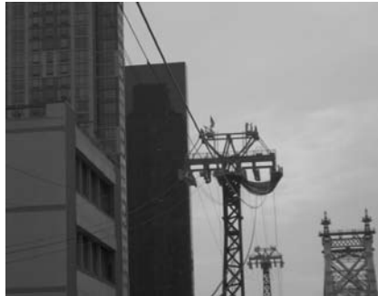
Picture 9 – Tower Top Construction Protection (ESG)
