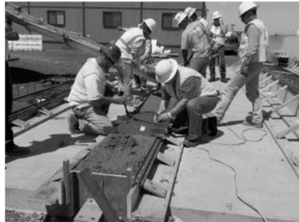
Figure 14: Floating Exp. Joint Assy.
