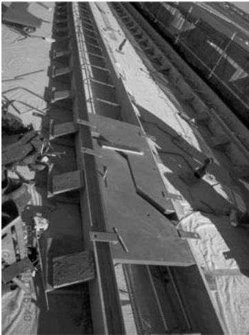
Figure 13: Expansion Joint Tie Downs
