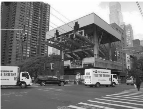
Picture 7 - Manhattan Station Looking Southwest (ESG)
