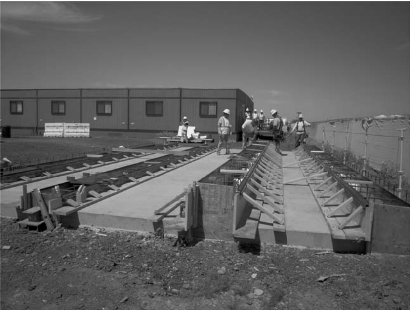
Figure 3: Guideway Mockup 1A – Straight Section
