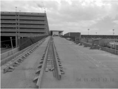
Figure 15: Horizontal Slip Forms
