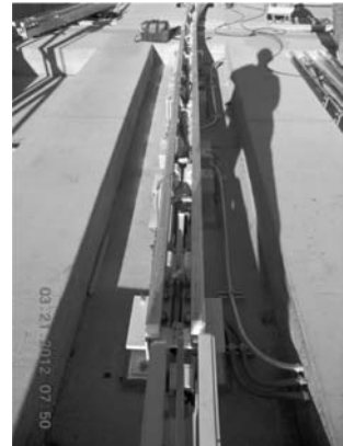
Figure 22: Power Rail Installed
