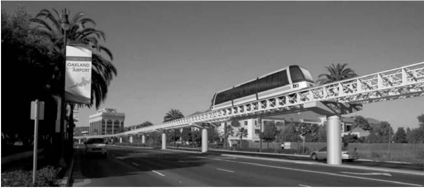
Figure 2. DCC Open Truss Guideway along Hegenberger Road (Courtesy of BART / FPJV)
