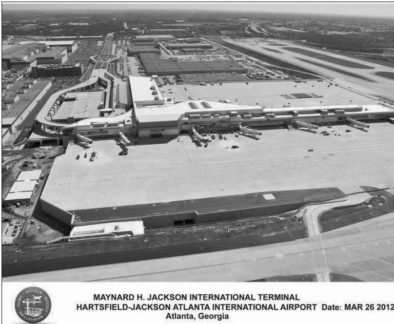
Figure 3. Looking East, International Terminal Tie-In Point in 2012 (3)
