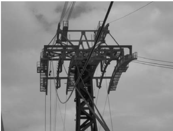
Picture 12 – Rope Installation Detail (ESG)
