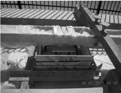
Figure 19: Guide Beam Pedestal Forms
