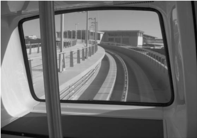
Figure 2: APM Guideway – The Vital Link - Bombardier
