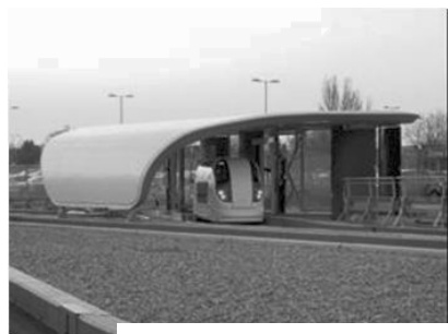
Figure 3 Station in Car Park
