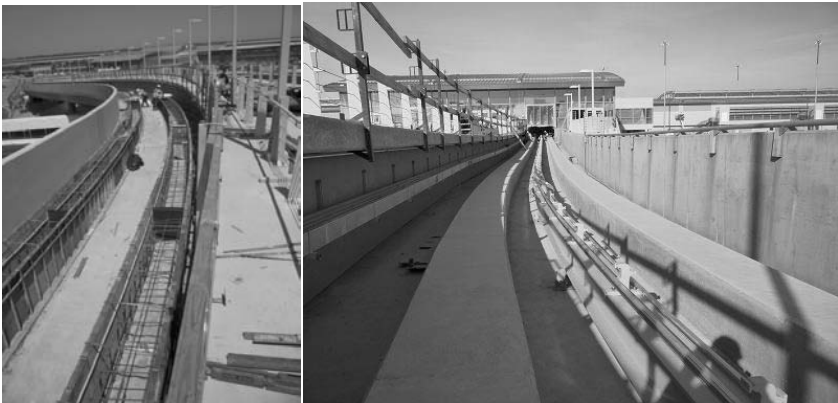
Figure 10: Running Beam and Guidebeam Installations – Bombardier
