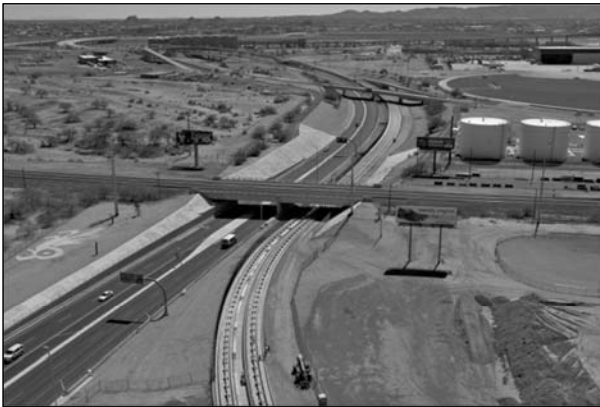
Figure 7 - APM Crossing UPRR , photo courtesy of Hensel Phelps Construction Co.
