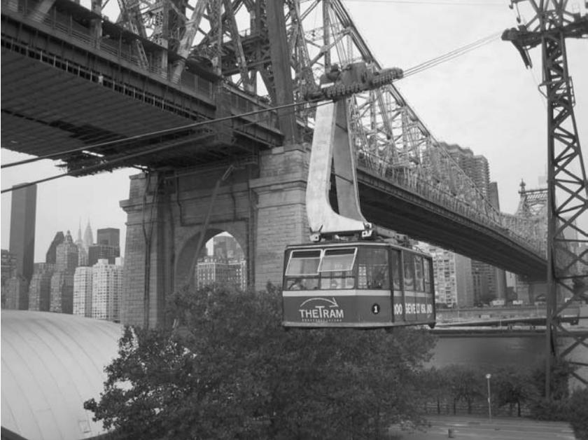
Picture 1- Original Tram-Queensboro Bridge (59 th Street) Looking West (ESG)
