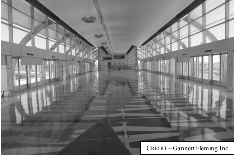
Figure 15 – Terrazzo Floors & Metal Ceiling at 44 th Street Station
