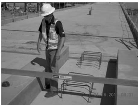
Figure 17: Flatness Testing
