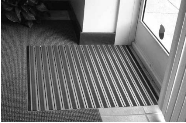
Figure 6-13 Sample entryway grate.
