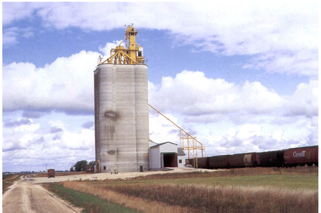
Plate 12 A new-style, yellow and white Manitoba Pool elevator at Tucker Siding, just east of Portage. This elevator, which has an exposed leg, opened in 1986, replacing older-style elevators at Portage. Capacity is 5,500 tonnes (J. Everitt).
