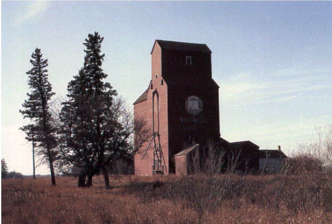
Plate 11 Bradwardine elevator, now closed. An old-style, red-painted Manitoba Pool elevator with annex. This elevator, which had a capacity of 57,500 bushels (approximately 1,610 tonnes), was located on the now-abandoned Great North West Central Line (the Lenore extension; Case Study 14.2 on page 217) (J. Everitt).
