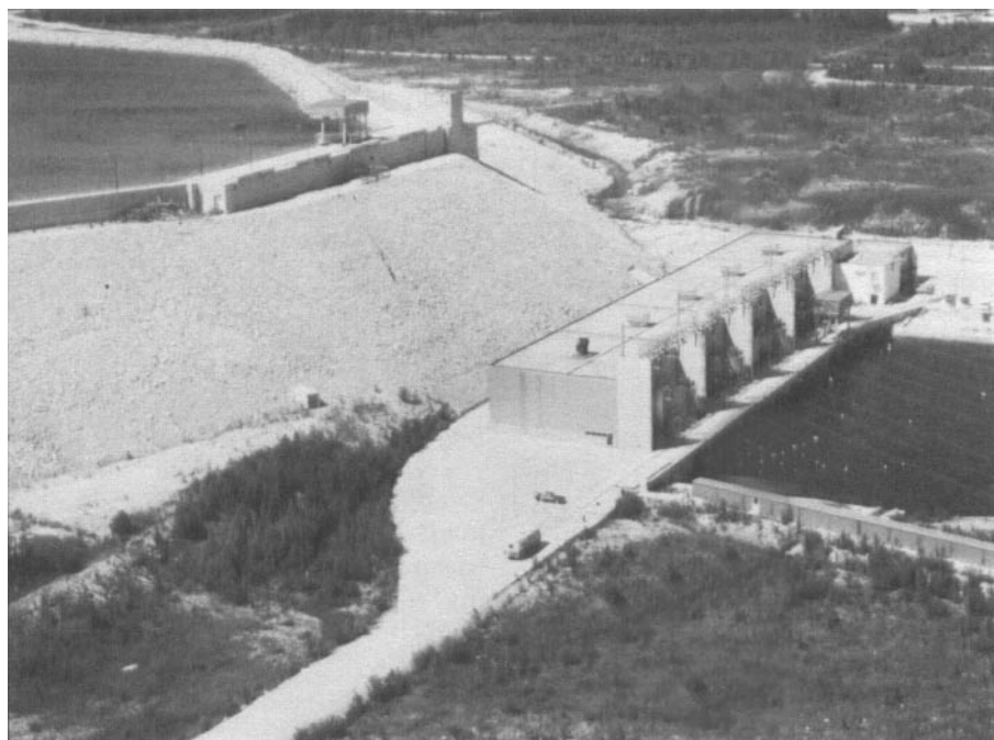
Figure 18.7 Hydro-electric Power Station at Grand Rapids, on the Saskatchewan River West of Lake Winnipeg. This was the first hydro station in "northern" Manitoba and, with a fall of 36.5 m, has the greatest head of any Manitoba station. (Photograph: Manitoba Hydro)
