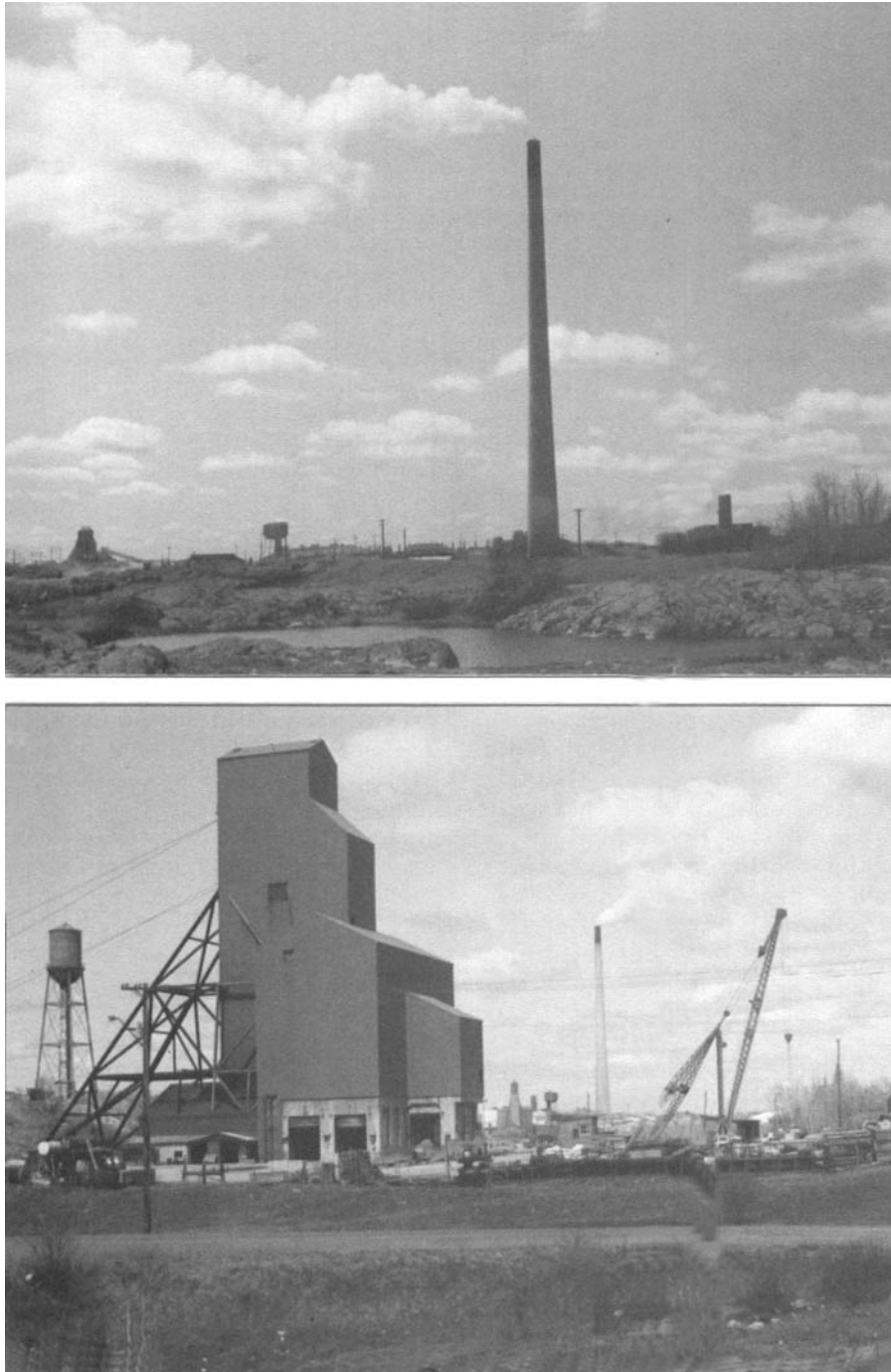
Figure 16.9(a) Hudson Bay Mining and Smelting Complex at Flin Flon; (b) Headframe, South Main Mine, Flin Flon. (Photographs: H. Young)
