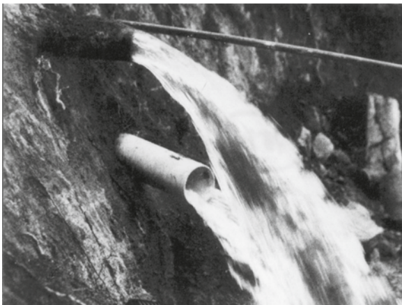
Fig. 17.5 Example of horizontal wells tapping weathered andesite at a height of 2400m above m.s.l. in the Lake Tahoe Basin, California, USA. (After Matthews 1985)
