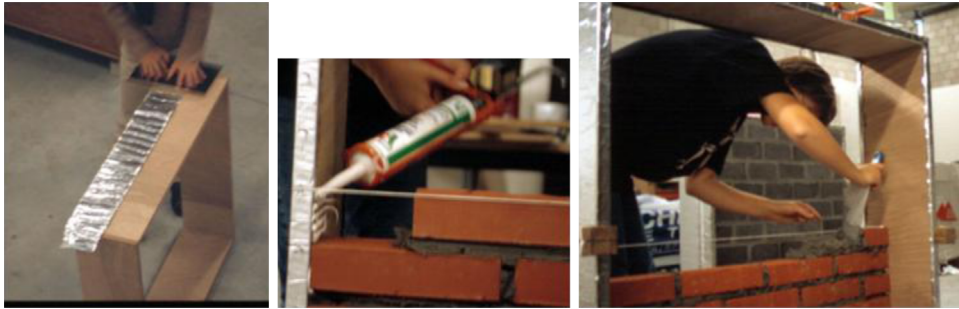
Figure 6.1 Preparing wall samples for measuring the air permeance.
