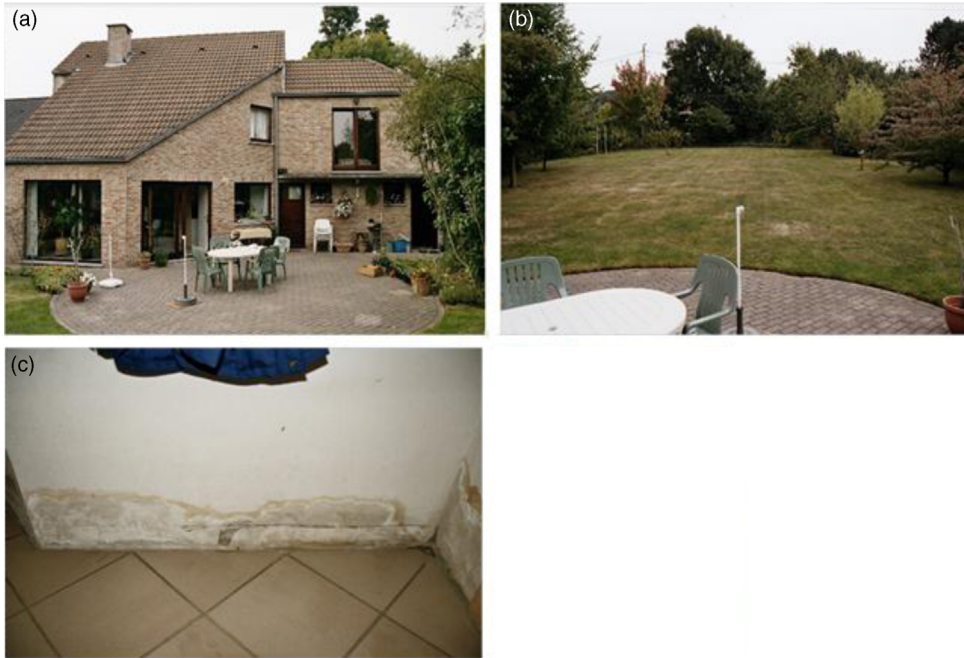
Figure 4.33 (a) Villa, (b) sloping garden and terrace, (c) rising damp in a partition wall.
