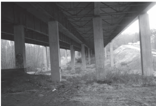
Bridge under view.
