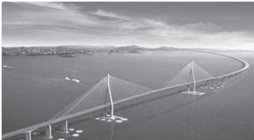
Figure 1. Incheon Bridge, Cable stayed Bridge, Main span length = 800 m.
