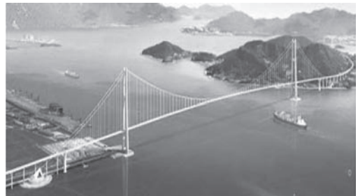
Figure 2. Leeshunsin Bridge, Suspension bridge, Main span length = 1545 m.
