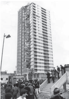
Figure 1. Ronan point collapse.
