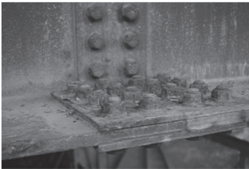
Figure 2. Corrosion shortcoming.
