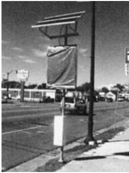
Figure 1: Pole-mounted, SMD just after installation
