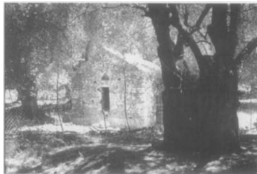
Figure 4.2 The chapel of Sotiris o Christos, south-west Crete: olive trees, c. 275–300 years old, seal the deposit which has buried the foundations of the chapel.
