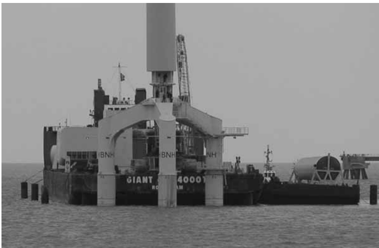
16.8 BARD Tripile foundation for the Hooksiel demonstration plant (© BARD Engineering GmbH).
