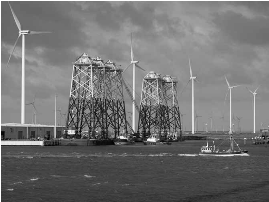
16.6 Jackets for the test field Alpha Ventus (© DOTI 2009, Photographer: Mathias Ibeler).
