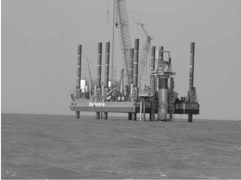
16.23 Driving of a monopile with a jack-up unit (© RWE Innogy GmbH).
