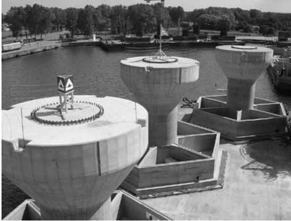
16.4 Fabrication of concrete gravity based foundations, for the Lillgrund wind farm, on special barges (© HOCHTIEF Construction AG, Civil Engineering and Marine Works, Hamburg, Germany).
