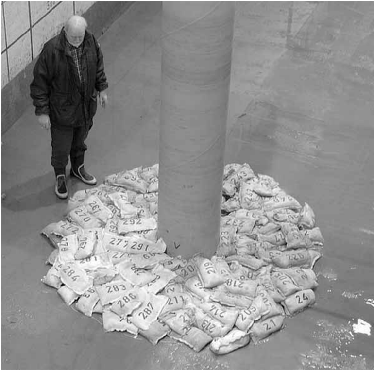
16.22 Geotextile containers as scour protection around a monopile (© Forschungszentrum Küste).
