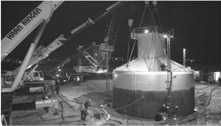
16.11 Prototype of a suction bucket foundation for a 3 MW offshore wind turbine in Frederikshavn (DK) (Ibsen, 2008).
