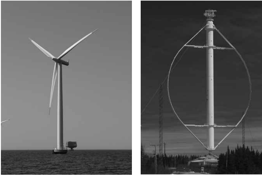
6.1 Left, horizontal axis wind turbine (HAWT): Siemens 2.3 MW wind turbine, 69 m hub height, situated at Rødsand, Denmark (Photo by Christian Bak, Risø DTU). Right, vertical axis wind turbine (VAWT): Éole 4 MW wind turbine, height of 110 m, situated at Cap Chat, Quebec, Canada (Photo by Paul Gipe).
