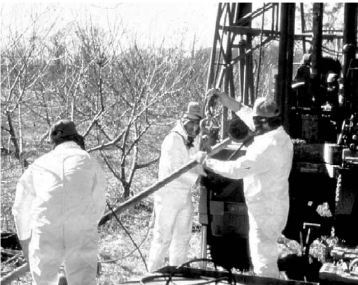
FIGURE 15.3 Workers in Level B protective clothing with supplied air respirators (SAR). (Courtesy of URS Corporation, 100 California Street, San Francisco, CA.)
