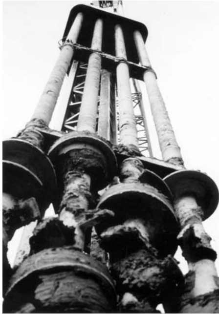
FIGURE 11.15 Deep soil mixing equipment used in situ solidification. (From Geo-Con Incorporated, 4075 Monroeville Blvd., Suite 400, Monroeville, PA 15146. With permission.)
