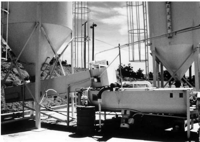
FIGURE 7.16 Solidification process. Pugmill mixing and related equipment.
