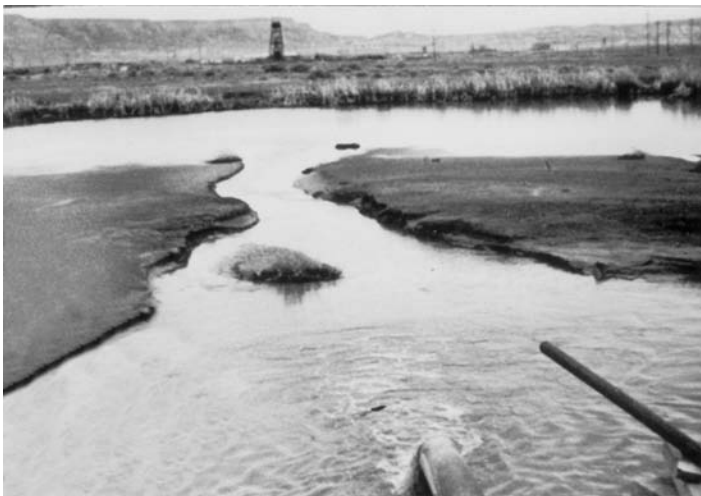
FIGURE 1.14 Surface impoundment. (From the U.S. Environmental Protection Agency.)
