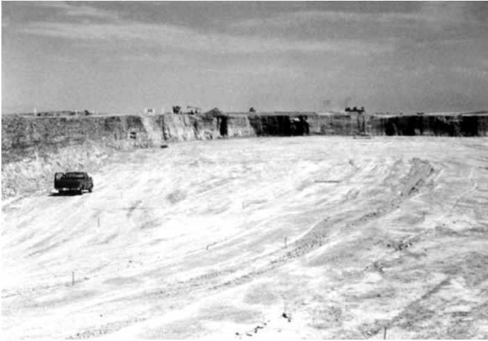
FIGURE 11.18 Extent and magnitude of excavation necessary to “clean-close” a former hazardous waste impoundment. (Courtesy of Safety-Kleen Corporation.)
