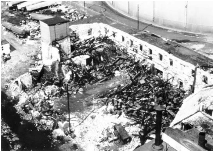
FIGURE 1.5 ABM-Wade site (Chester, Pennsylvania). (From the U.S. Environmental Protection Agency.)
