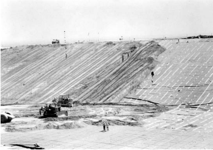
FIGURE 7.30 Liner bedding for protection from puncture.
