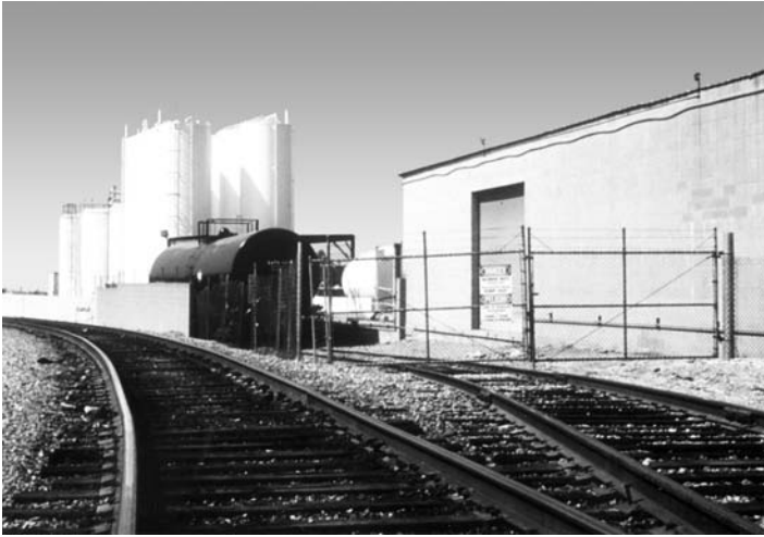
FIGURE 7.1 Site security requirement for RCRA sites.
