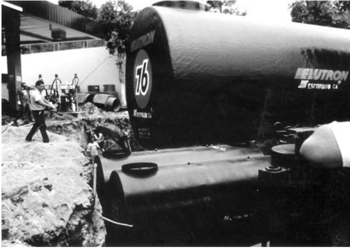
FIGURE 14.6 Composite steel-fiberglass reinforced plastic tanks.
