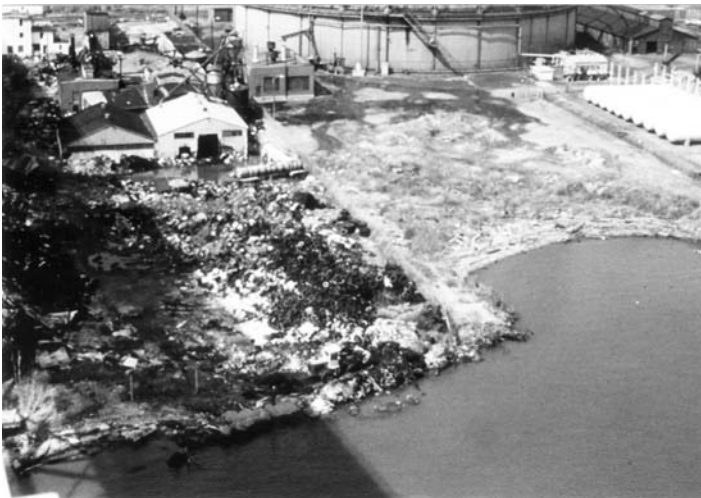
FIGURE 1.7 ABM-Wade site (Chester, Pennsylvania). (From the U.S. Environmental Protection Agency.)
