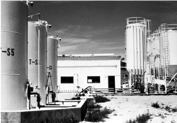
FIGURE 7.14 Solidification process. Liquid waste storage and blending.
