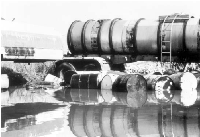
FIGURE 1.9 ABM-Wade site (Chester, Pennsylvania). (From the U.S. Environmental Protection Agency.)
