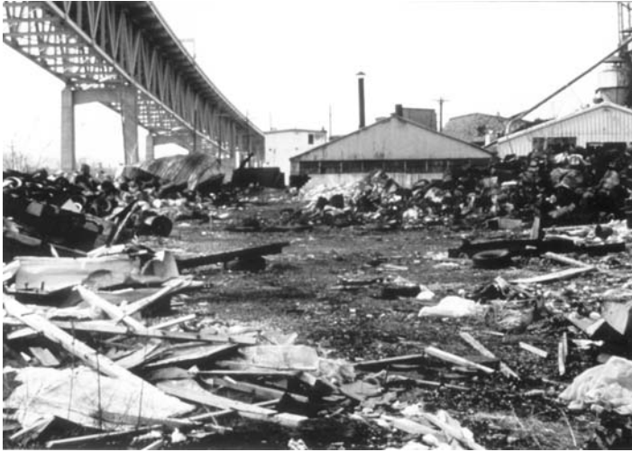
FIGURE 1.6 ABM-Wade site (Chester, Pennsylvania). (From the U.S. Environmental Protection Agency.)
