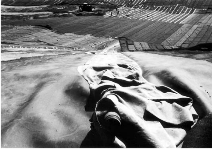
FIGURE 7.28 Secure landfill leachate detection and monitoring access gallery.
