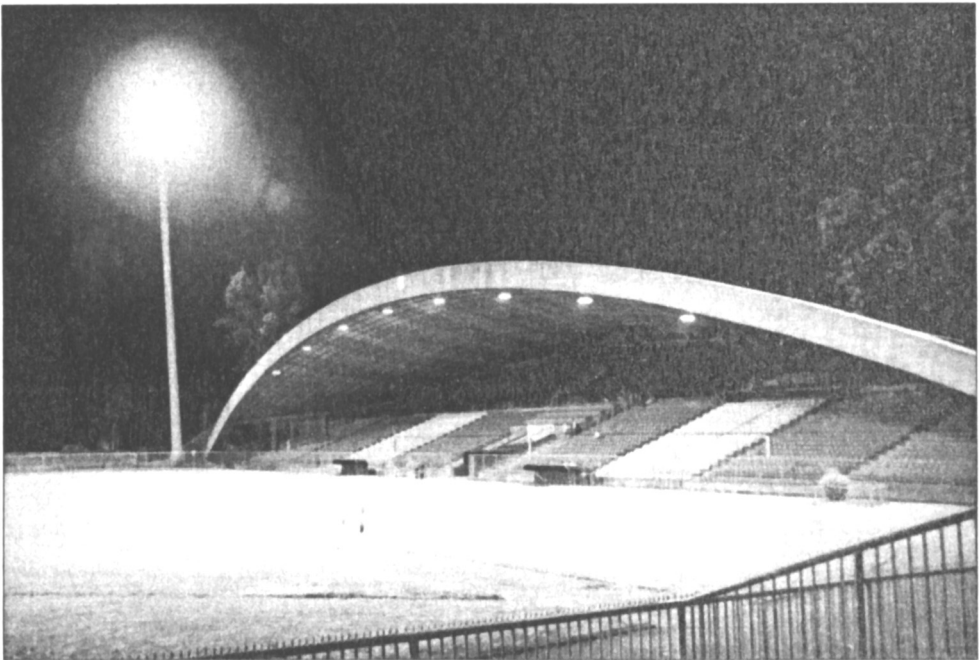
Figure 1.1: An example of CAD design (top picture) and photograph (bottom picture) of the sports stadium in the city of Maribor
