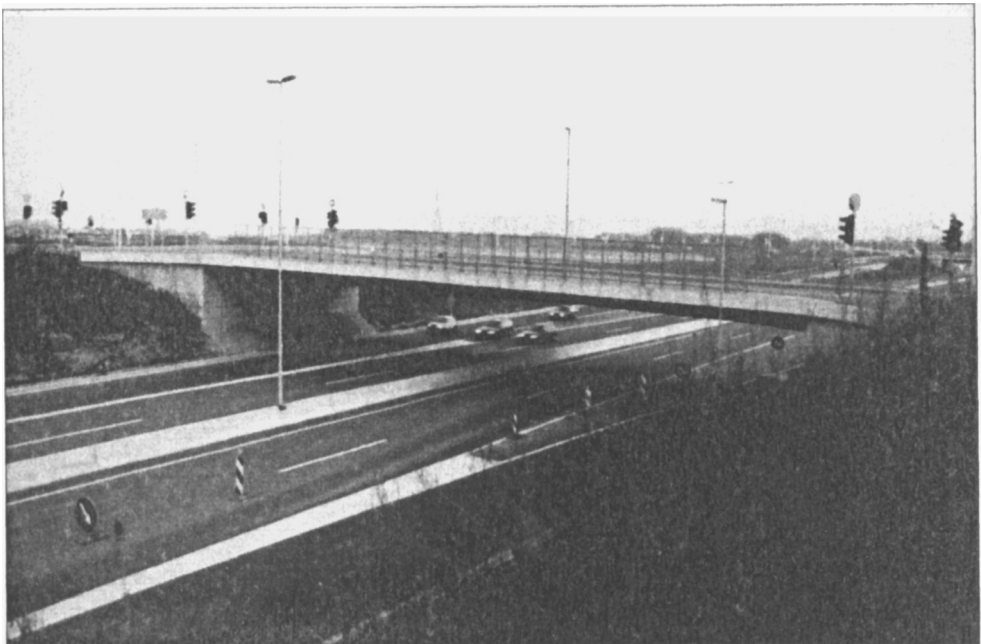
Figure 1.11: The bridge on East Highway, Ljubljana (Courtesy of Gradis BP Ltd.)
