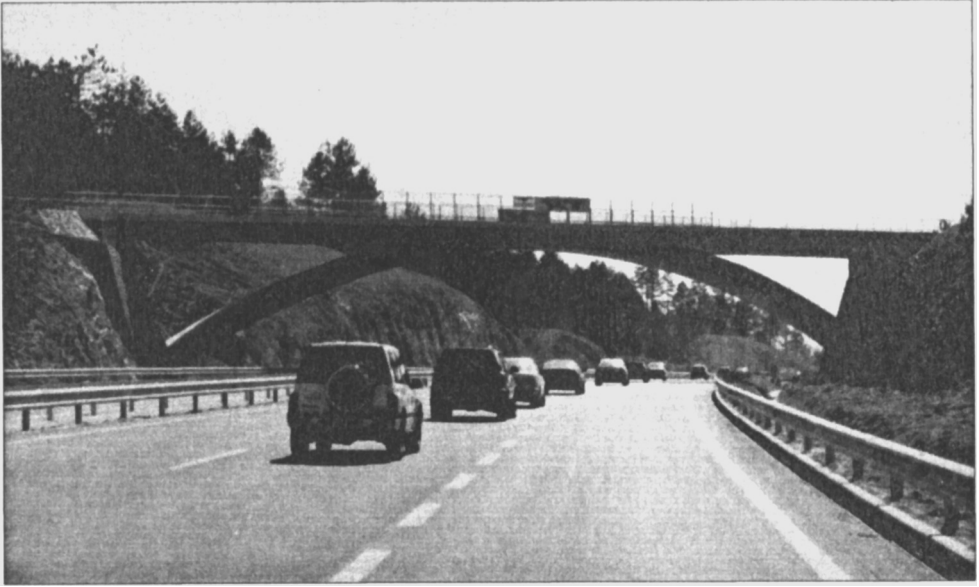
Figure 1.8: The bridge at Kozina (Courtesy of Ponting Ltd.)
