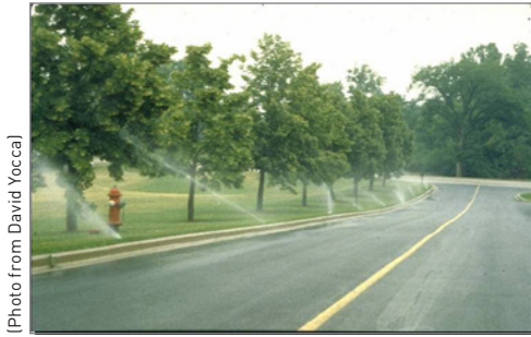
FIGURE 3-68: Conventional above-ground lawn irrigation systems can use considerably more water than is necessary due to overspray, excessive overlap of head ranges, leaks, evaporation, or poor maintenance of the system.
