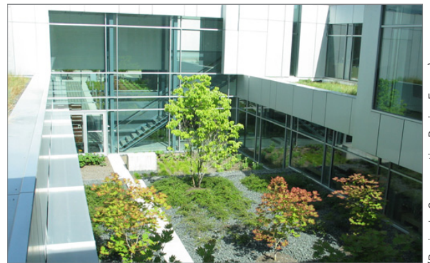
FIGURE 4-14: The green roof courtyard at the Kresge Foundation in Troy, MI, accommodates large- and small-scale vegetation.
