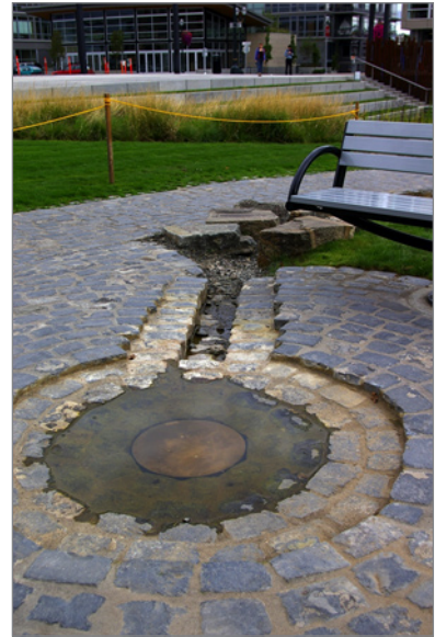
FIGURE 3-17: The recirculating rain water system at Tanner Springs Park in Portland, OR, is an excellent example of water that is safe and touchable because of the small shallow design.
