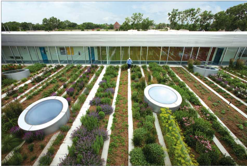
FIGURE 6-32: At the Rooftop Haven for Urban Agriculture at the Gary Comer Youth Center in Chicago, Hoerr Schaudt Landscape Architects used plastic lumber pavers made from recycled milk containers to form pathways within the garden that align with the courtyard garden’s window frames.
