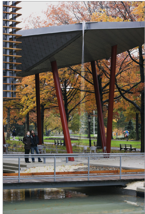
FIGURE 3-61: A roof scupper becomes a visual focal point as it carries rainwater from the roof into the stormwater water feature for holding and eventual reuse.
