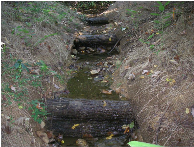
FIGURE 3-44: Step pools focus erosive energy to the bottoms of pools and away from the banks to minimize erosion.
