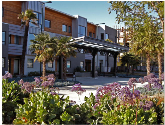
FIGURE 6-7: The repurposed canopy structure in the 14th Street Pocket Park.
