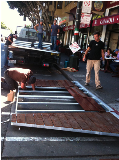
FIGURE 6-19: Each 3-ft-wide prefabricated Walklet module provides a single, specific program (e.g., benches, planters, bike parking, and tables) that can be mixed and matched with other Walklet modules. Modules, constructed of bamboo and redwood, are easily disassembled and removed. They can be recombined and reused in other locations.
