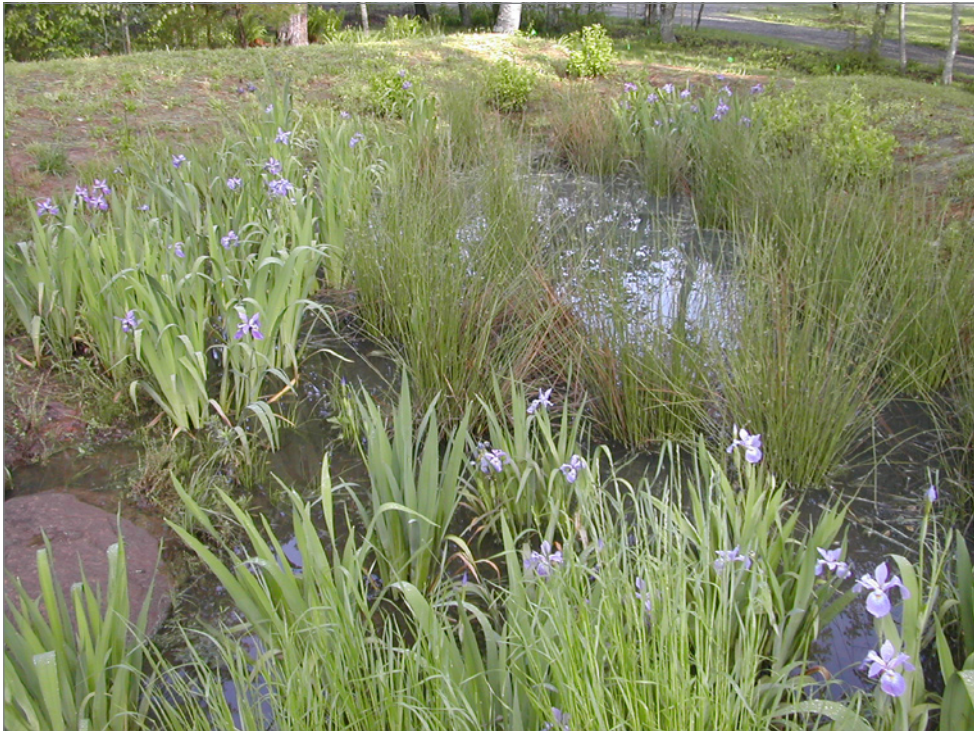
FIGURE 3-54: Stormwater wetland that treats parking lot runoff and is planted with indigenous, emergent aquatic vegetation.
