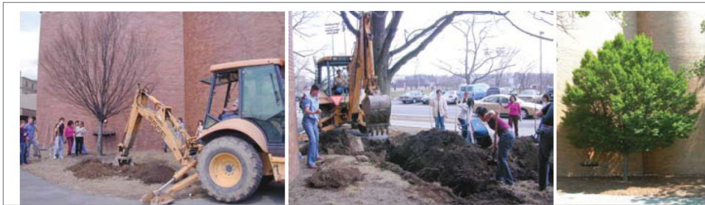
FIGURE 5-27: Radial trenches were excavated to provide a European hornbeam with better drainage. Four years later the tree is thriving.
