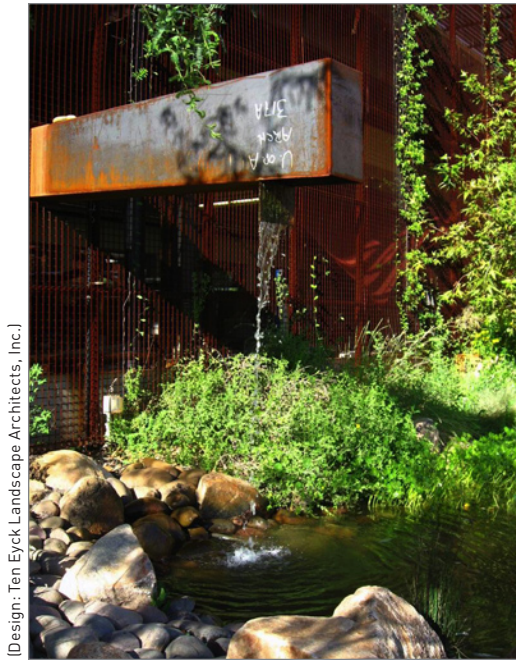
FIGURE 6-33: A reclaimed steel duct is used as a runnel and scupper at the Underwood Family Sonoran Landscape Laboratory in Tucson.
