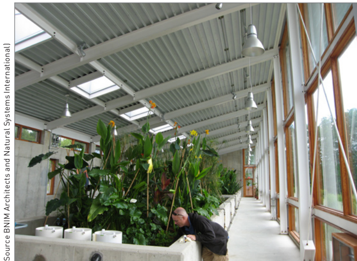
FIGURE 3-82: The Solar Aquatic System at the Omega Center for Sustainable Living in Rhinebeck, New York, designed by John Todd Ecological Engineering and Natural Systems International, is part of an integrated water system for the building and site.
