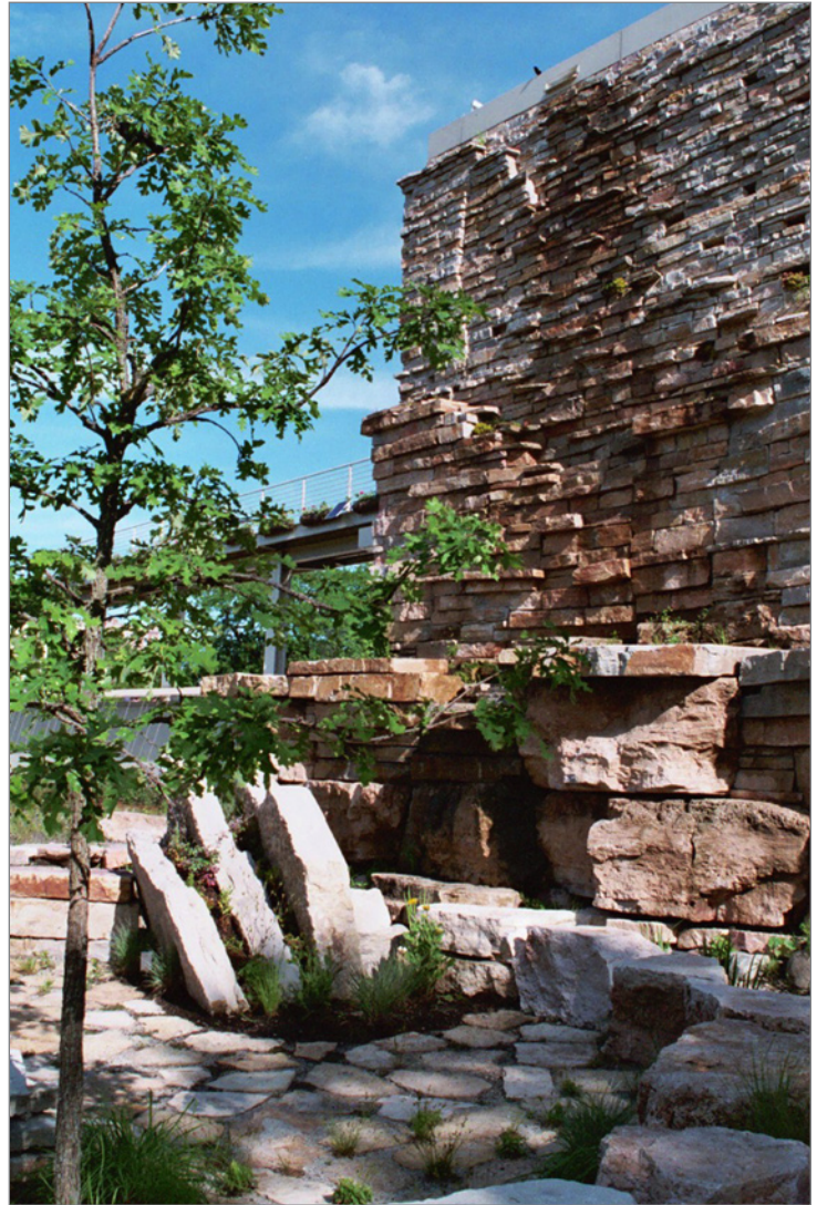
FIGURE 3-71: The facade of the Peggy Notebaert Nature Museum building includes a “water wall” made of natural limestone veneer over a CMU block wall that allows surplus rainwater from the green roof to cascade down to provide water to small planting pockets; overflow water is stored in a cistern and recirculated with solar energy to irrigate the wall and provide makeup water for the created wetland in an outdoor classroom space.
