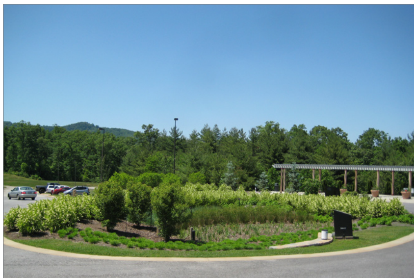
FIGURE 3-38: This bioretention area in the parking lot at the Oregon Museum of Science and Industry receives runoff from adjacent pavement.
