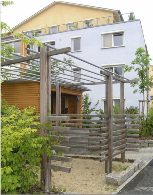
FIGURE 6-8: A parking arbor in Asperg, Germany, uses smaller wood members to provide enclosure. Small lumber sizes and built-up members can be derived from younger trees, shortening the renewability period for wood products.
