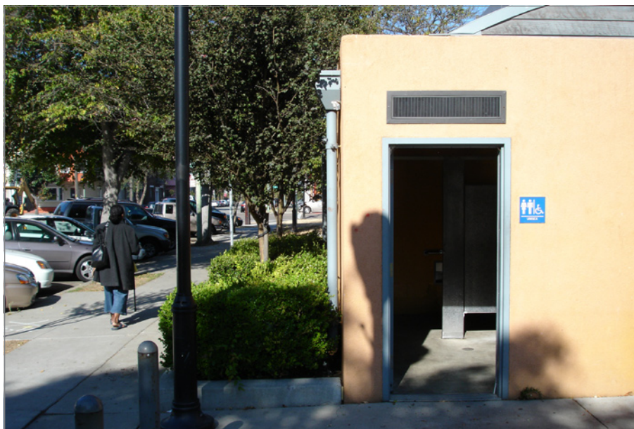
FIGURE 7-9: Restroom facilities at Lafayette Square Park, which are a rarity in many downtown parks, were designed in a creative manner that allows for human needs while responding to concerns about public safety.
