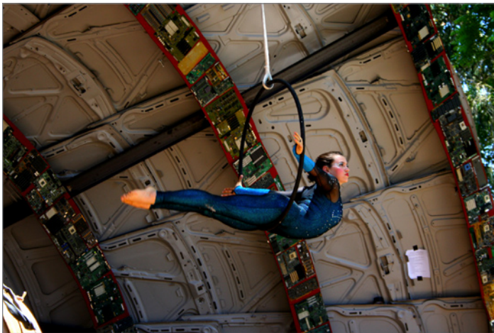
FIGURE 6-23: The project was a collaboration between The Finch Mob, The REBAR Group, and Christopher Guillard of CMG Landscape Architecture. Inside the bandshell, computer circuitboards were a fascia for the reclaimed steel structural members.
