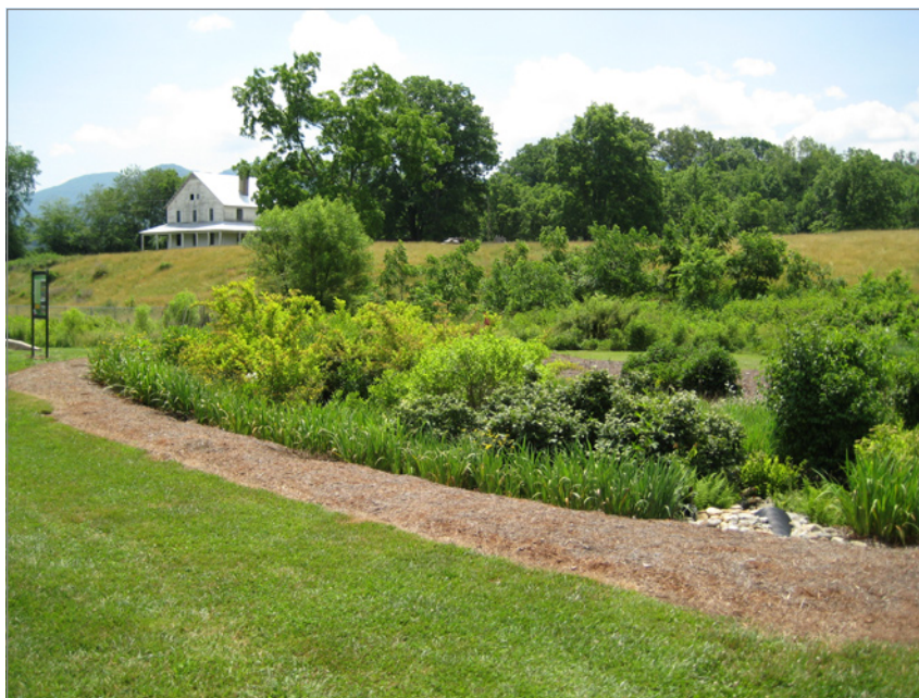
FIGURE 3-39: Bioretention area at an elementary school that features indigenous species to treat roof runoff.
