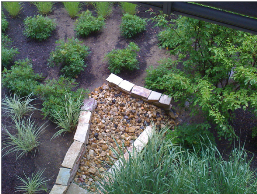
FIGURE 8-14: A bioretention feature, such as this one at the Northwest Community Hospital in Arlington Heights, Illinois, should be monitored after storm events to evaluate for signs of clogging or erosion.
