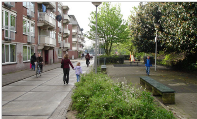
FIGURE 7-34: The Dutch woonerf or living street incorporates trees and park space to slow down vehicular traffic and create a shared street for bikes and people.
