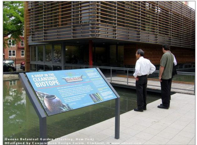
FIGURE 8-17: The water in this water feature at the Queens Botanical Garden is from rainwater that is cleaned via filtration through plant root systems.
