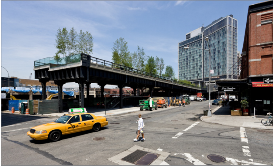
FIGURE 6-11: The existing rail structure of the High Line was retrofitted to make it safe, accessible, and usable, yet the majority of the structure was reused. The design retains elements of the historic railroad.
