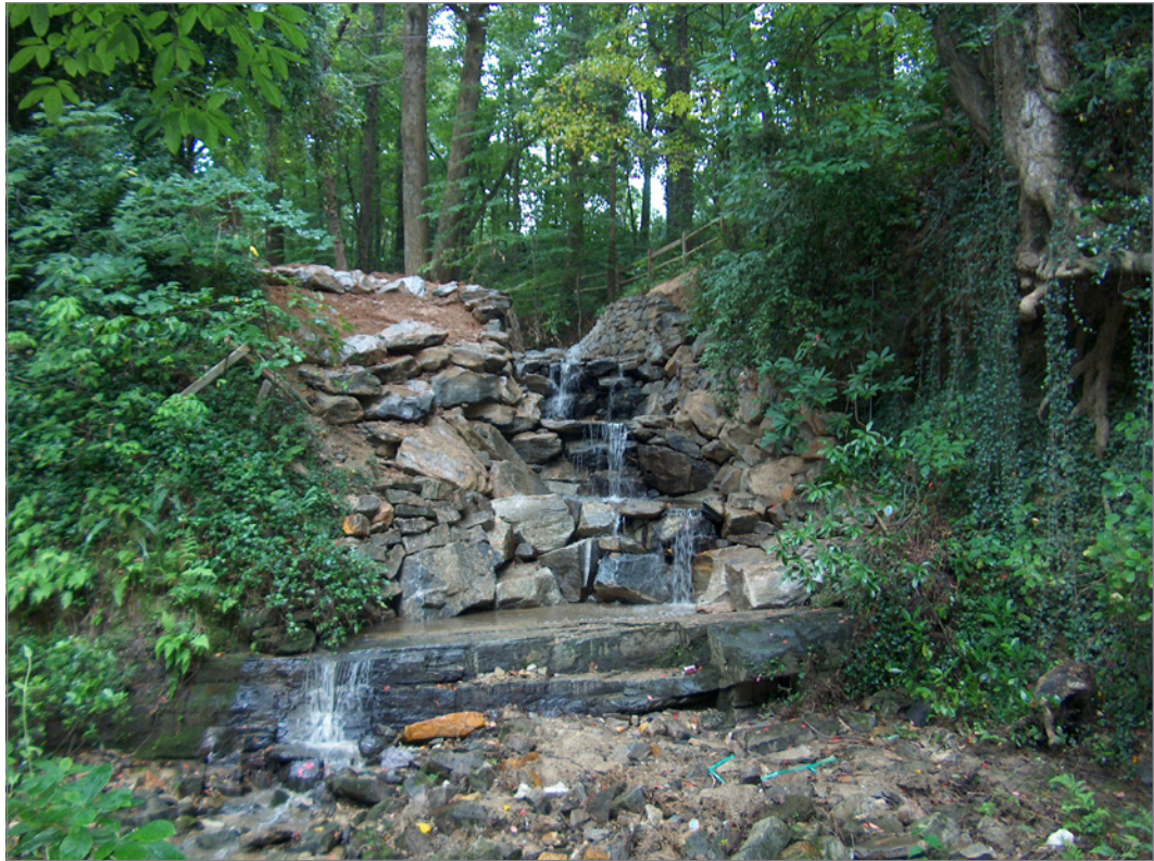
FIGURE 3-43: Significant grade changes require energy dissipation in order to prevent scouring—the natural model of a step pool swale/cascade provides an attractive and functional solution.
