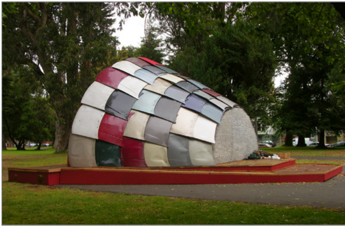
FIGURE 6-22: The Panhandle Bandshell is a modular performance stage structure constructed entirely from reclaimed materials that occupied a place in San Francisco's Panhandle Park for a three-month period in 2007.
