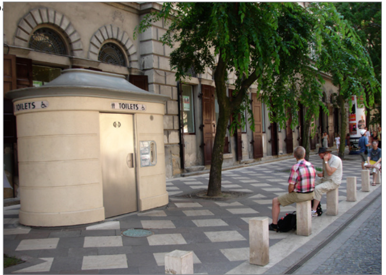
FIGURE 7-13: This free-standing restroom facility in Budapest, Hungary, is designed for human comfort, unlike the adjacent bollards, which serve as makeshift seating areas.
