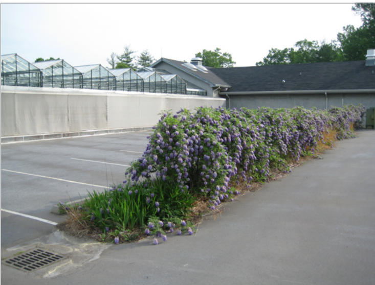
FIGURE 3-48: Bioswale planted with American wisteria, blue flag iris, and soft rush to treat parking lot runoff before draining to stormwater wetland.
