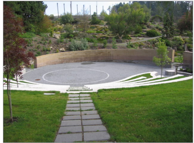
FIGURE 6-30: Rammed earth walls enclose an amphitheater at the University of British Columbia Botanical Garden. Constructed by Clifton Schooley & Associates, the circular wall is 55 ft long and fades into the grade.
