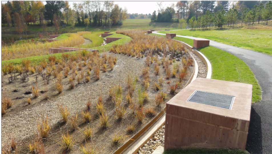
FIGURE 3-51: Runoff is diverted into a series of drop boxes that convey into a level spreader, bioretention area, and littoral shelf at the North Carolina Museum of Art.
