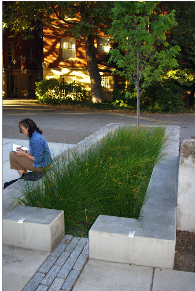
FIGURE 3-13: The bioretention at Epler Hall at Portland State University is an excellent example of a simple design that enhances pollutant removal and increases aesthetic appeal.
