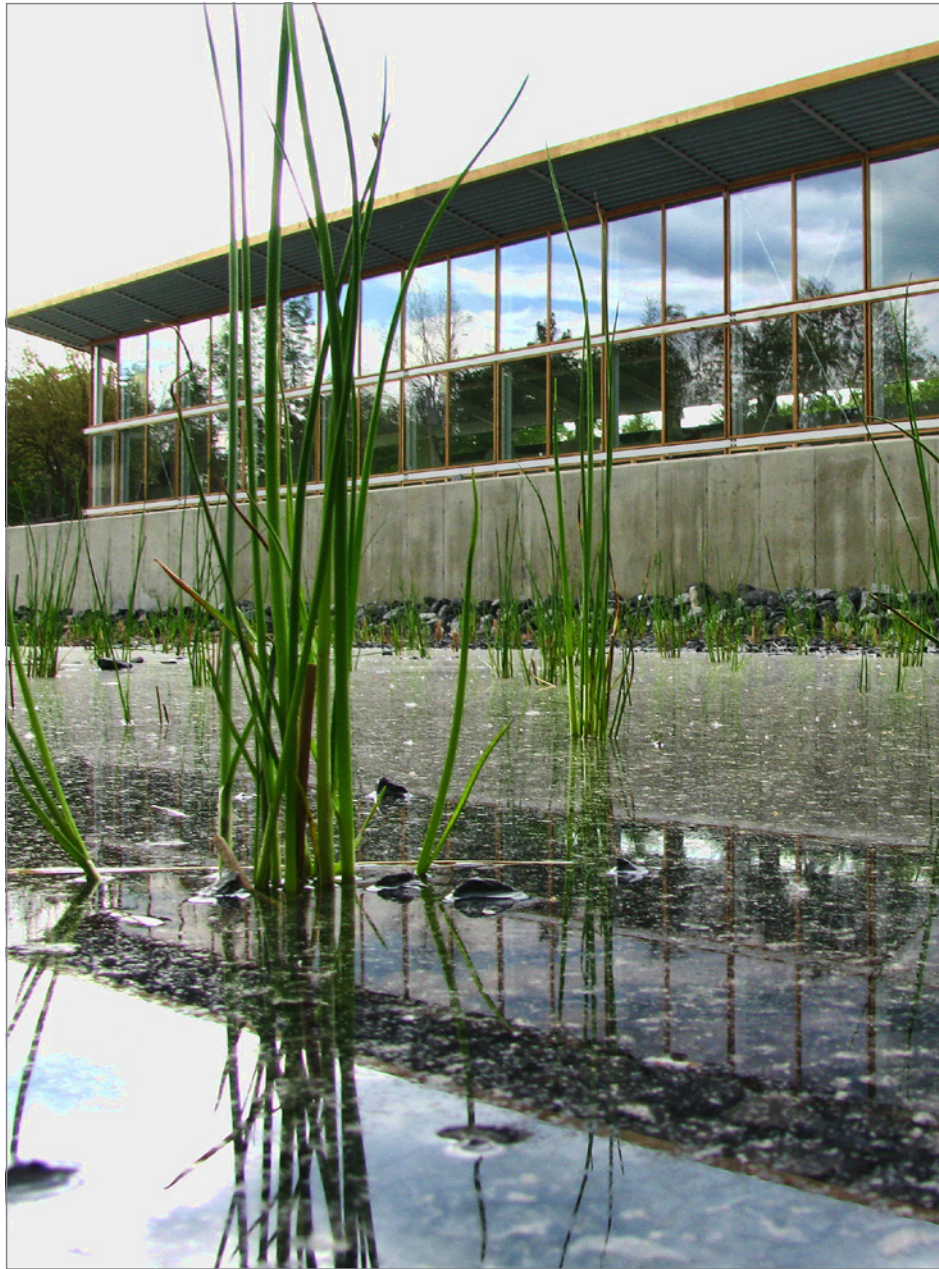
FIGURE 3-67: A living system at the Omega Center for Sustainable Living in Rhinebeck, NY, treats all of the wastewater generated on this 500-acre learning center campus; clean water is then infiltrated through a series of chambers below the parking lot.
