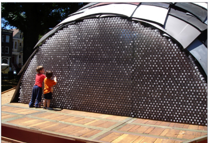
FIGURE 6-24: Sixty-five reclaimed auto hoods clad the structure with a back wall constructed from 3,000 plastic water bottles.
