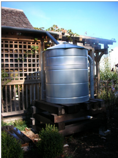
FIGURE 3-27: An aboveground cistern system collects roof runoff for irrigation and water for dyeing fabrics at the North Carolina Arboretum.
