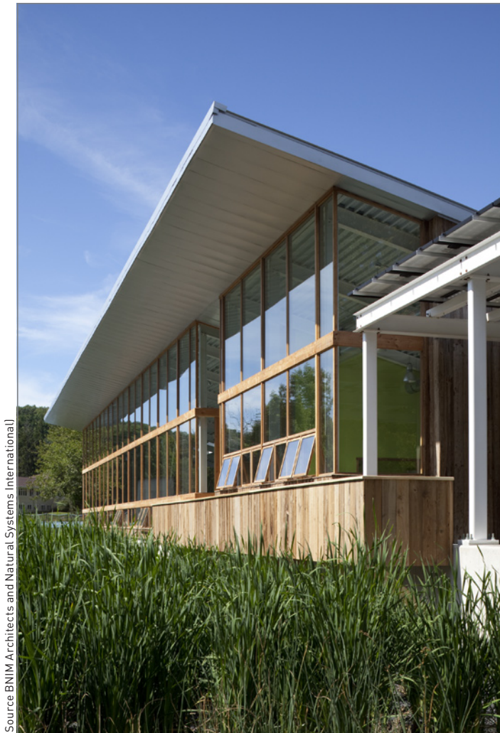
FIGURE 3-83: Constructed wetlands outside the Omega Institute Solar Aquatic System greenhouse treat wastewater and stormwater onsite.
