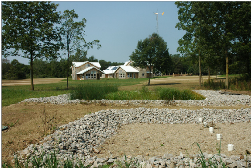
FIGURE 3-80: The Merry Lea Environmental Learning Center was created to house Goshen College's expanding environmental science program and to enable students to live near the ecosystems they study. At Merry Lea, this cycle is achieved in Phase 1 by passing effluent through the constructed wetland and the recirculating sand filter. Including a trickling filter and an aerated lagoon in the treatment process for Phase 2 enhances the nitrogen cycle. The trickling filter and lagoon nitrify the effluent, which is subsequently denitrified as it passes through the wetlands. A similar process occurs within the sand filter, which provides final nitrogen reductions prior to disposal or reuse.
