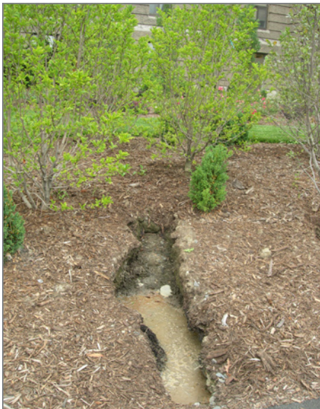
FIGURE 5-30: The effect of a nondraining, compacted subgrade underneath soil that drains well. At the interface of these layers, water does not drain and backs up into the growing medium, severely limiting its usefulness.
