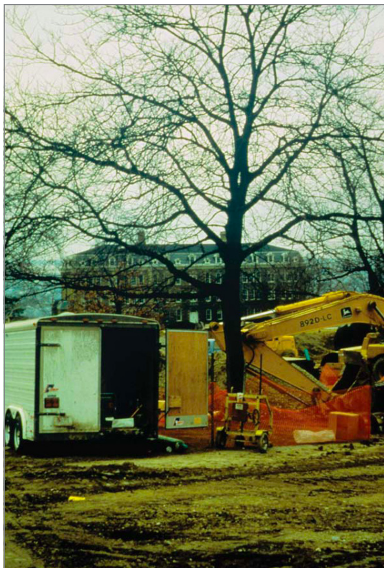
FIGURE 5-35: This construction site offers no protection for the existing tree. Consequently equipment is operated and materials storage is occurring within the root zone of the tree.
