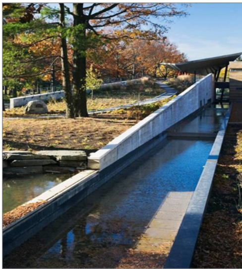
FIGURE 3-60: Harvested rainwater is celebrated in visible, accessible water elements that also clean the water and provide for nonpotable uses.
