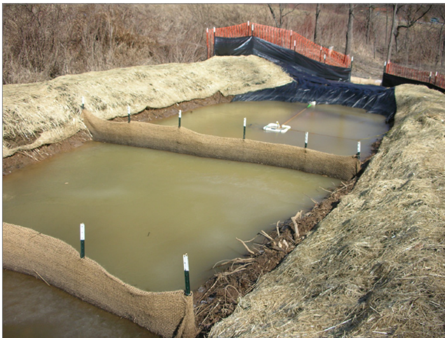
FIGURE 3-57: Skimmer sediment basin with porous baffles. Porous baffles promote laminar flow, and topwater drawdown devices help minimize turbidity and sediment discharge into receiving waters.
