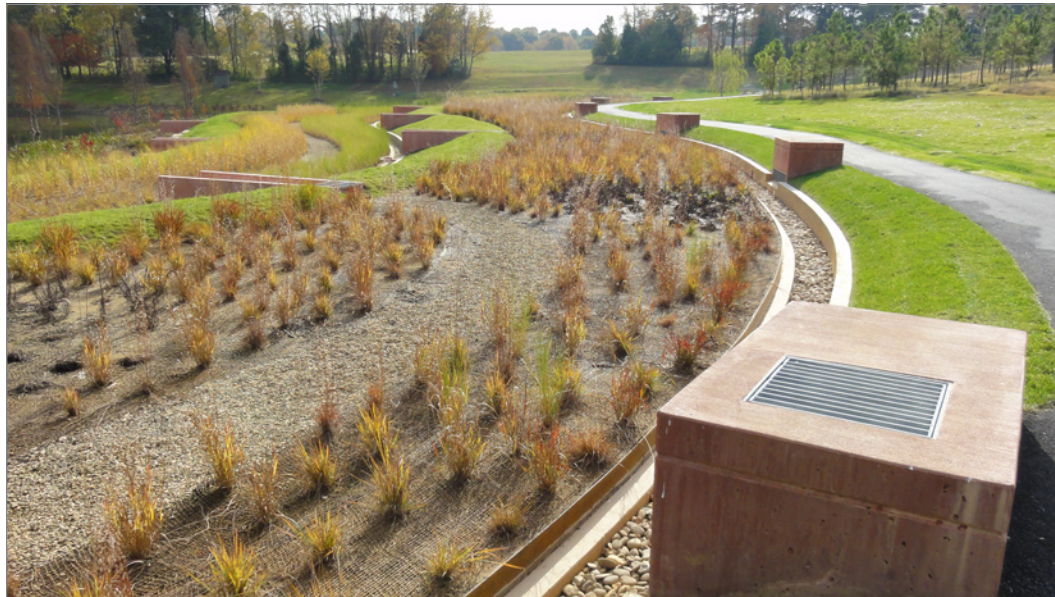
FIGURE 3-35: The "pocket rain garden," a name coined by Glenn Palmer, is generally smaller than a bioretention area and consists of amended, indigenous soils and plants.
