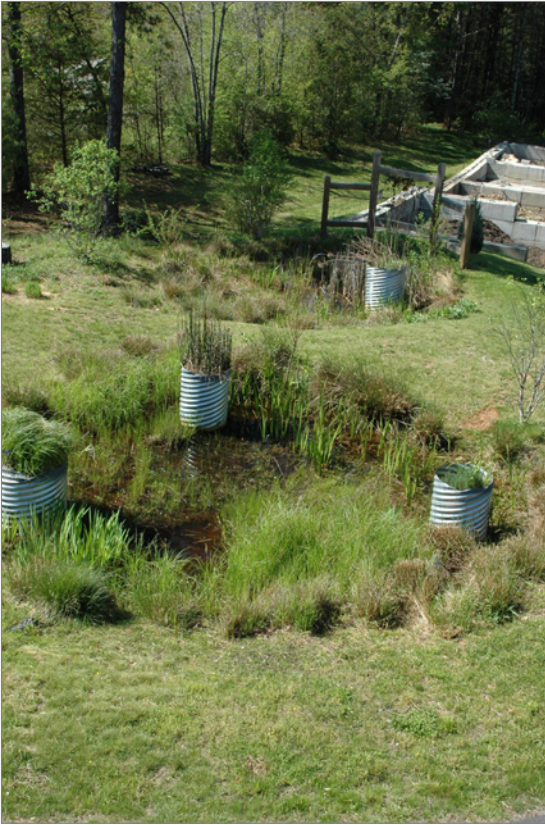
FIGURE 3-47: Bioswale with micropools. Roof and parking lot runoff is treated by flowing through swales and pools.
