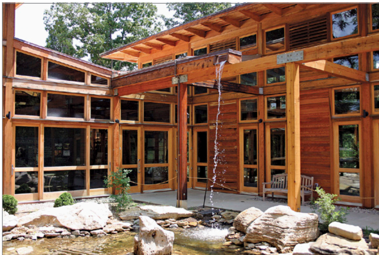
FIGURE 6-17: The mechanical connections and reconfigurable modules at the Bernheim Arboretum Visitor Center in Clermont, Kentucky, allow for ease of disassembly and deconstruction for building alterations.
