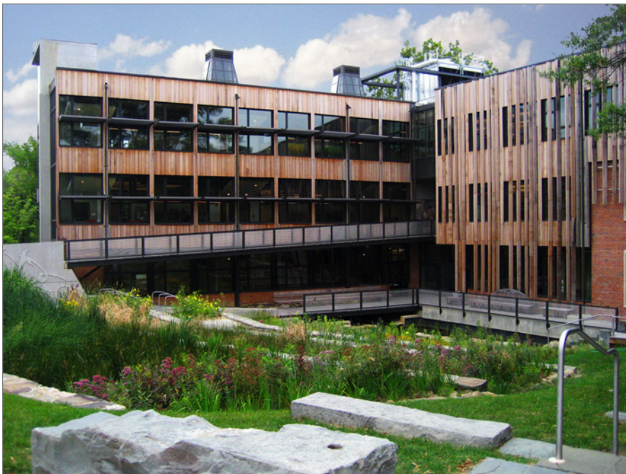
FIGURE 3-76: The Sidwell Friends Middle School incorporates a constructed wetland, the first in Washington, DC, that treats building wastewater onsite. Other wetlands and rain gardens treat onsite stormwater.
