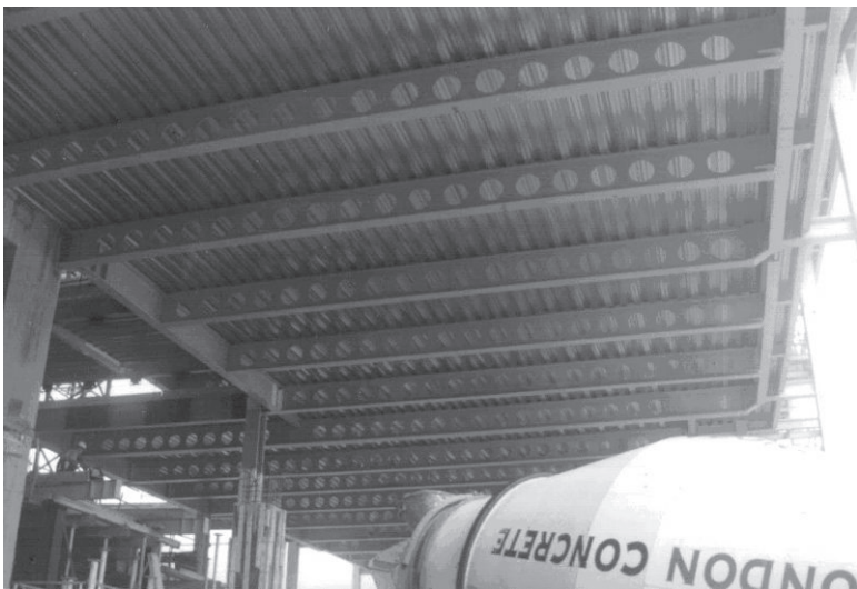
8.5 Composite steel–concrete beams, More London, UK.
