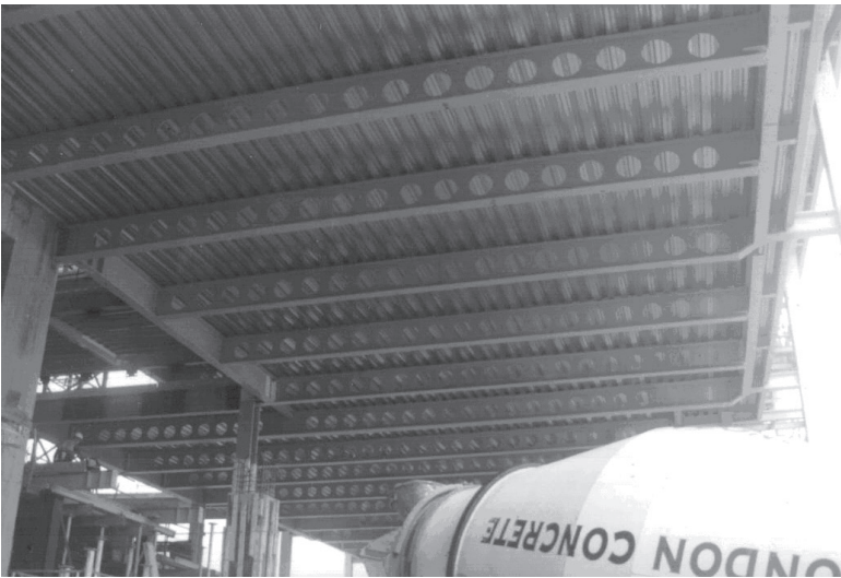
8.5 Composite steel–concrete beams, More London, UK.
