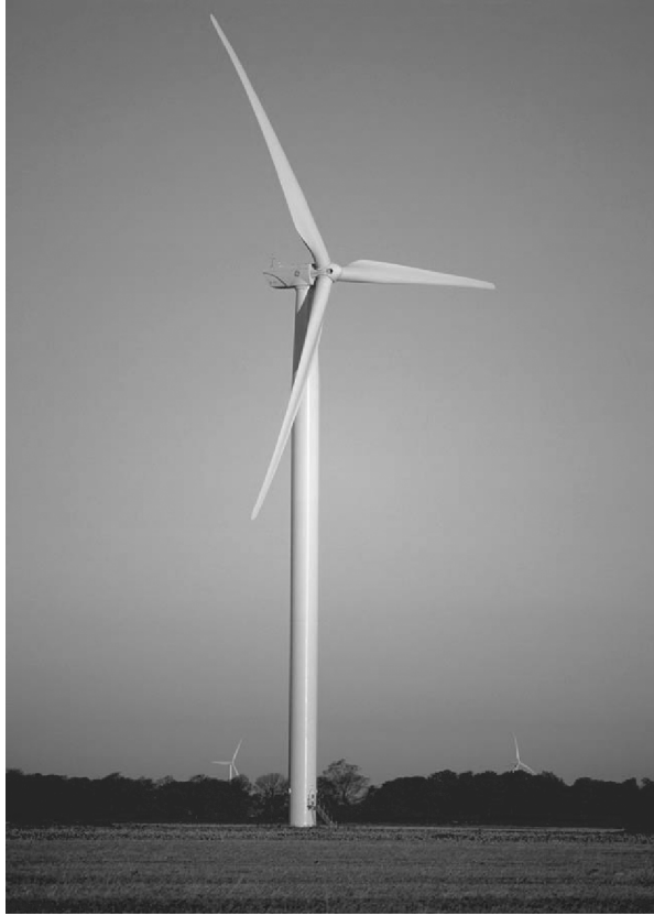
Figure 2 GE 2 · X prototype in Wieringermeer, Netherlands. (Courtesy of Ref. 5.)
