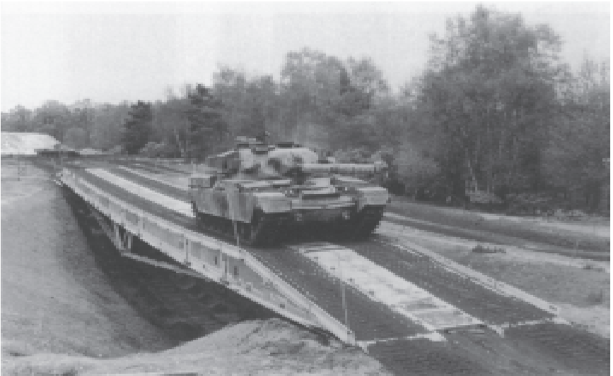
The 'BR90' bridging system, which entered service with the British Army in 1997. The trussed version shown here is carrying the Challenger battle tank on a 56m span. Built by Vickers Defence Systems at Wolverhampton, using 7xxx-series alloy.
