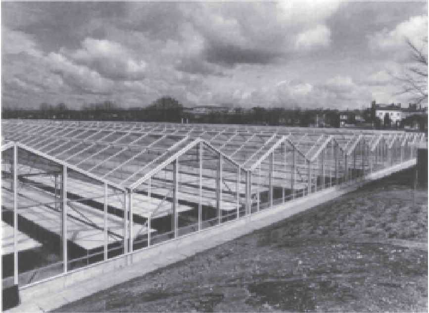
Aluminium glazing system for commercial greenhouses, built from a suite of extrusions including a special valley gutter section. (Courtesy of Cambridge Glass Co.)
