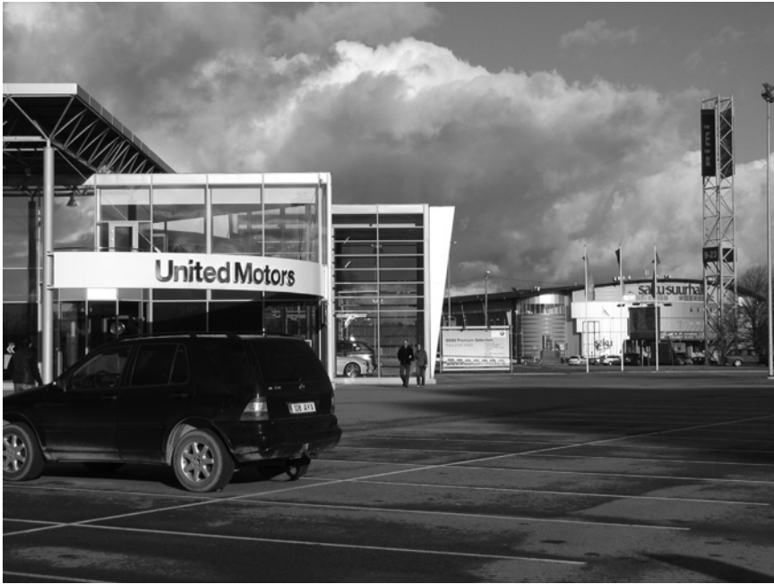
Figure 7.7 New retail and service facilities on the edges of the city (Tallinn, Tabasalu roundabout). Photo by Kadri Leetmaa.
