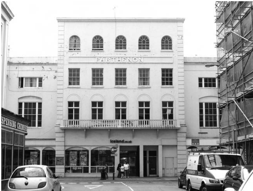
4.11. The Parthenon, Leamington Spa, 1819 combined reading rooms and a ballroom.
