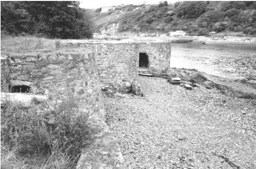
2.5. Lime kilns on the quay, Solva, Pembrokeshire. Small kilns like these are commonly found in harbours and estuaries where the lime and fuel were probably delivered by sea and the burnt lime taken inland by horse and cart (by kind permission of Marilyn Palmer).
