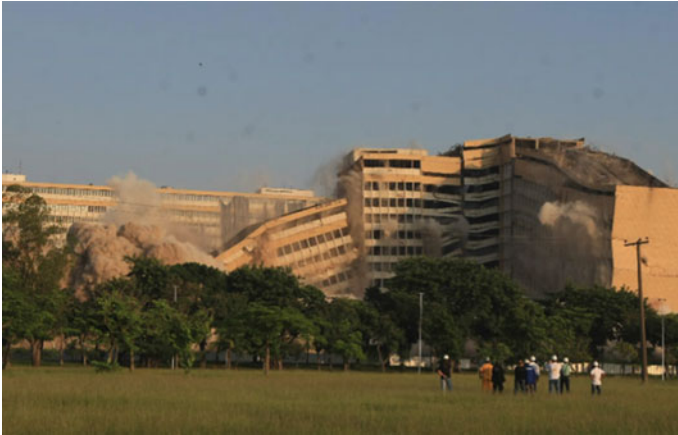
Fig. 4.17 Demolition of hospital section, Ilha do Fundão, Rio de Janeiro, Brazil
