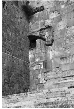
The remains of the Double Gates can be seen immediately above the protruding arch in the form of a half lintel and subtle arch. The wall made of small stones located to the left of the arch was constructed by the Crusaders in about AD 1099.
