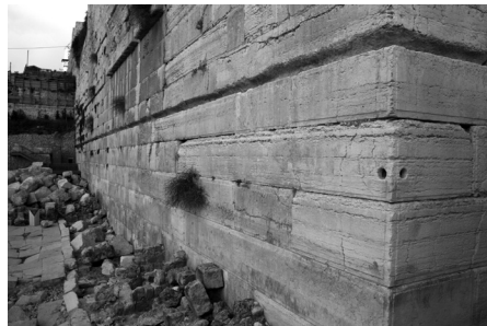
The southwest corner of the Temple Mount features some of the largest Herodian stones visible above ground. As the builders placed these massive stones one upon another, they carefully made sure that each stone was set back about one inch from the lower stone it rested upon. This ensured that the enormous weight and pressure from the fill material placed on the other side of the wall would not cause the wall to collapse.
