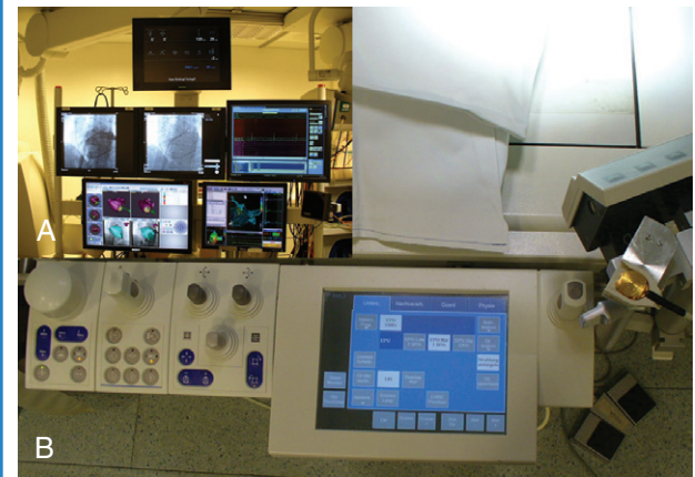
FIGURE 21-3 A , Monitor gantry with six monitors arranged to allow the best orientation for the operator, with live monitors for fluoroscopy and intracardiac signals side by side. B , Controls of the fluoroscopy system (AXIOMS Artis; Siemens, Munich, Germany) positioned at the table side to allow rapid navigation through recorded scenes, again supporting single-operator functionality.
