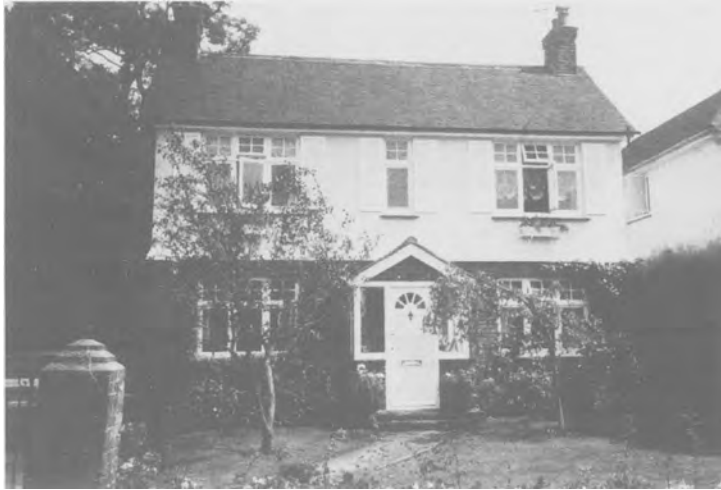
FIG. 9.3. Typical rendered outside wall on upper part of a house.
