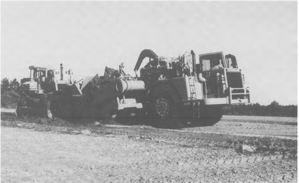
FIG. 4.5. Overburden being removed by scraper with tractor-dozing assistance (courtesy of Caterpillar).
