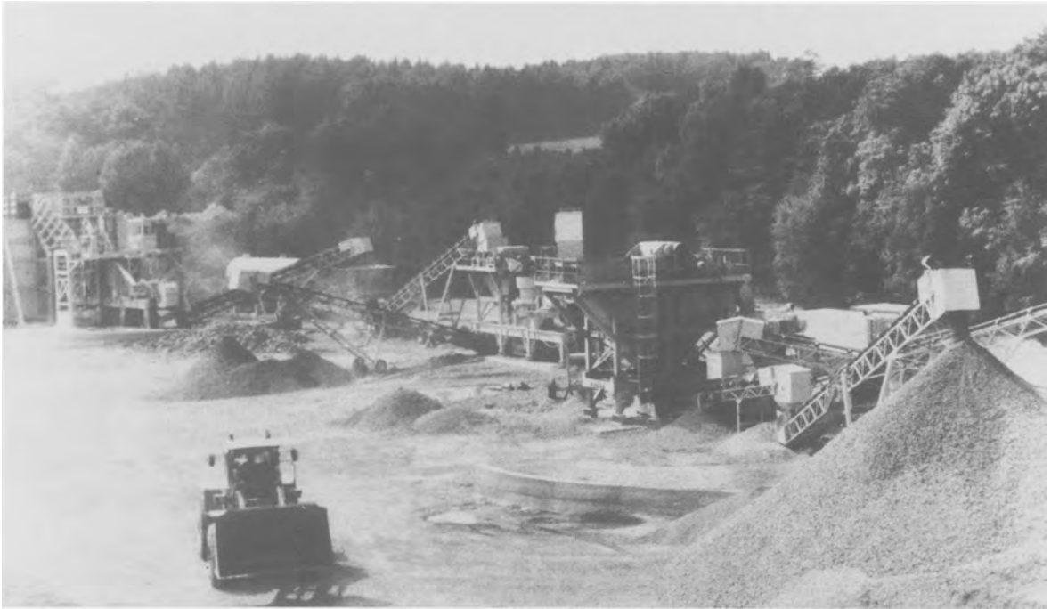
FIG. 5.55. Modular mobile plant crushing 'granite' (courtesy Pegson Ltd).
