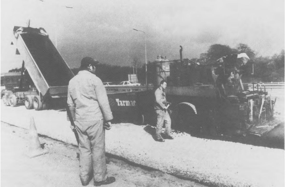
FIG. 10.2. Bitumen macadam being laid over an unbound sub-base.
