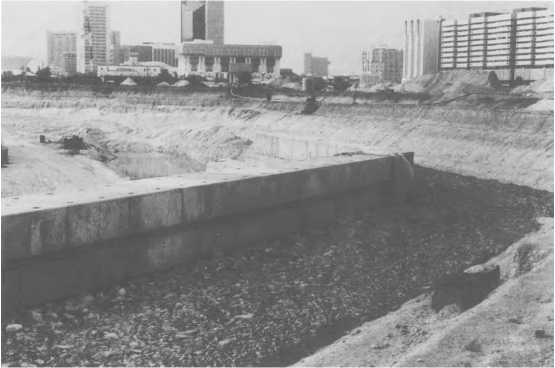
FIG. 13.3. Filter media placed behind sea-wall.
