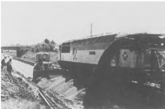
FIG. 12.2. Blanketing sand being laid (courtesy K. Rowlands, British Rail Civil Engineering).
