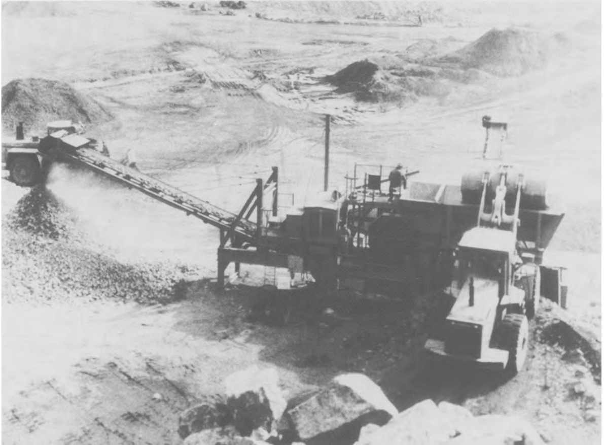
FIG. 5.54. Mobile crusher producing DTP type-1 aggregate (courtesy Pegson Ltd).
