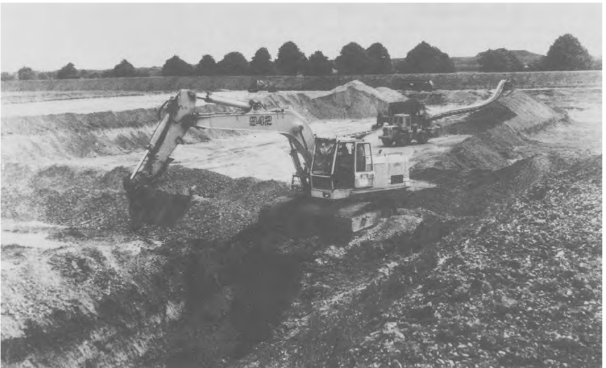
FIG. 4.18. Hydraulic back-hoe excavator loading a field conveyor system (courtesy of Tarmac).
