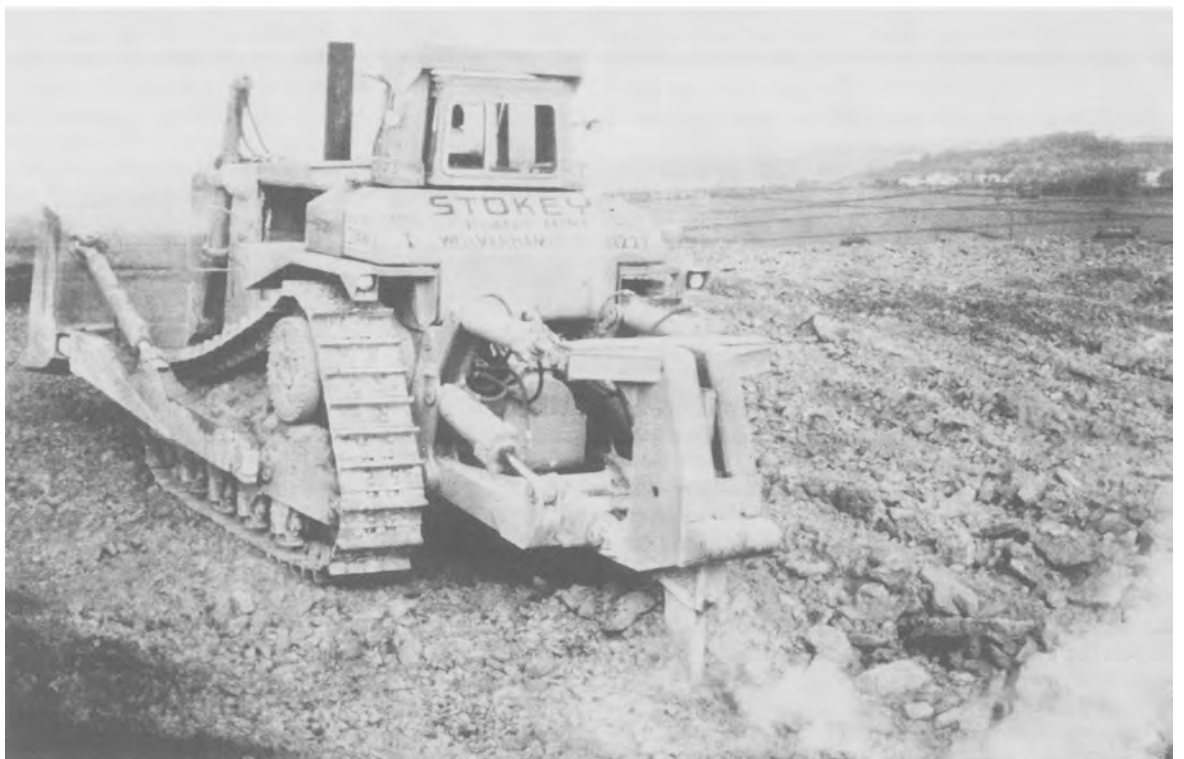
FIG. 4.6. Tractor-dozing machine fitted with ripper (courtesy of Caterpillar).
