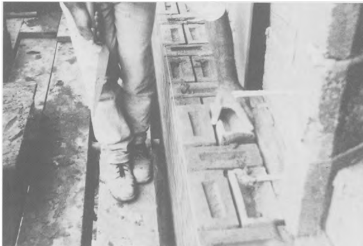
FIG. 9.1. Typical brick and mortar construction for jointing.
