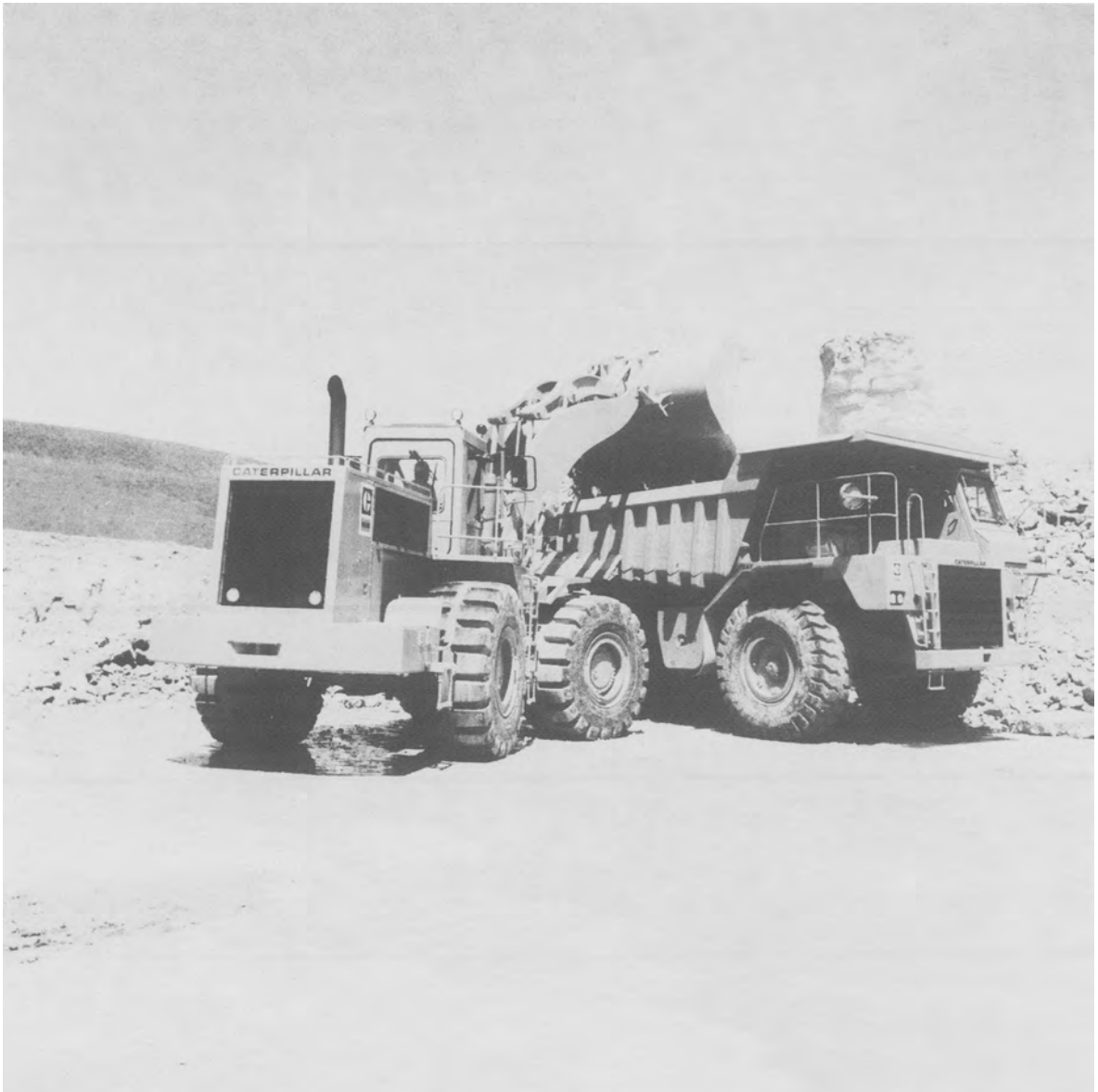
FIG. 4.19. Wheeled loader (F.E.L.) loading a rigid body dump truck (courtesy of ARC Ltd).
