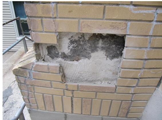
Fig. 18. Outer layers of cracked stucco overlay removed exposing underlying masonry.
