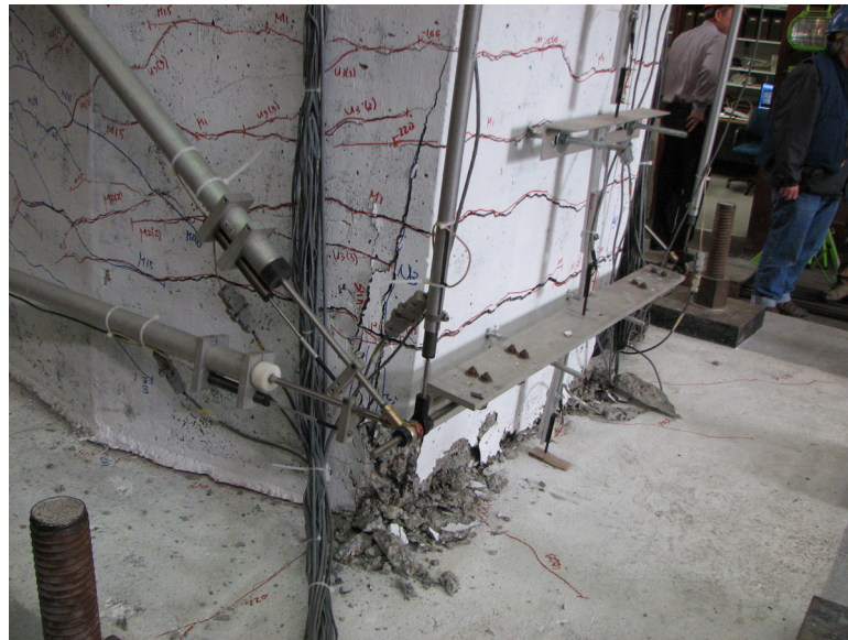
Fig. 4: South Column at 12-Inch Positive Displacement
