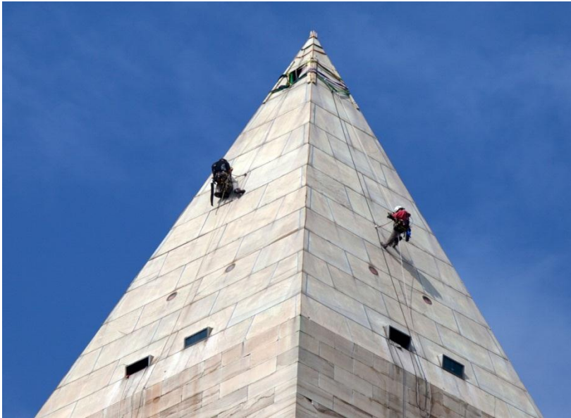
Figure 7. Rope access on the Washington Monument
