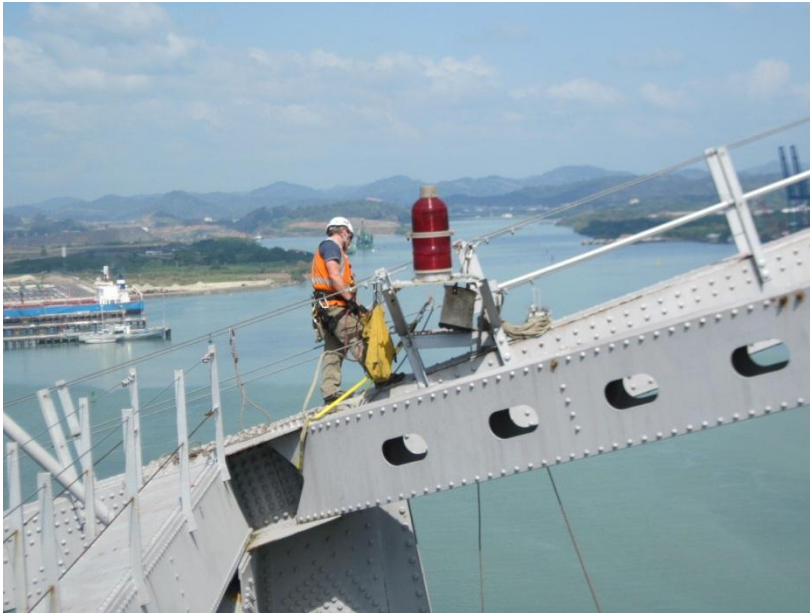
Figure 9. Rope access on a pier at the Bridge of the Americas
