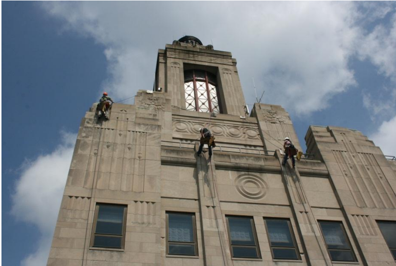
Figure 11. Rope access on the Bank of America building
