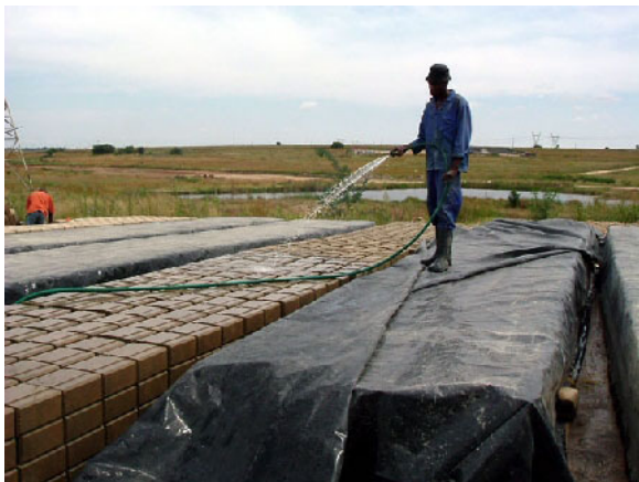
Figure 2: Curing process of interlocking blocks Source: Field Survey, 2011
