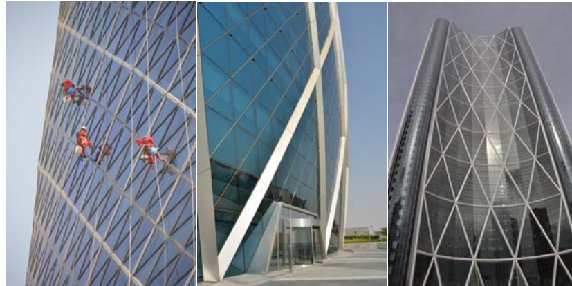
Fig. 4: Capital Gate, Abu Dhabi (left) has a small module and uses a triangular window system that accommodates operable windows. Aldar HQ, Abu Dhabi (center) has a larger module and also employs a triangular system. Bow Encana, Calgary (right) has the largest module and the faceting of the structure allows for the use of a rectilinear glazing system.
