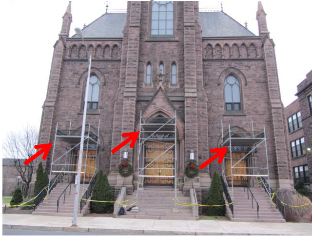
Fig. 3. Overhead protection allowed for continued use of the front entrance.
