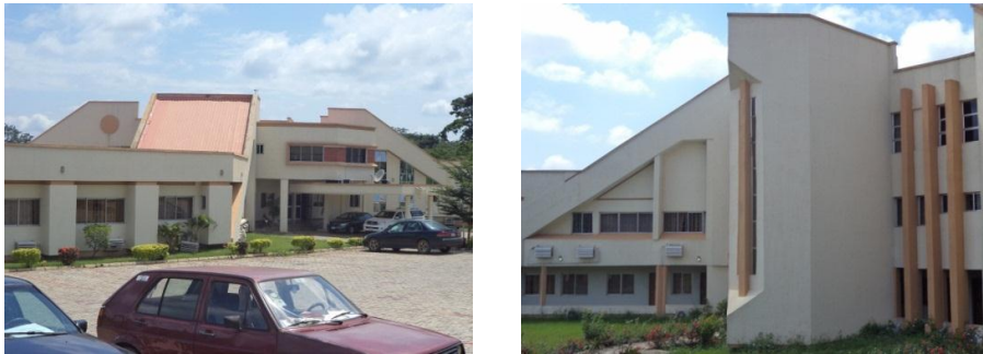
Figure 6: Views showing the slanting roof planes
