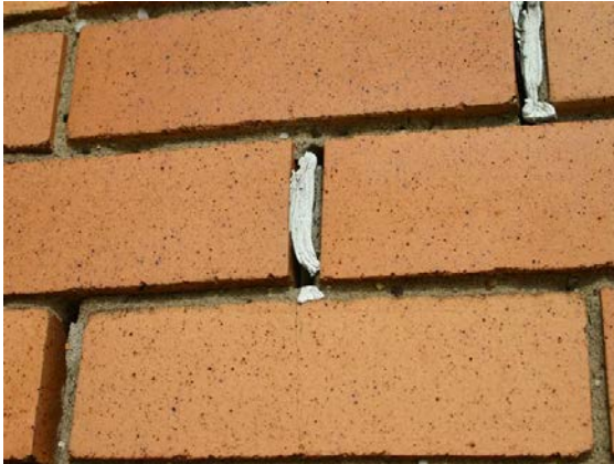
Fig. 16. Sealant applied over failed mortar joints.
