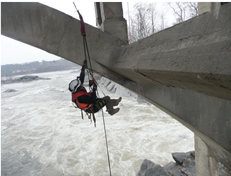
Figure 6. Example of rope access
