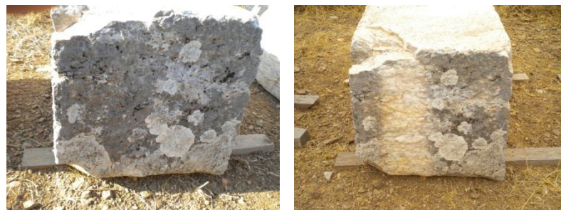
Figure 6. Before and After Cleaning-Wall Block . Left- AT099 before any treatment in 2011, Right- AT099 in 2012, one year after the treatments. It is clear that the algae and lichen was killed with the solution applied, and new growth was successfully avoided.
