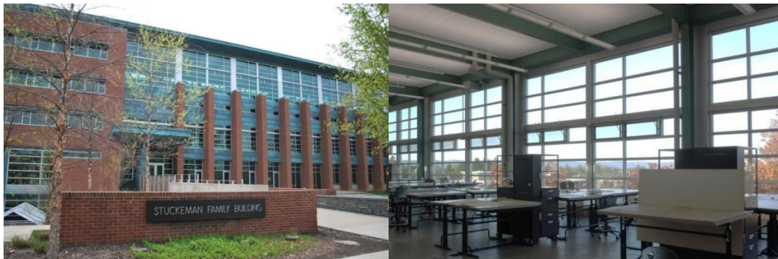
Figure 1: The School of Architecture and Landscape Architecture's (SALA) Stuckeman Family Building located on Penn State's University Park campus can be seen with its curtain wall from the interior and exterior perspectives.
