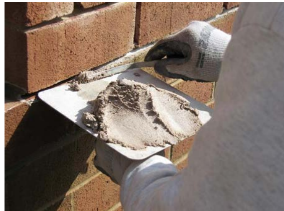
Fig. 20. Placement of new mortar in multiple lifts.
