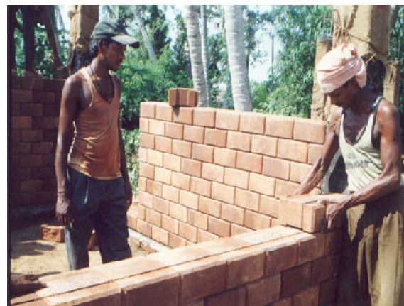
Figure 3: Construction process of interlocking masonry.
