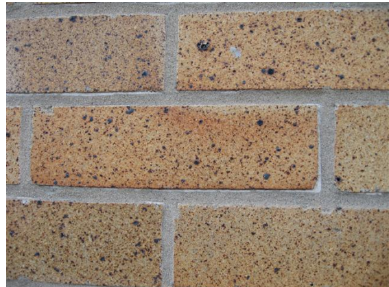
Fig. 14. Thin layer of grout applied to the masonry surface.
