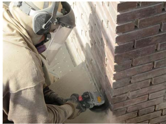
Fig 19. Part of the mortar joint removal process.
