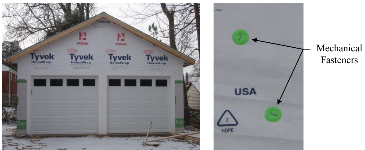
Figure 1: Mechanically Fastened Barrier applied to a Building Exterior
