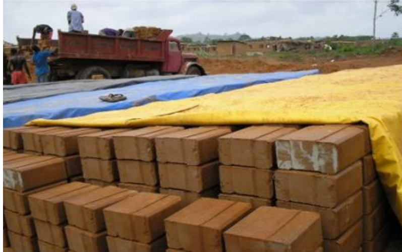
Figure 1: Curing and Stacking of Interlocking Blocks
