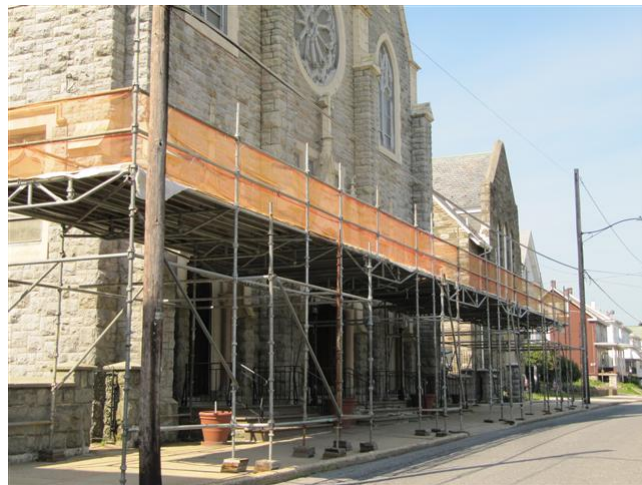
Fig. 4. Overhead protection installed along entire length of sidewalk.
