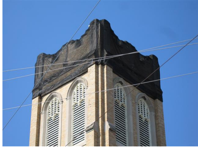
Fig. 8. Properly installed netting at the top of a church tower.
