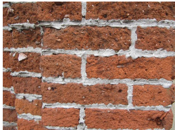
Fig. 15. Sandblasting removed the fired brick exterior surface.
