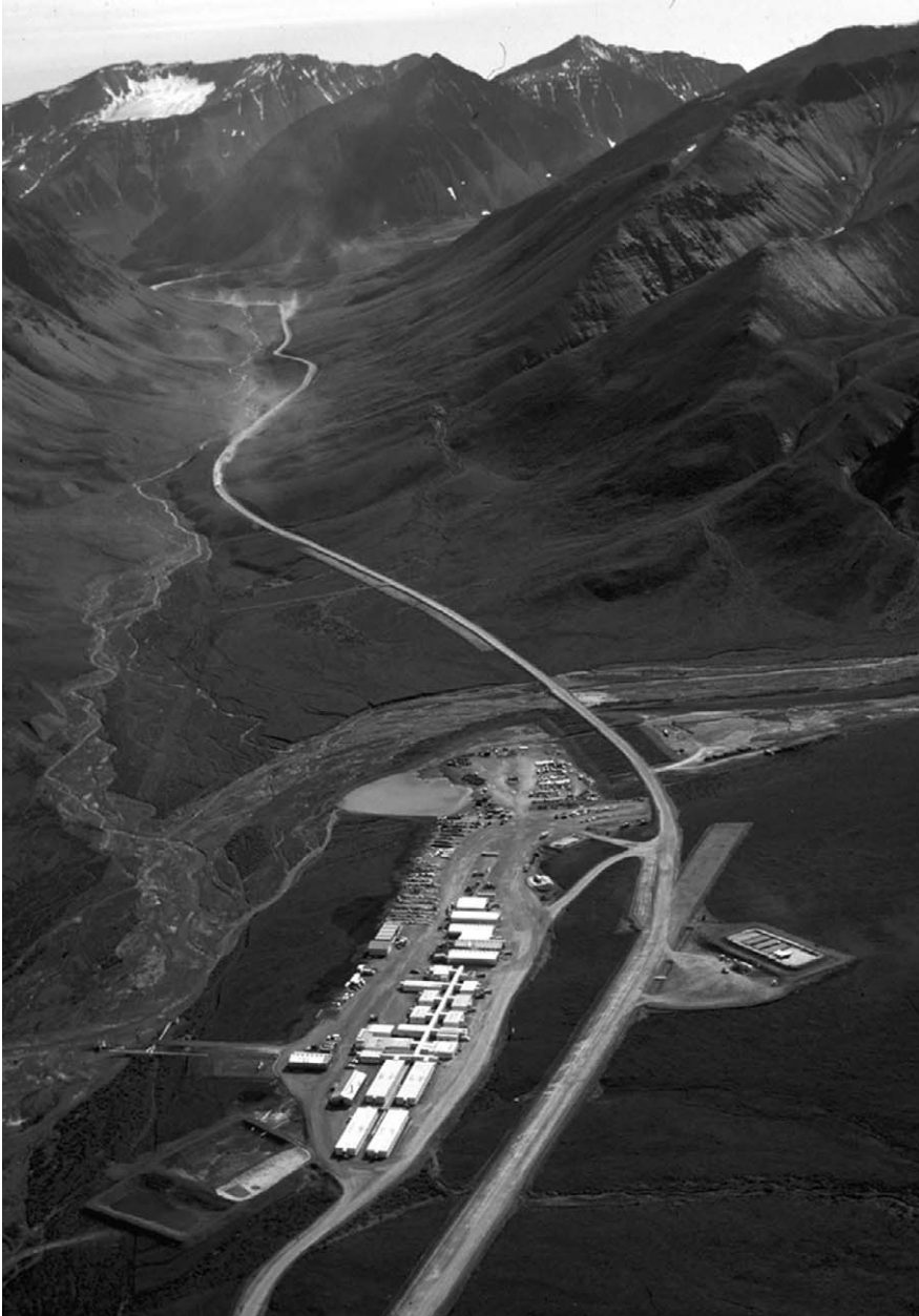
Figure 5.34 Atigun construction camp, Trans-Alaska Pipeline project. © Alyeska Pipeline Service Company.
