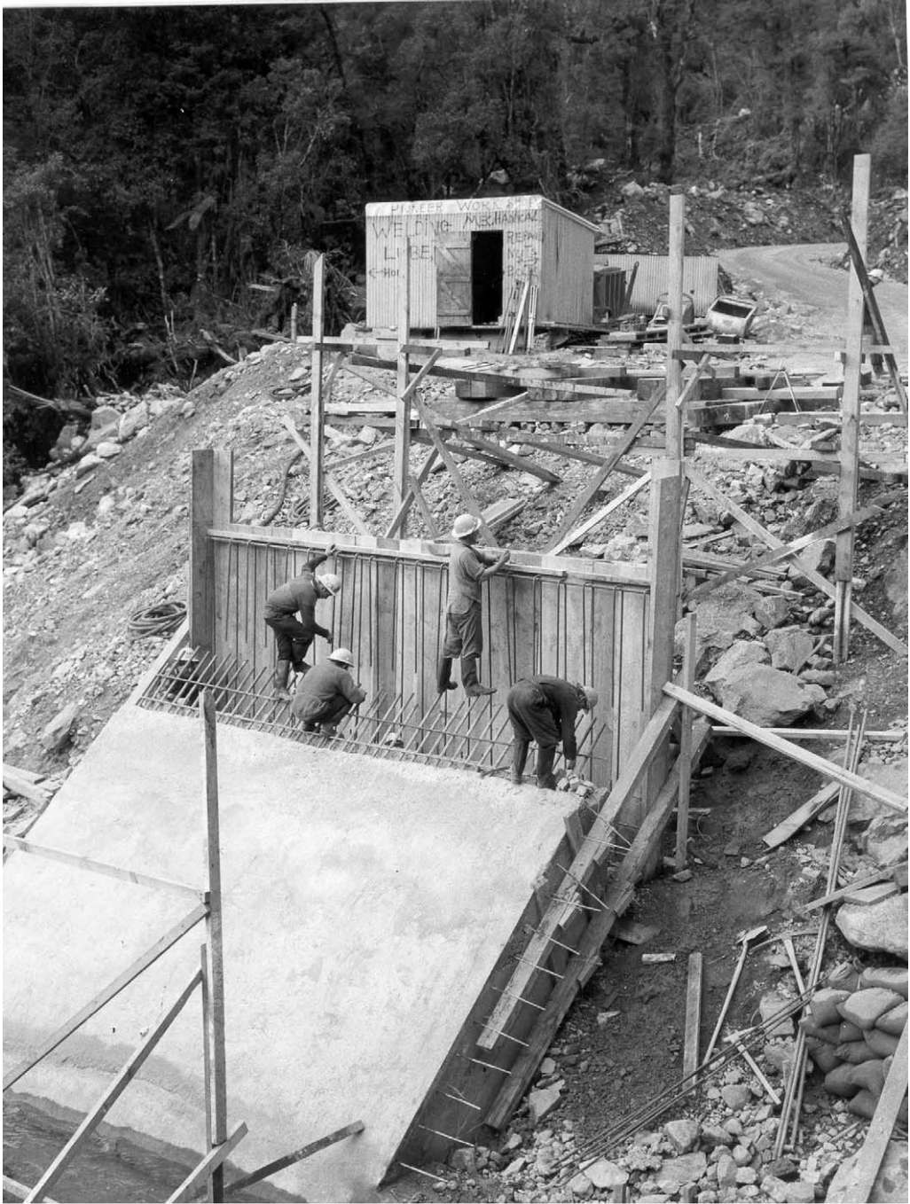
Figure 5.29 Bridge construction on Wilmot pass road, 1965.
