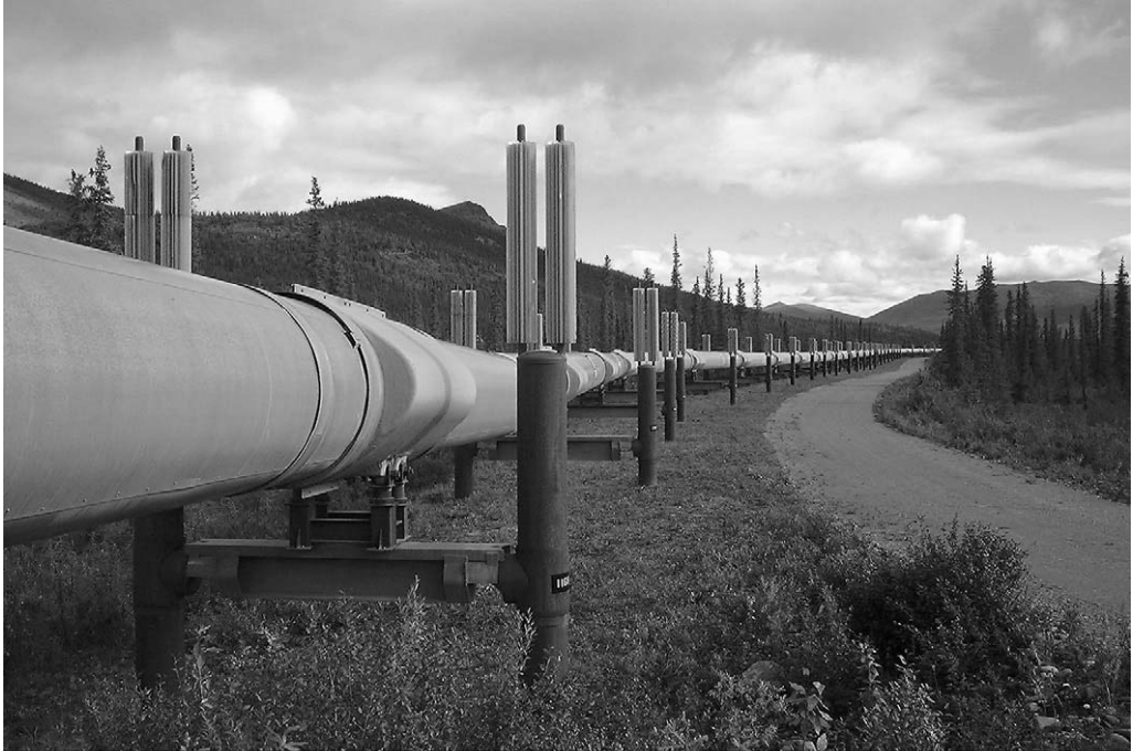
Figure 5.32 Large portions of the Trans-Alaska Oil Pipeline were built in remote areas of the USA's largest state.
