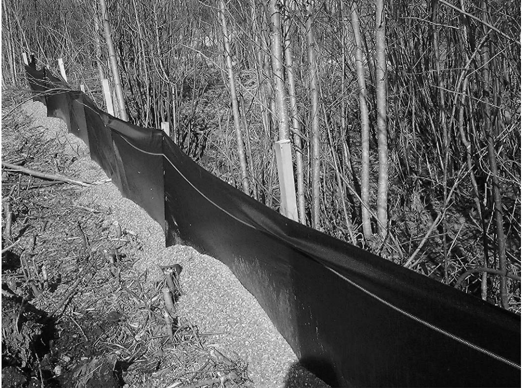
Figure 6.10 Silt Fence, 350–400 mm high, beside highway project clearing, Wasilla, Alaska.
