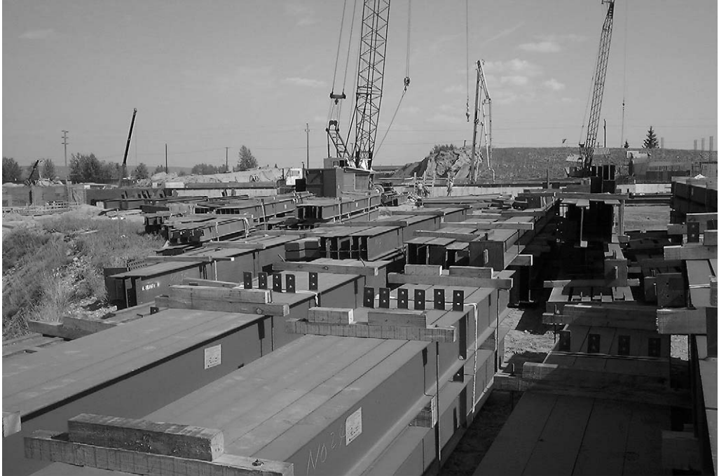
Figure 6.17 Portion of structural steel laydown yard, Bassett Hospital Replacement Project.
