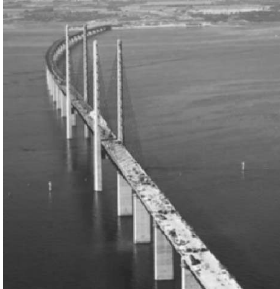
Figure 2.12 Öresund bridge under construction, November 1999. Looking east toward Malmö, Sweden. Courtesy of Hochtief AG, Essen, Germany.
