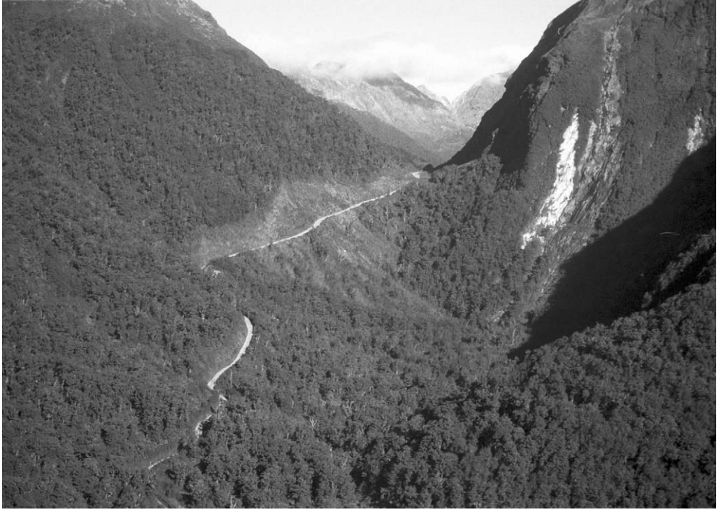
Figure 5.30 Deep Cove side of access road over 700m Wilmot Pass.
