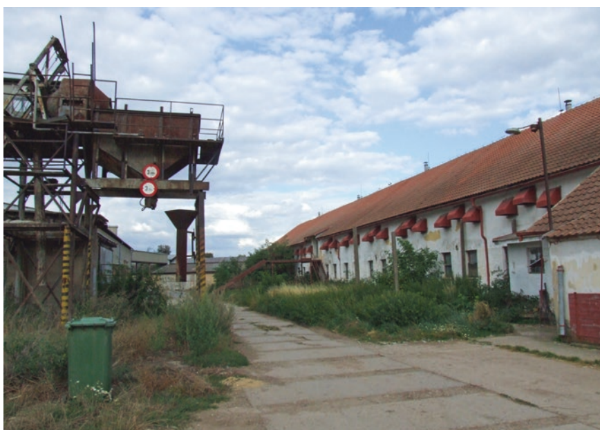
Fig. 3.18 Agrobrownfields. Following the disintegration of large cooperatives, many former farm buildings and agricultural complexes fell into disuse and neglect (often due to unclear ownership rights). Such buildings keep decaying and gradually become overgrown by shrubs and trees. Photo Radim Perlin
