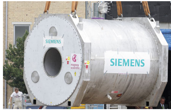
Fig. 21 The 9.4 T 90 cm MRI magnet from Magnex/Varian (D. Houlden 2010, private communication) being craned into a building
