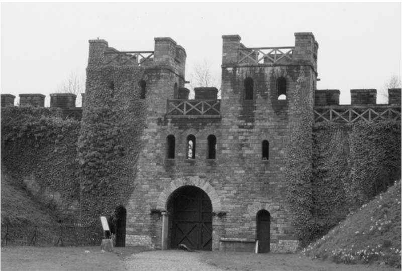
Figure 6.7 The rear gate
