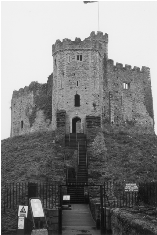
Figure 6.3 The original tower on the motte
