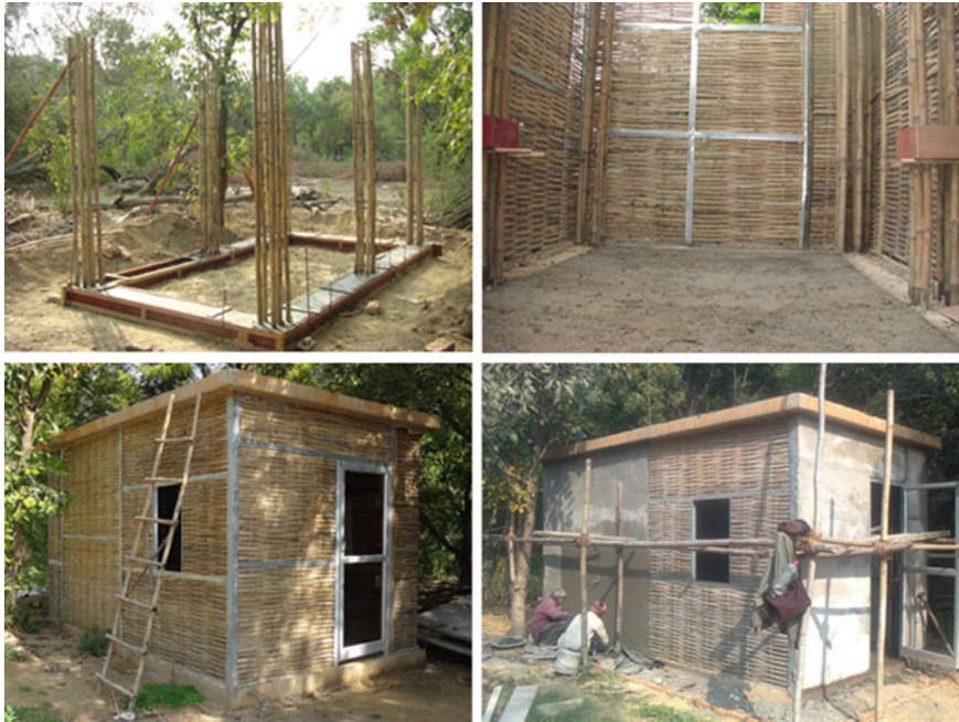
Fig. 2 Different stages of bamboo concrete house construction at IITD
