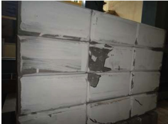
Fig. 5 Crack pattern due to out-of-plane load
