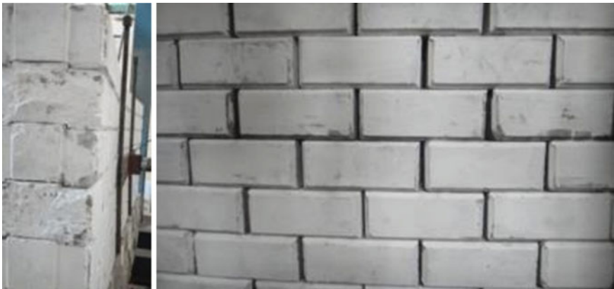
Fig. 16 Failure patterns of flexure loading under horizontal loading
