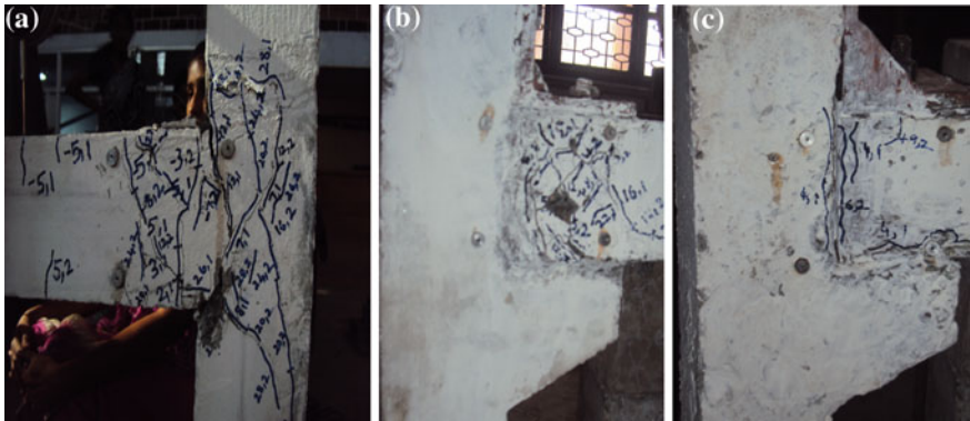
Fig. 6 Crack pattern of all specimens. a Specimen MO. b Specimen SD-SS. c Specimen SD-DS
